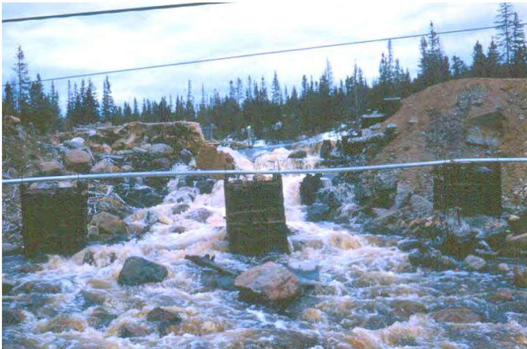
Photo 24: View looking at former pipeline carrying diesel fuel from the shipping dock fuel tanks in the Town of Cartwright to the main fuel storage tank at the Site - June 1964.
