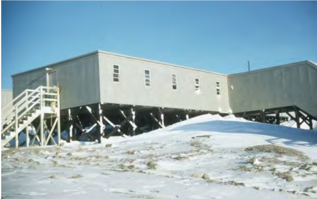
Photo 3: View of typical barracks at Cartwright Air Station. Note the wood cribbing with preservative supporting the barracks - 1953
