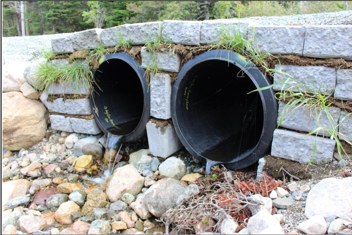
Figure 5.8 Two Culverts with a Shared Outlet Location
