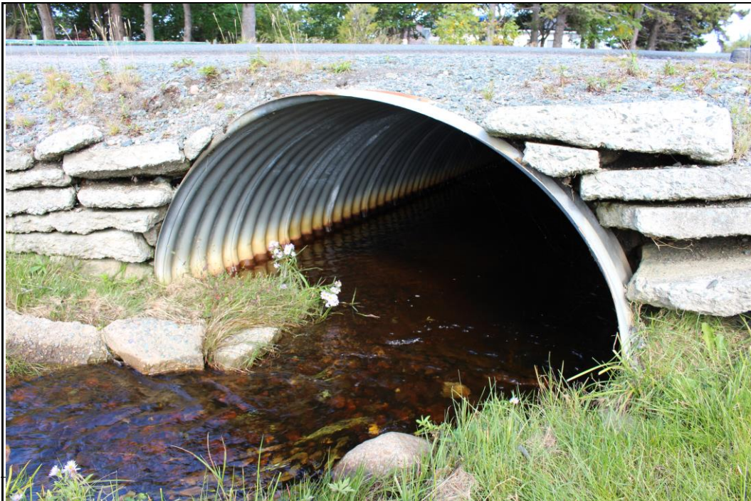
Figure 5.3 Corrugated Steel Arch Culvert
