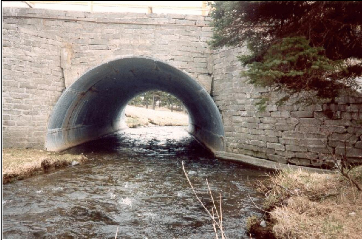
Figure 5.9 Pipe Arch Culvert with Masonry Headwall and Wingwalls
