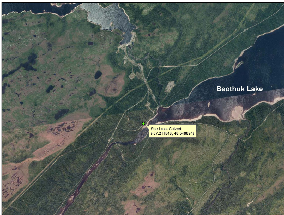
Replacement of a culvert across an unnamed tributary of Beothuk Lake
