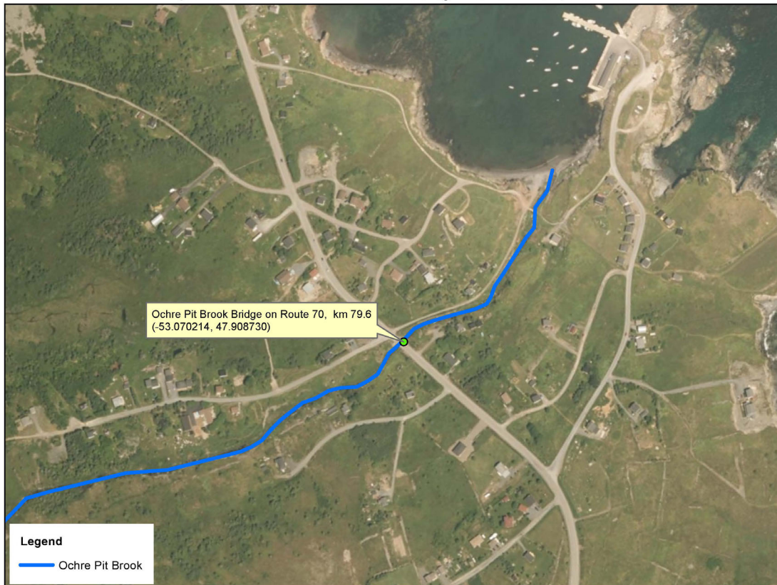
Replacement of Ochre Pit Brook Bridge on Route 70, km 79.6
