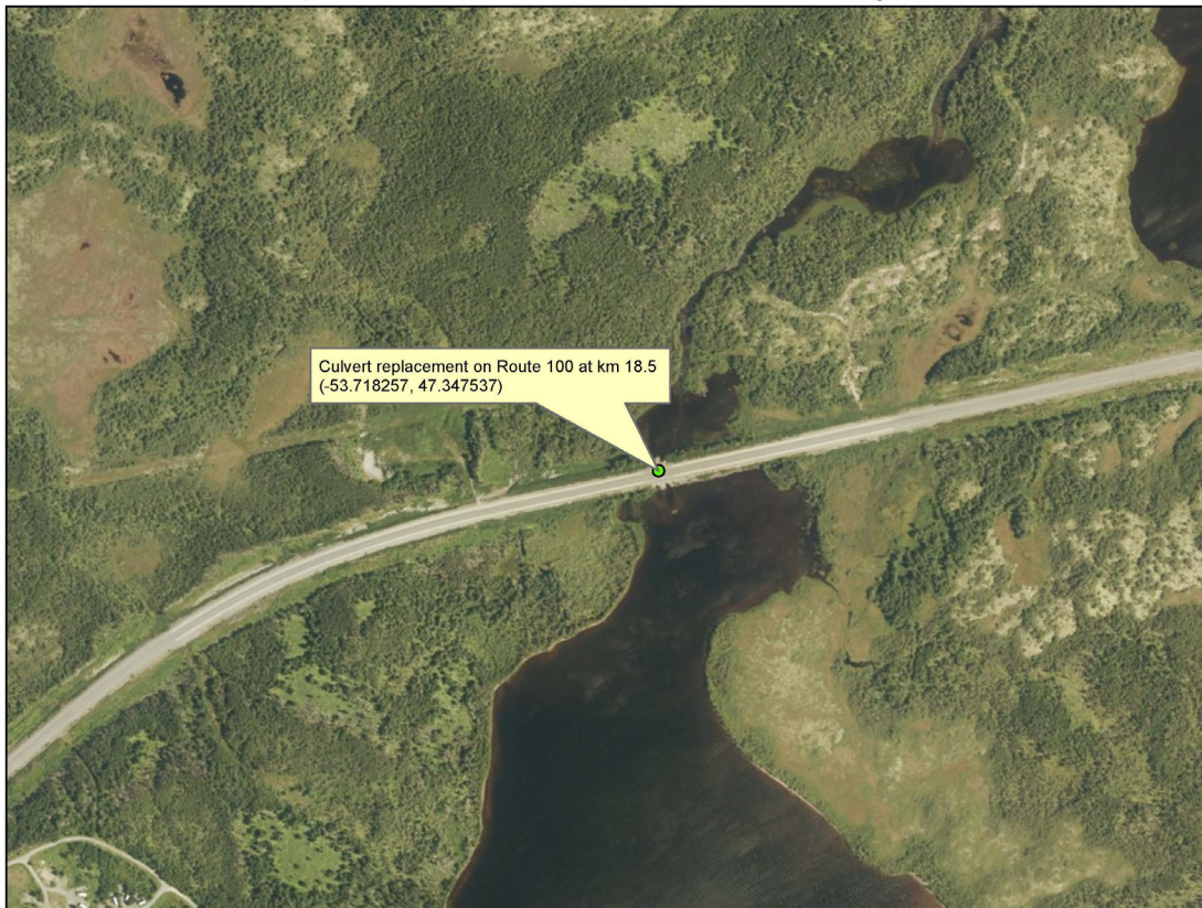
Culvert replacement on Route 100 at km 18.5 across Fitzgeralds Pond
