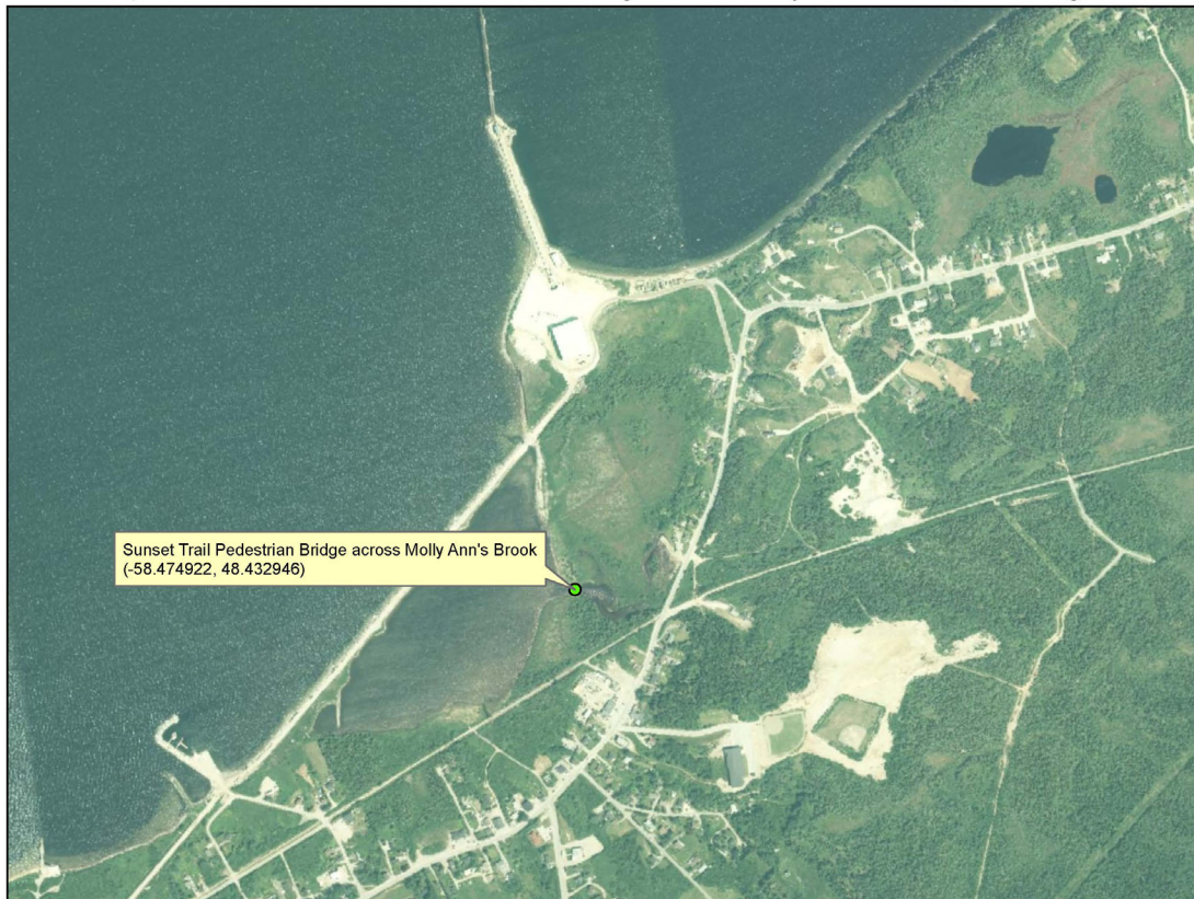
Replacement of Sunset Trail Pedestrian Bridge across Molly Ann's Brook, St. George's
