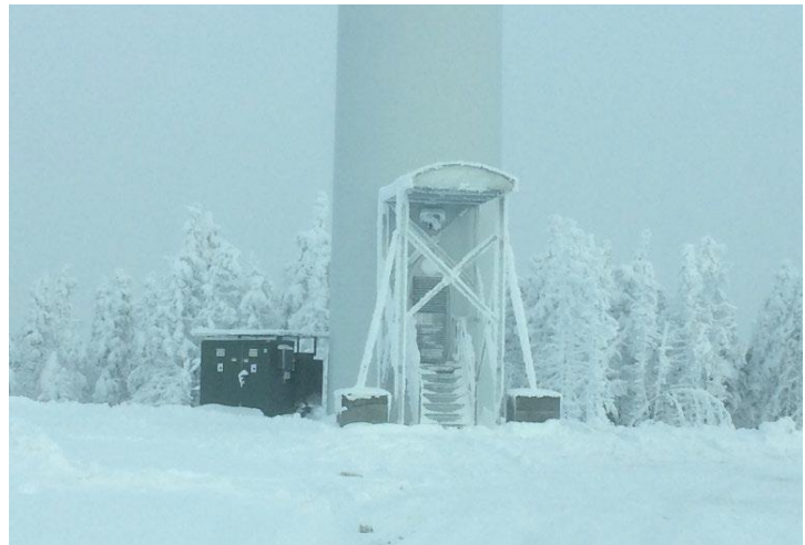
Figure L-2.3-1 Permanent ice protection device installed at wind turbine base (CanREA, 2020).
