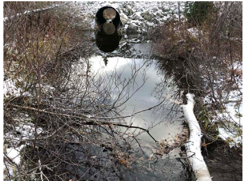
Photo 24 SS5 Looking Upstream (50m)
