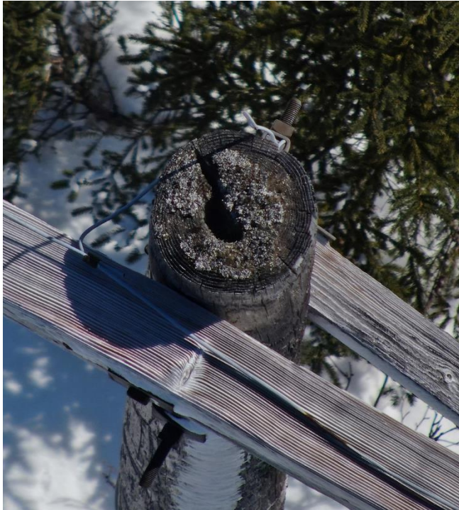
Figure 2 Void in a Pole Top demonstrates a hollow pole
