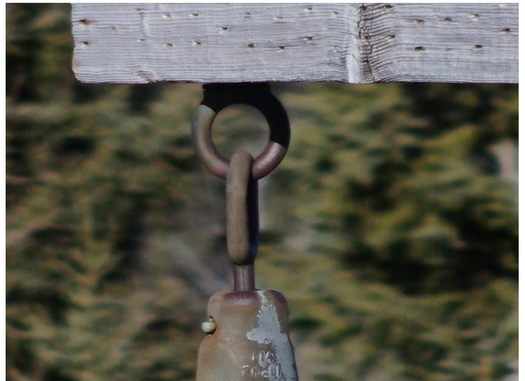
Figure 3 Insulator worn through a significant portion of eye bolt
