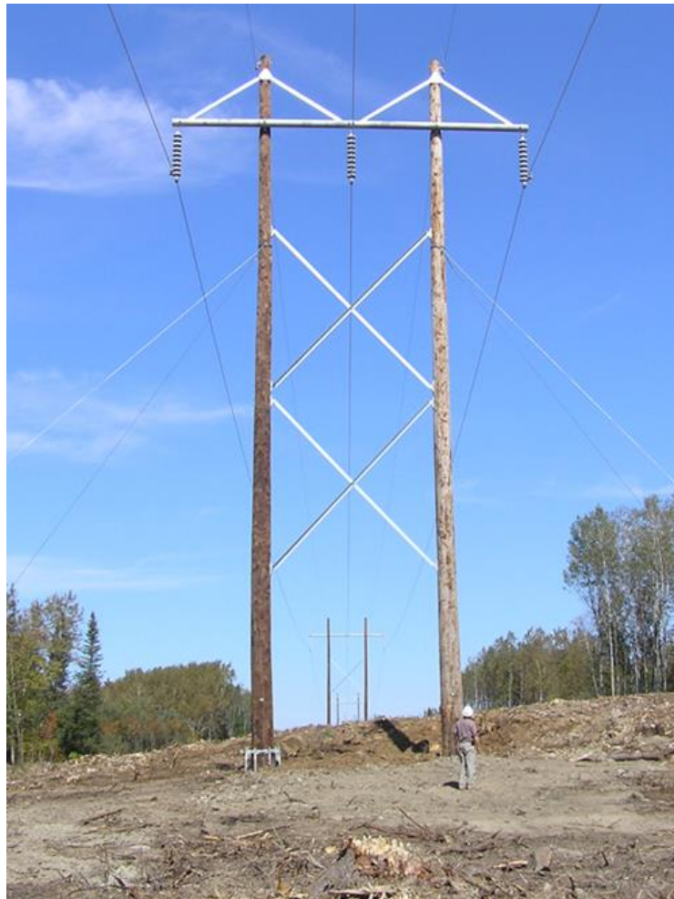
Figure 2-15: Typical H-Frame Transmission Structure (Wood and Steel)
