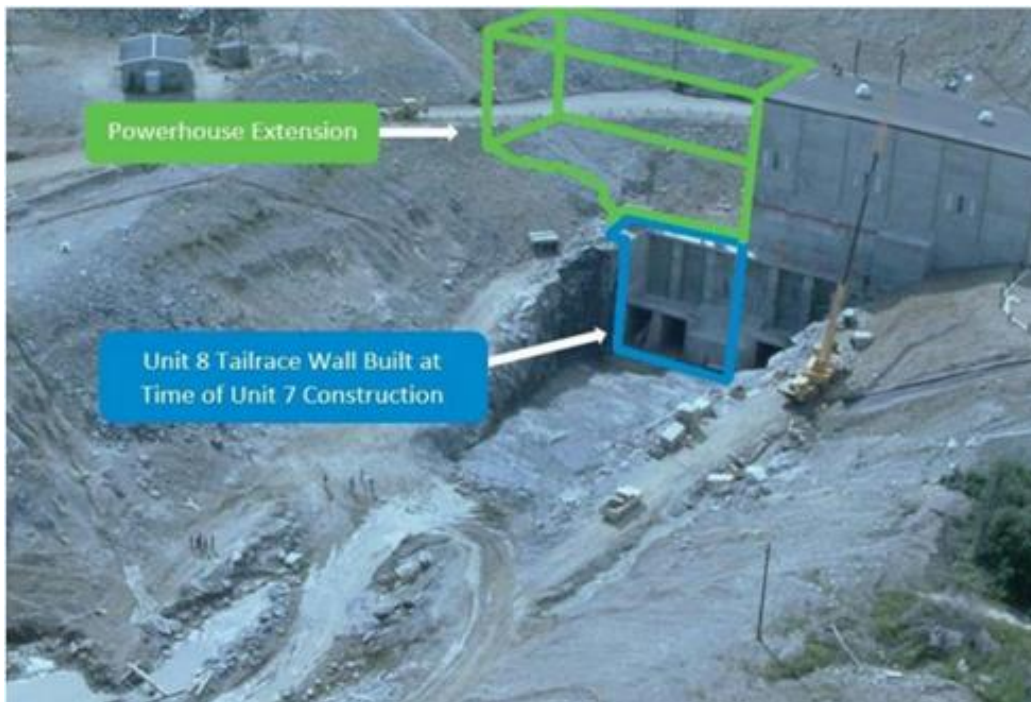
Figure 2-9: Existing Tailrace and the Draft Tube Outlet (Blue) for the Proposed Unit 8 Powerhouse 2 Extension (Green) at the Bay d'Espoir Hydroelectric Generating Facility
