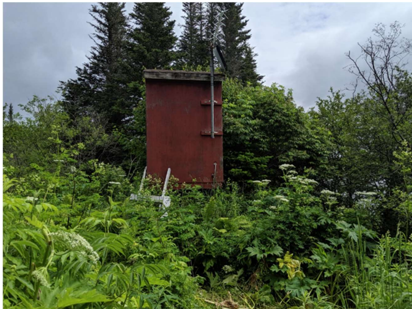
Figure 19. Former wooden walk-in shelter above the creosote stove stilling well prior to decommissioning (Photograph taken July 16, 2019).
