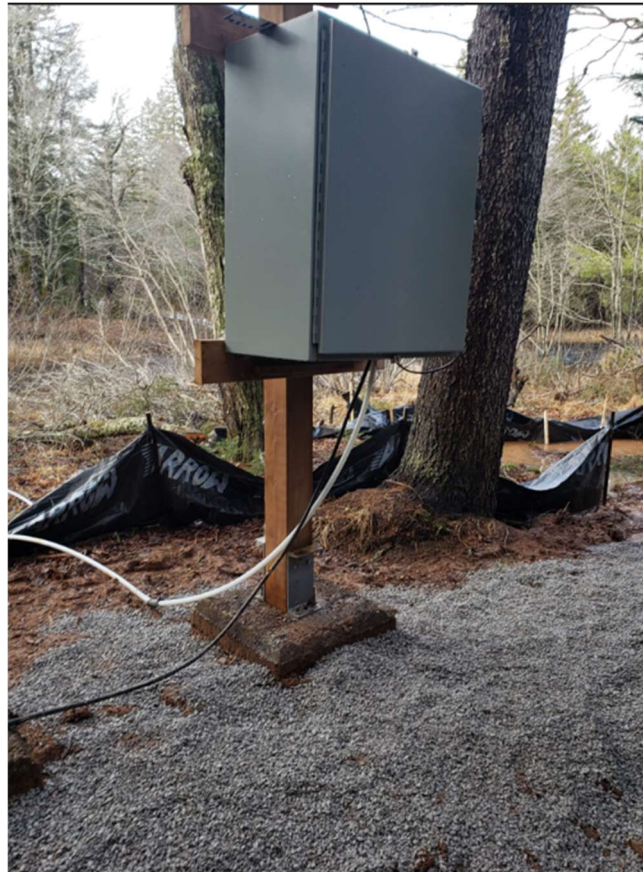
Figure 11. New look-in shelter on the right bank on the former cableway pedestal footing (Photograph taken December 21, 2022).
