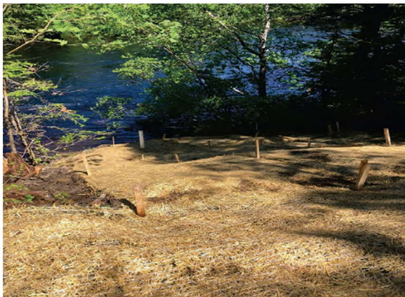
Figure 16. View following reinstatement of the former shelter/stilling well area with a biodegradable erosion control blanket (Photograph taken June 20, 2022).
