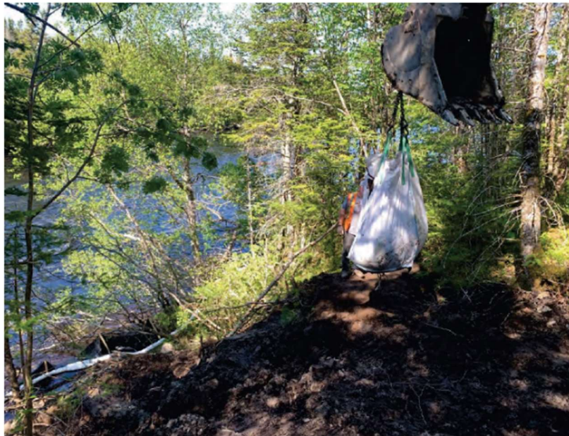
Figure 15. View during the removal of the petroleum hydrocarbon (PHC) impacted soil from near the stilling well (Photograph taken June 15, 2022).
