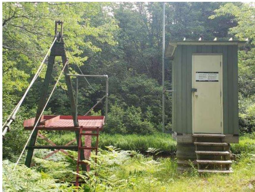
Figure 7. Shelter and an A-frame of the cableway on the left bank at 01DL001 (photograph taken July 22, 2020).
