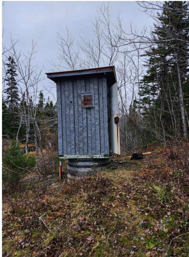
Figure 12. Stilling well and walk-in shelter at 01FJ002 MacAskills Brook near Birch Grove (Photograph taken November 20, 2023).
