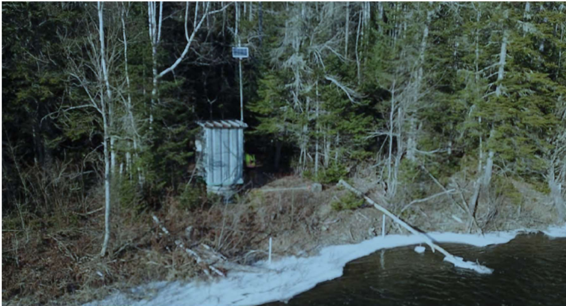
Figure 4. Stilling well structure as viewed from south side of river.
