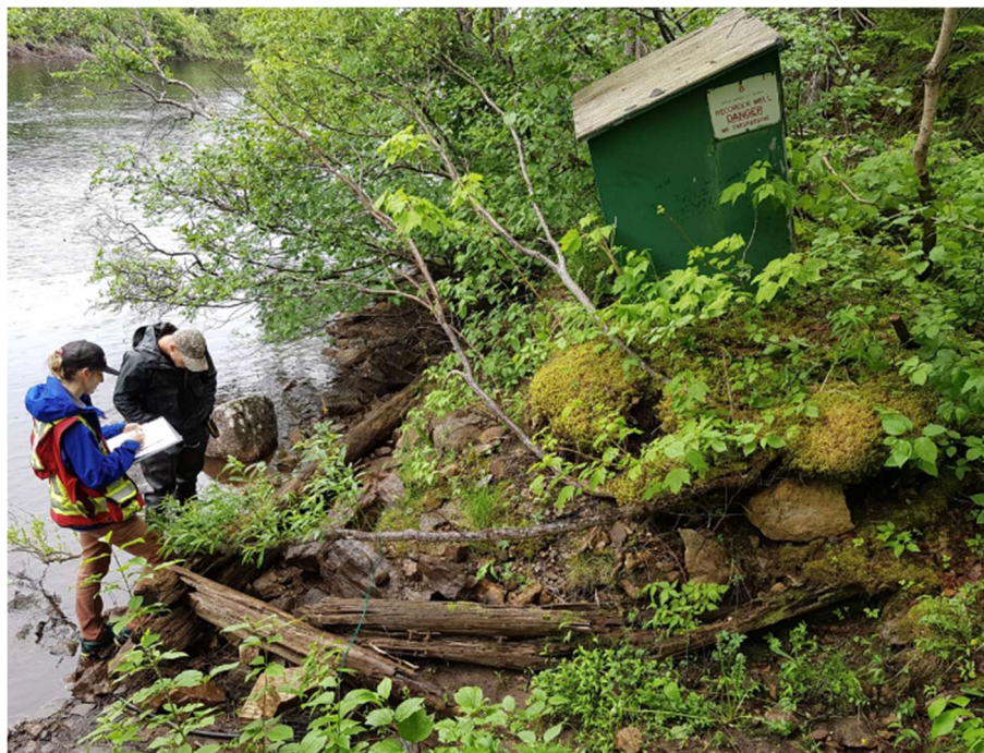
Figure 14. View of the inactive stilling well and shelter and creosote timber cribbing prior to decommissioning (Photograph taken July 15, 2019).
