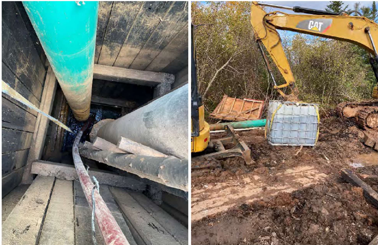
Figure 21. View during the removal of the petroleum hydrocarbon (PHC) and PAH impacted groundwater from the stilling well on October 12, 2022.
