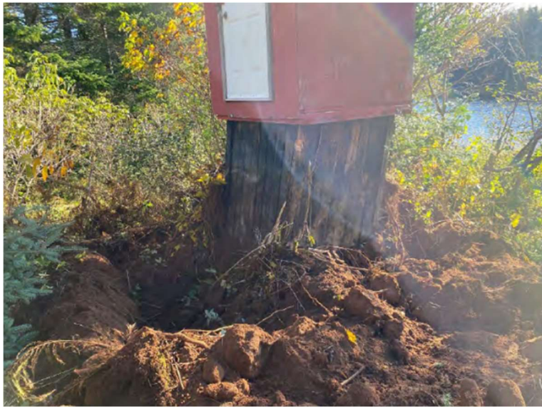
Figure 20. View during the removal of the creosote-treated stilling well, wooden shelter, and impacted soil adjacent to the stilling well on October 12, 2022.
