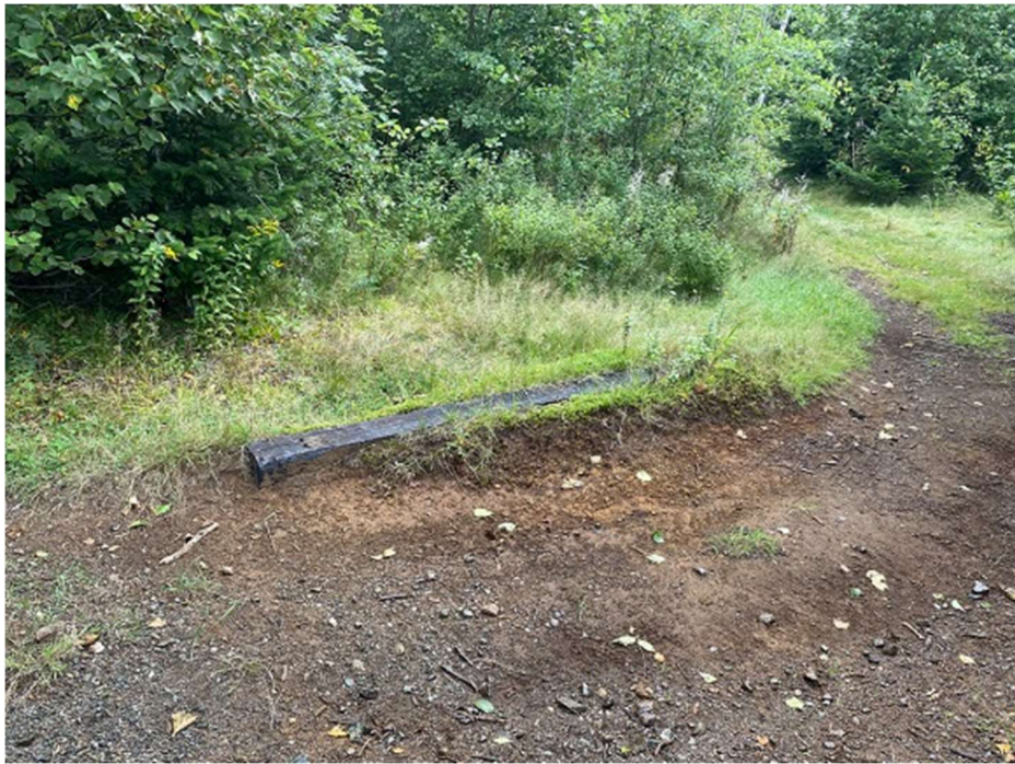
Figure 24. Creosote timber footing of the former cableway (Photograph taken September 16, 2022).
