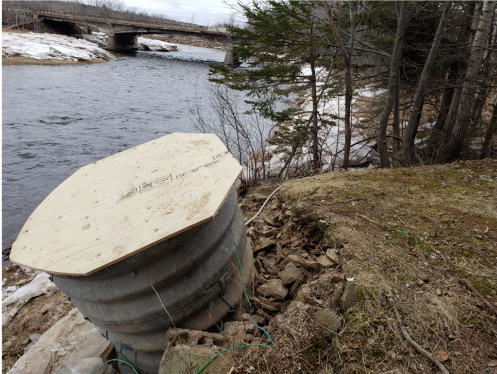
Figure 6. Damaged stilling well at 01BU002 Petitcodiac River near Petitcodiac (Photograph taken March 16, 2022).
