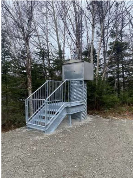
Figure 20. New corrugated metal standpipe and dog-house style look-in shelter with metal stairs/platform at 02YR003.
