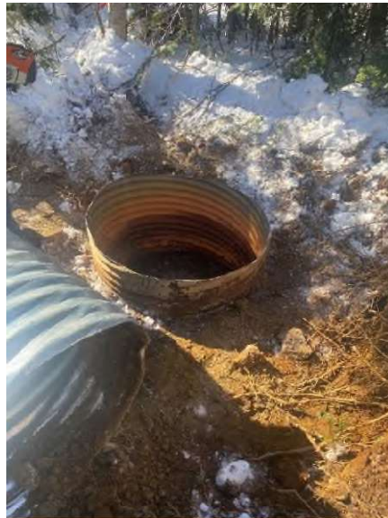
Figure 18. View of the cutdown stilling well during decommissioning at 02YR003 (Photograph taken on February 21, 2024)
