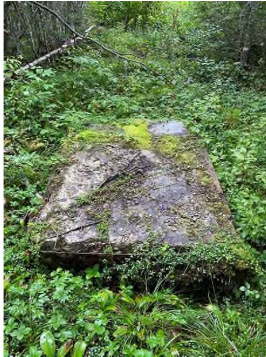
Figure 16. Concrete mass anchor from former cableway at 02YR003 (Photograph taken September 16, 2022).
