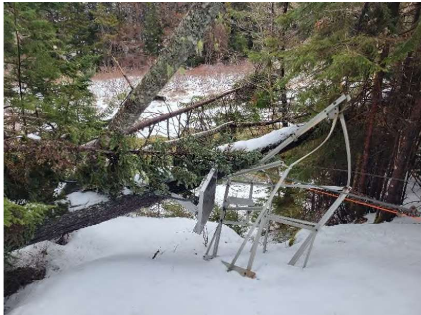
Figure 8. View of cableway with fallen tree overtop at 01BV006 Point Wolfe at Fundy National Park (Photograph taken in March 2023).
