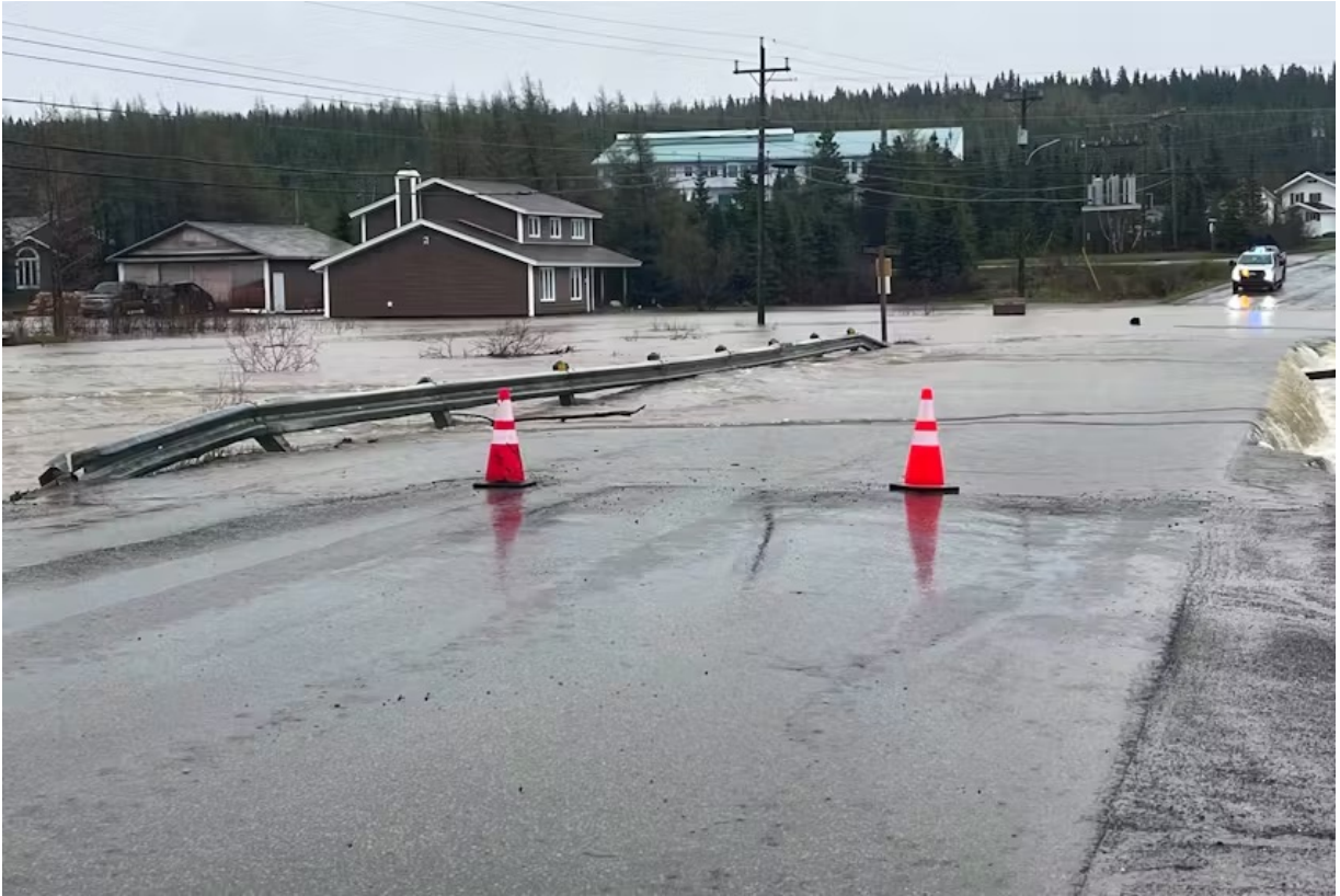
Figure 2.2 Road washout on the Northern Peninsula – Roddickton on June 10 th , 2023. (Photo Credit: Government of Newfoundland and Labrador Staff)
