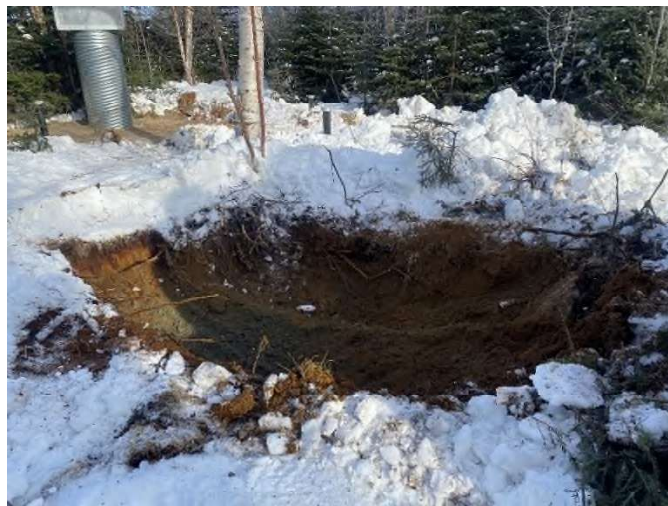
Figure 19. View following the removal of the PAH impacted soil on the northside of the site at 02YR003 (Photograph taken on February 22, 2024)
