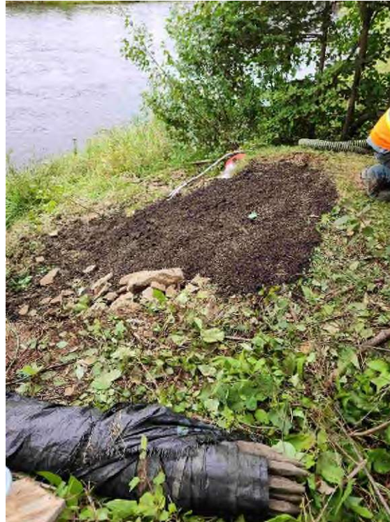
Figure 1. Topsoil overlaid on the decommissioned well at 01BU002 Petitcodiac River near Petitcodiac (photograph taken on September 9th, 2023).
