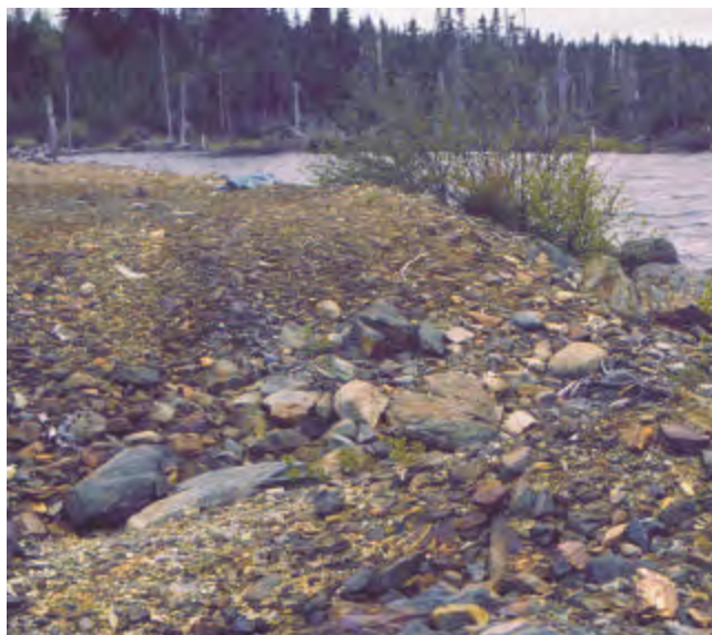
Plate 1. Looking southwest from tailings pond across breach in dyke into Little Rambler Pond. Note the abundance of weathering, sulphide-rich, waste rock used in dyke construction.
