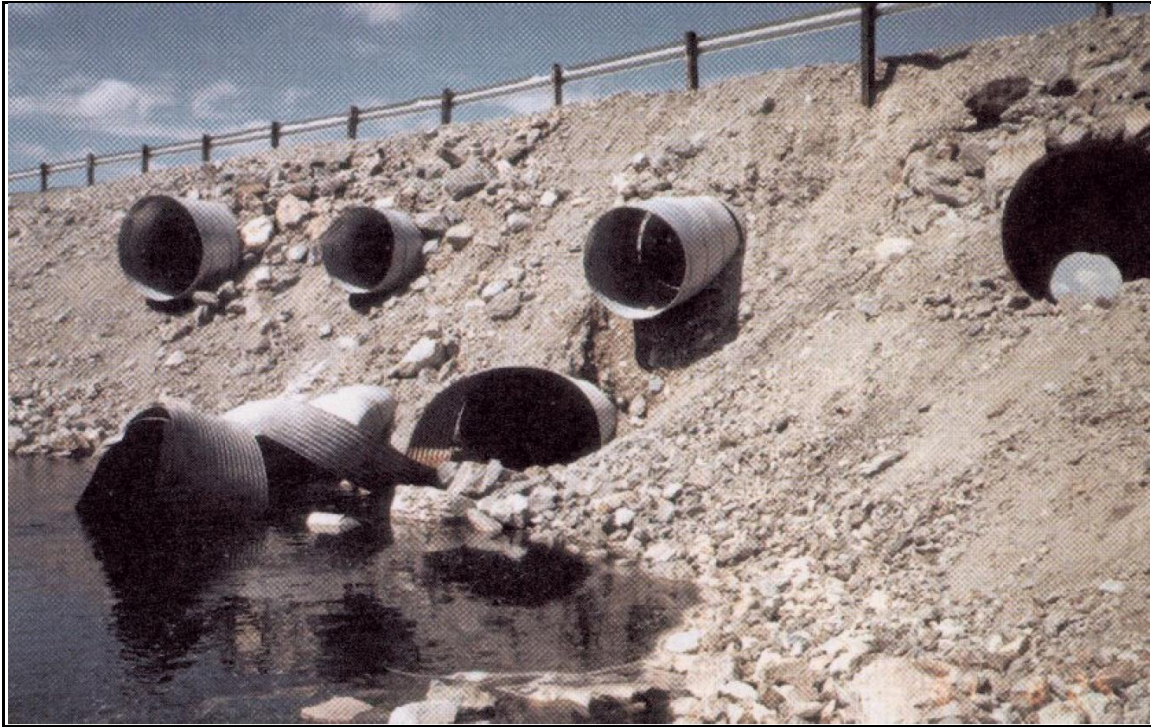
Figure 5.7 Poorly Installed Culverts
