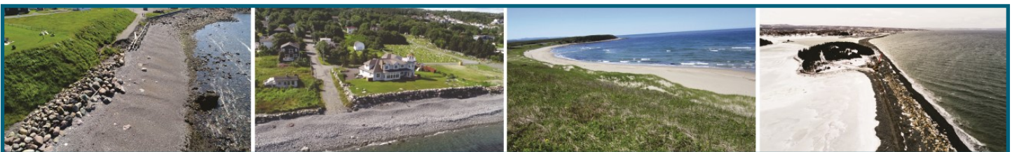
Examples of 'hard' coastal protection: Left- revetment at Fortune; centre left- boulder retaining wall, CBS . Examples of 'soft' coastal protection: Centre right-dune stabilisation, Gros Morne National Part, right – beach replenishment, CBS.
