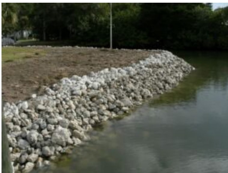
Figure 4-3: Riprap Placed Along a Slope (DFO, 2022)
