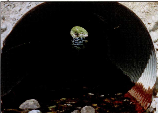
Figure 3. Countersunk Culvert
