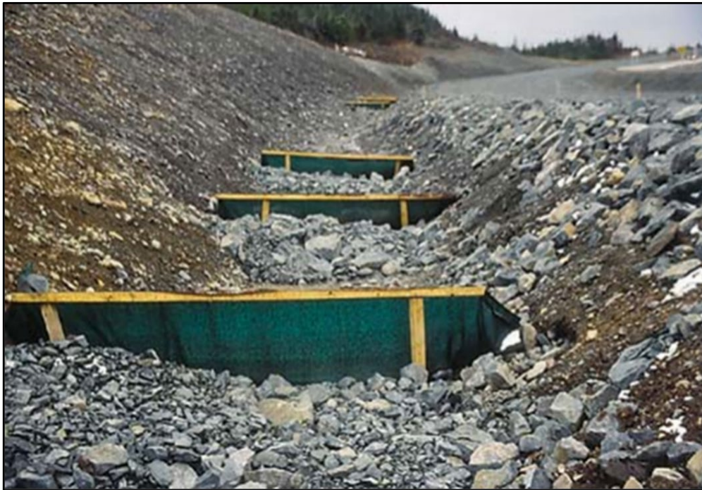
Figure 4-5: Filter Fabric Dams (Gosse et al. 1998; (DFO, 2022)
