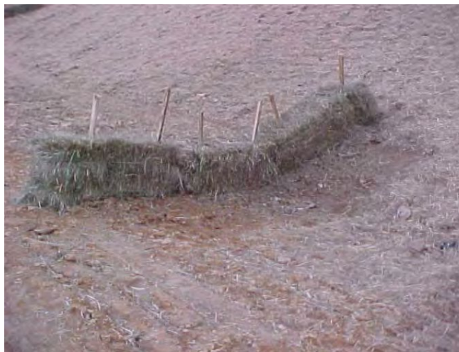
Figure 4-10: Anchored Straw Bale (Mississippi Department of Environmental Quality [MDEQ], n.d.)
