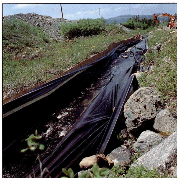
Temporary diversion - channel liner.
