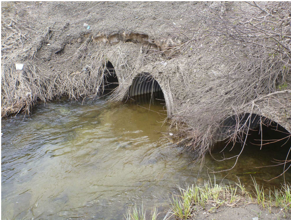
Figure 5-21: The Upper Reach of Tamarack-S1 at the Outflow of the Avalon Drive Culverts, June 5, 2013 (note the heavy sand and gravel from winter road ice control)
