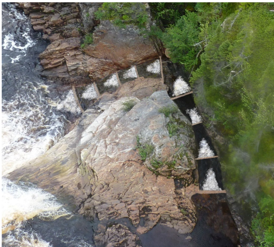
Figure 5-4: Fish Passage Concept with Concrete Baffles Creating Pools in the Run-Around Flow Pathway Occurring at the Falls Located at Kilometre 28
