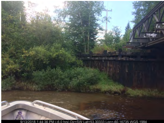
Sept. 13/18 – West side of channel at bridge (Photo #2)
