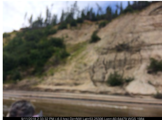
Sept. 11/18 – North Riverbank (Station 34+178)
