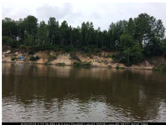
Aug. 30/18 – North Riverbank (Station 8+286)
