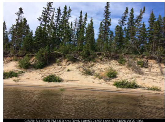
Sept. 5/18 – North Riverbank (Station 18+656)
