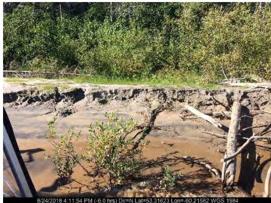
Aug. 24/18 – North Riverbank (Station 4+092)
