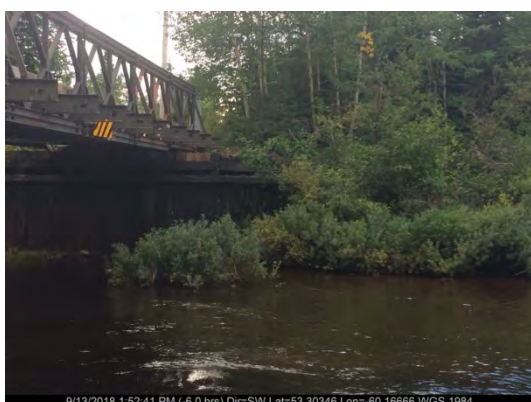
Sept. 13/18 – West side of channel at bridge (Photo #3)
