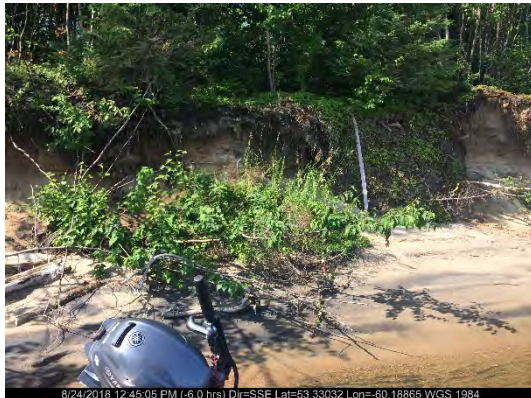
Aug. 24/18 - North Riverbank (Station 0+641)
