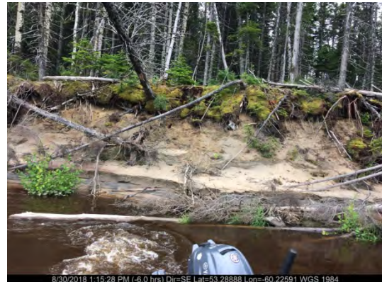
Aug. 30/18 – South Riverbank (Station 5+417)
