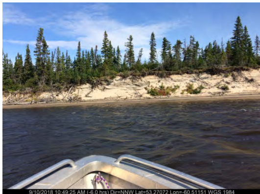
Sept. 10/18 – North Riverbank (Station 25+229)
