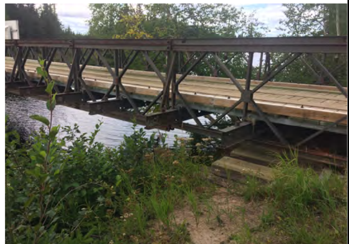
Bridge Photo 4 - Facing South East
