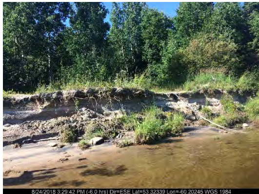
Aug. 24/18 - North Riverbank (Station 2+246)
