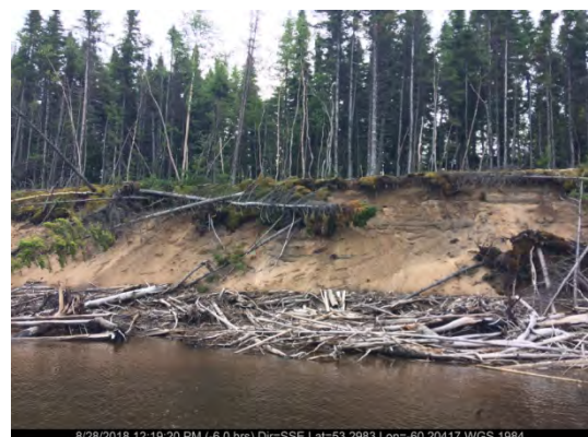
Aug. 28/18 – South Riverbank (Station 4+235)
