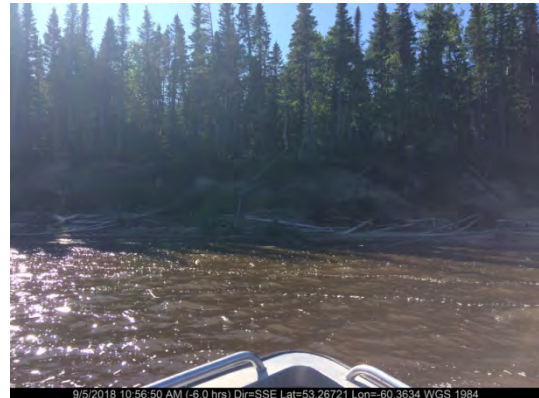
Sept. 5/18 – South Riverbank (Station 15+126)
