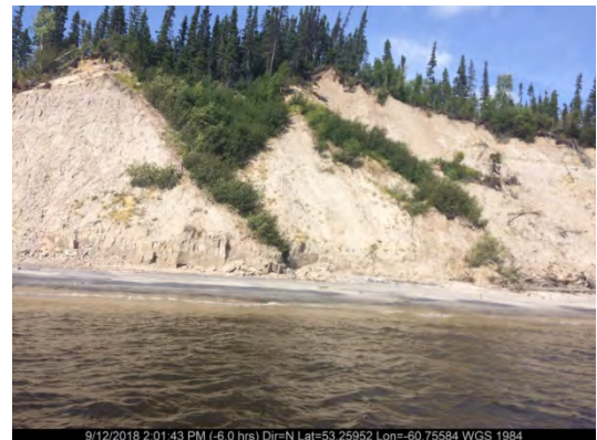
Sept. 12/18 – North Riverbank (Station 42+121)
