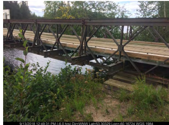
Mud Lake Bridge (Photo #6)
