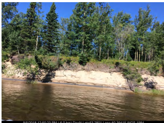
Sept. 5/18 – North Riverbank (Station 17+141)
