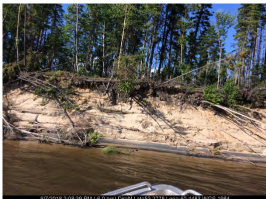
Sept. 7/18 – North Riverbank (Station 20+587)
