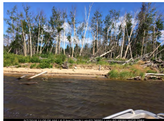
Sept. 7/18 – North Riverbank (Station 22+988)
