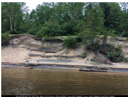
Aug. 30/18 – Facing south towards North side of island (Station 6+988)
