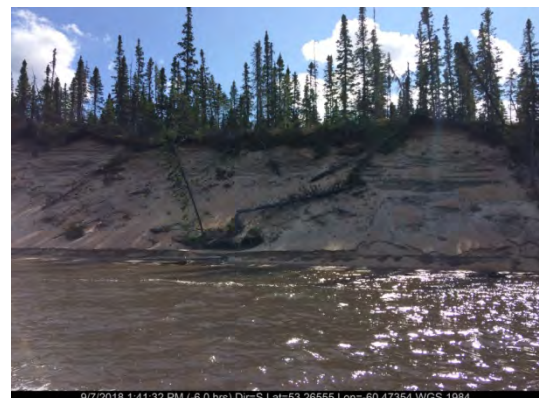
Sept. 7/18 – South Riverbank (Station 20+662)
