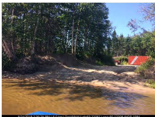
Aug. 24/18 - North Riverbank (Station 0+560)
