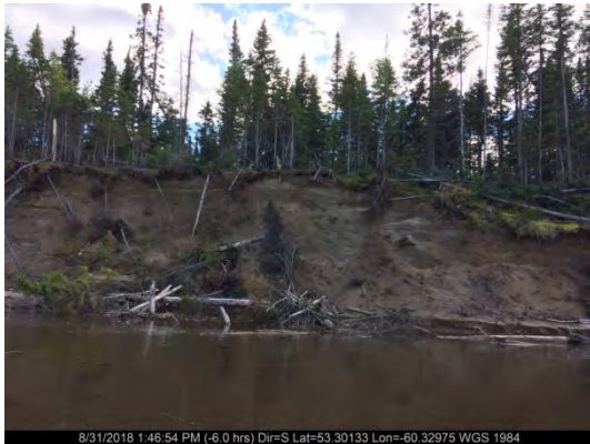
Aug. 31/18 – South Riverbank (Station 13+056)
