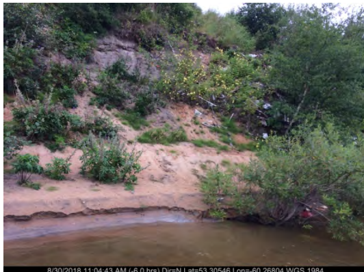
Aug. 30/18 – North Riverbank (Station 7+792)
