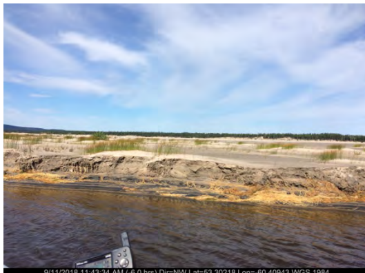
Sept. 11/18 – South side of sandbar (Station 17+624)
