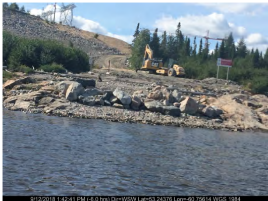
Sept. 12/18 – South Riverbank (Station 42+283)
