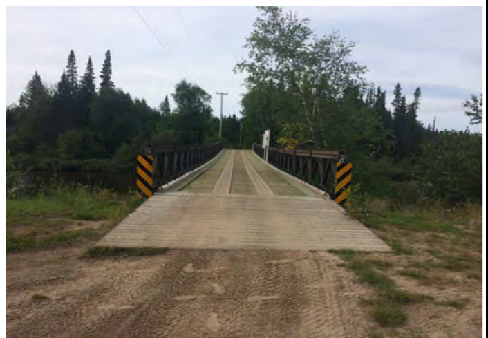
Bridge Photo 2 - Facing West
