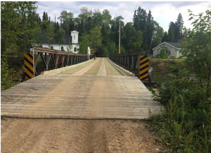
Bridge Photo 1 - Facing East
