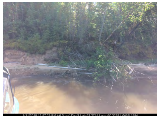
Aug. 31/18 – South Riverbank (Station 12+623)
