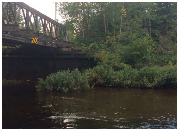
Bridge Photo 3 - North Side of Bridge
