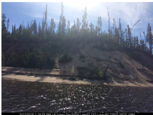
Sept. 12/18 – South Riverbank (Station 40+080)
