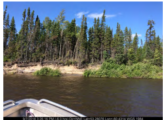
Sept. 7/18 – North Riverbank (Station 19+628)
