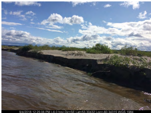
Sept. 4/18 – Facing SE along sandbar (Station 15+220)
