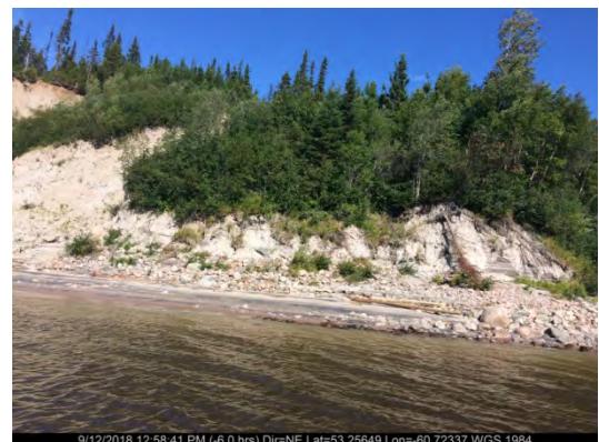
Sept. 12/18 – North Riverbank (Station 40+547)
