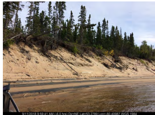
Sept. 11/18 – North Riverbank (Station 18+186)
