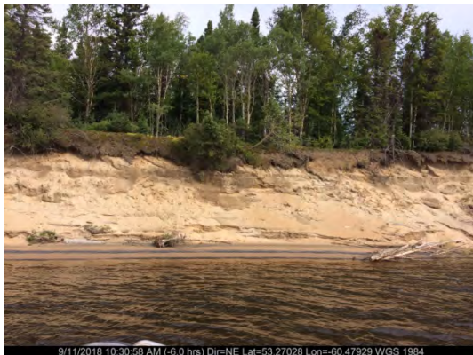
Sept. 11/18 – North Riverbank (Station 17+675)
