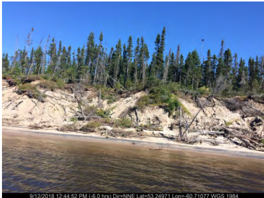
Sept. 12/18 – North Riverbank (Station 39+505)
