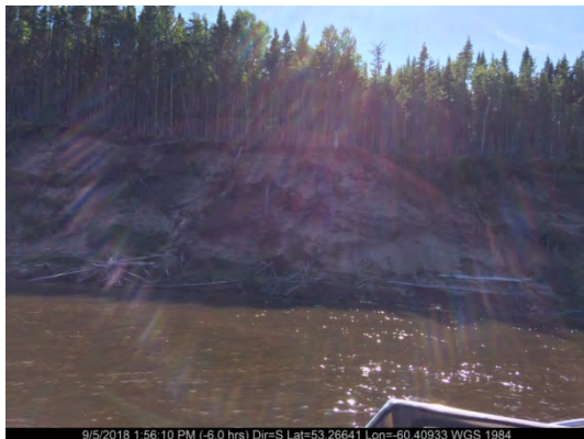
Sept. 5/18 – South Riverbank (Station 18+092)
