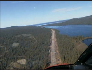
CLEARED RIGHT-OF-WAY - PHASE II
