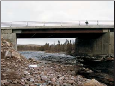
BRIDGE AT MARY'S HARBOUR
