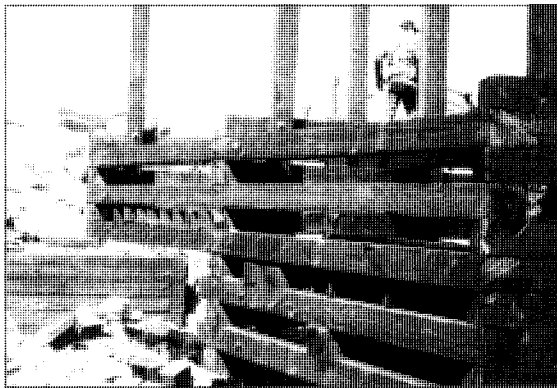
Timber crib construction for marine environment.
