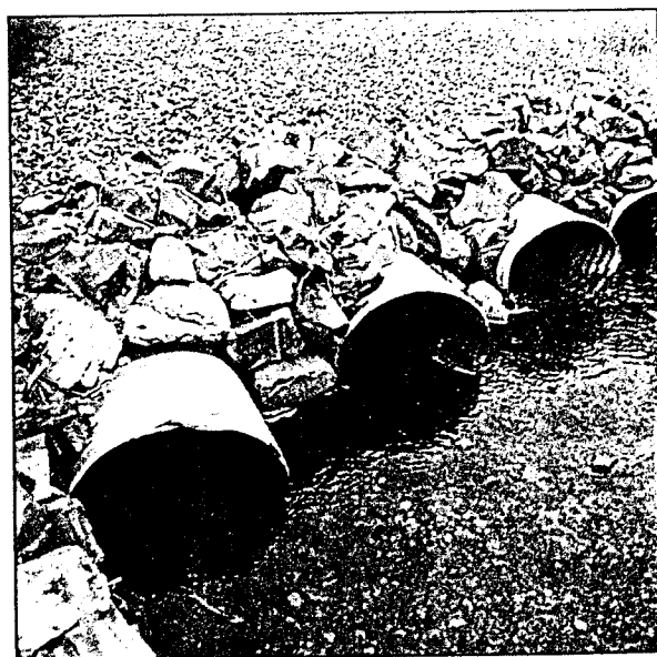
Stabilization of culvert outlets - rip rap.
