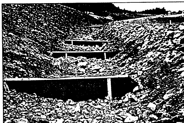
Filter fabric used for low point protection.
