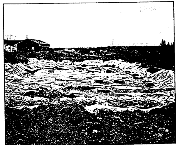
Settling basin lined with plastic.
