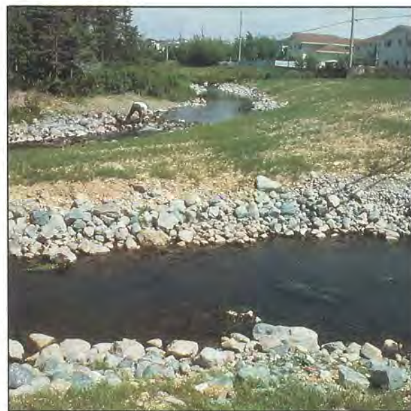
Stream bank stabilization using rip rap and hydroseed.
