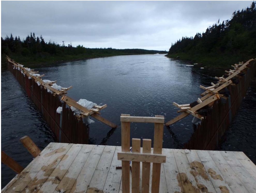
Figure 3.1. Downstream perspective of a typical counting fence used to monitor adult wild salmon returns in some Newfoundland and Labrador rivers (Photo courtesy of DFO).
