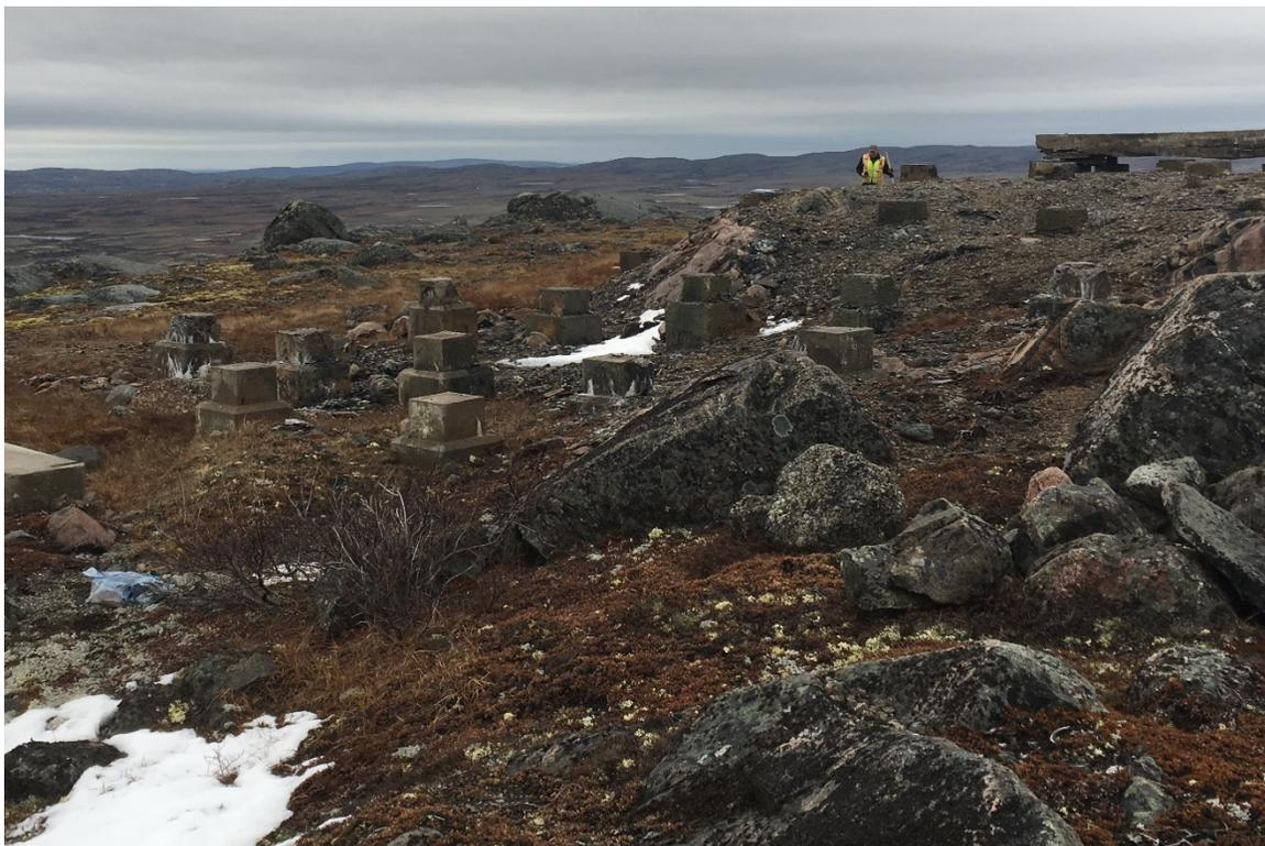
**Photo 18 – Upper Site: concrete slab and pillars of Former Operations Building. Looking southwest.**
