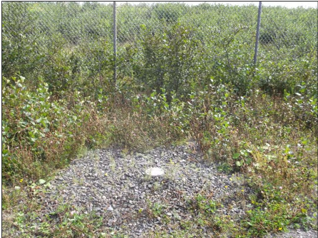
Photo 2: View, looking south, toward clean-out 2 near landfill fencing in the background. Note newly installed flush mount.
