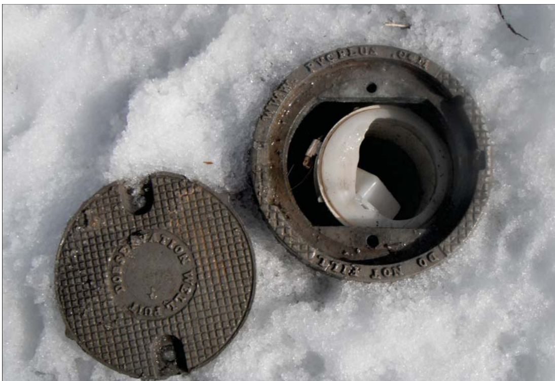
Photo 10 View of groundwater drainage system clean out CO2. Note the 4" drain cap is damaged.
