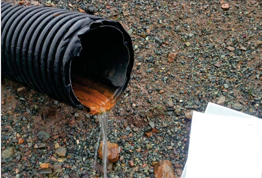
Photo 11 View of the groundwater drainage system outflow with visual evidence of iron floc deposits (December 2015).
