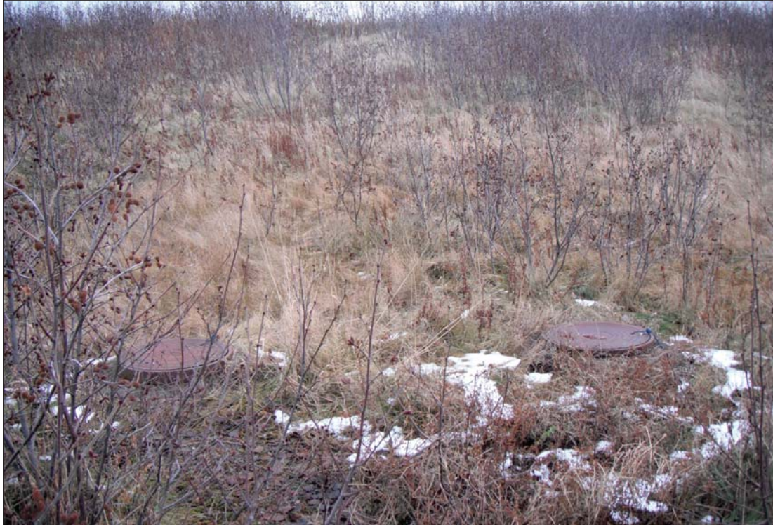
Photo 7 View, looking east, showing the vegetative overgrowth during the landfill cover inspection (December 2015).
