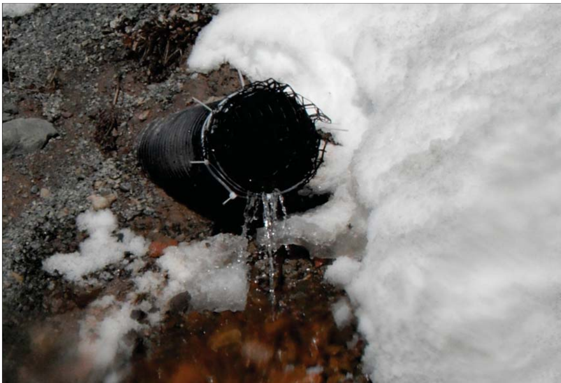
Photo 12 View of the groundwater drainage system outflow with a new rodent screen installed (March 2016).
