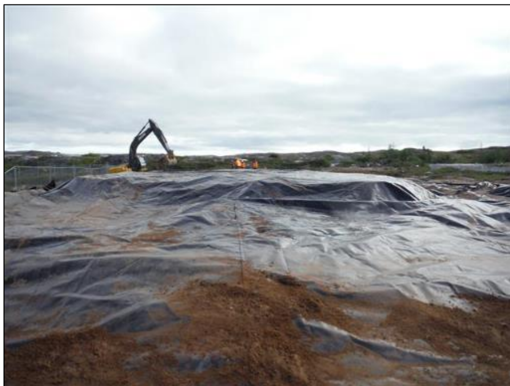
Photo 5 Securing the cover on the biopile, August 29, 2015.
