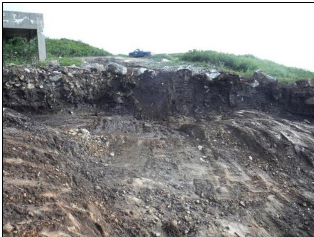
Photo 18 Soil removal at Main Base-Area 1, looking north, August 24, 2015.
