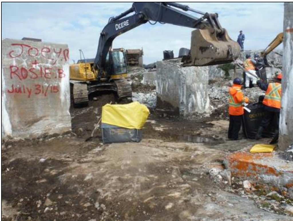
Photo 22 Soil removal at Main Base-Area 1, August 24, 2015.
