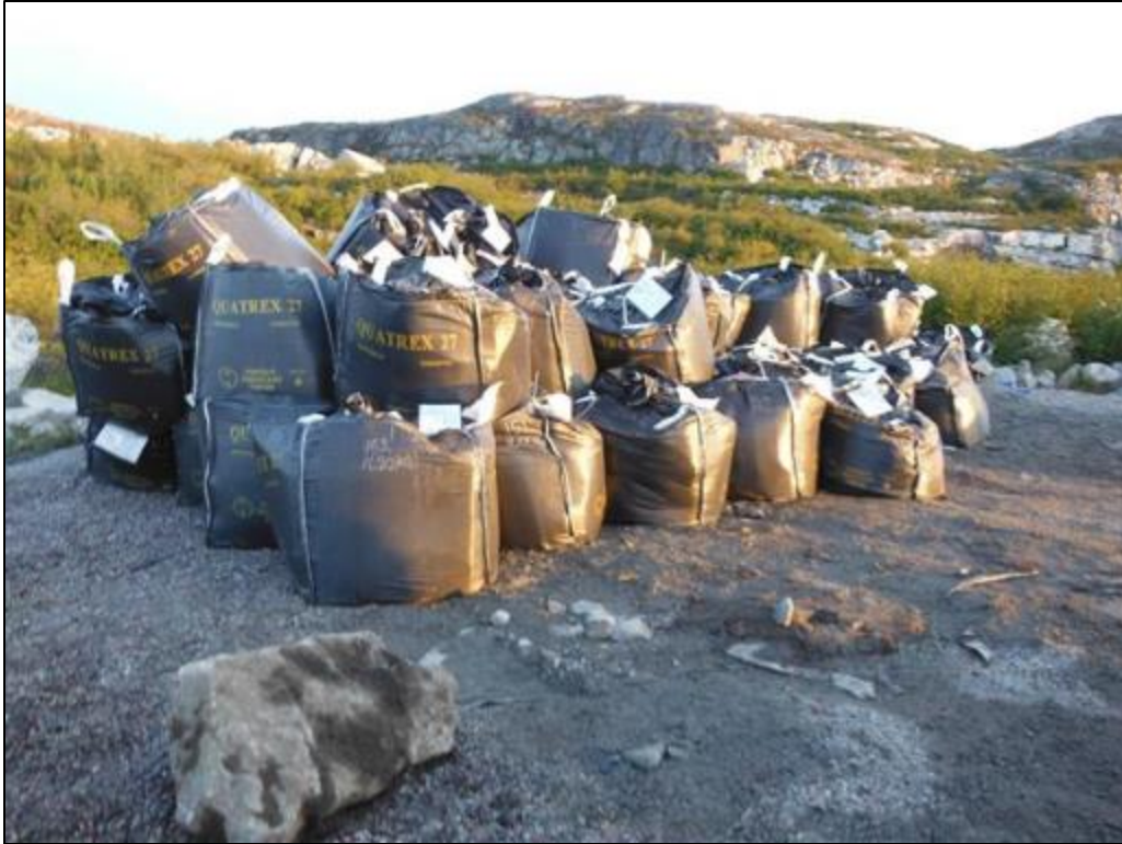
Photo 58 Pit No. 1, Staging Area for the storage of impacted soil bags, September 16, 2015.
