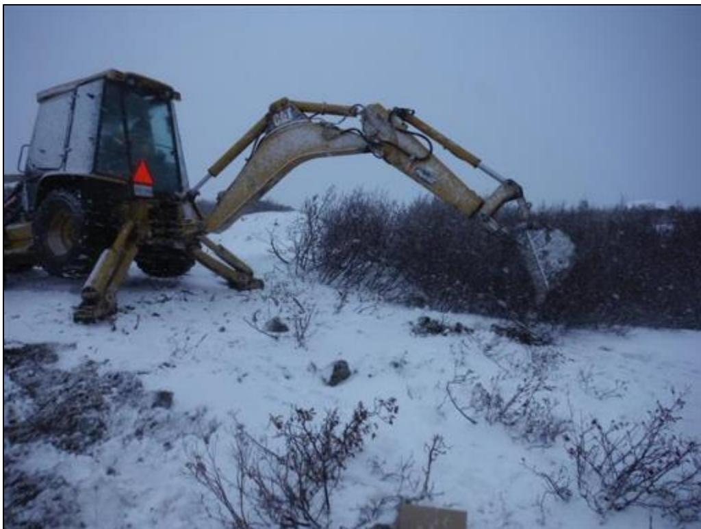
Photo 30 Additional delineation at Main Base-Area 1, October 30, 2015.
