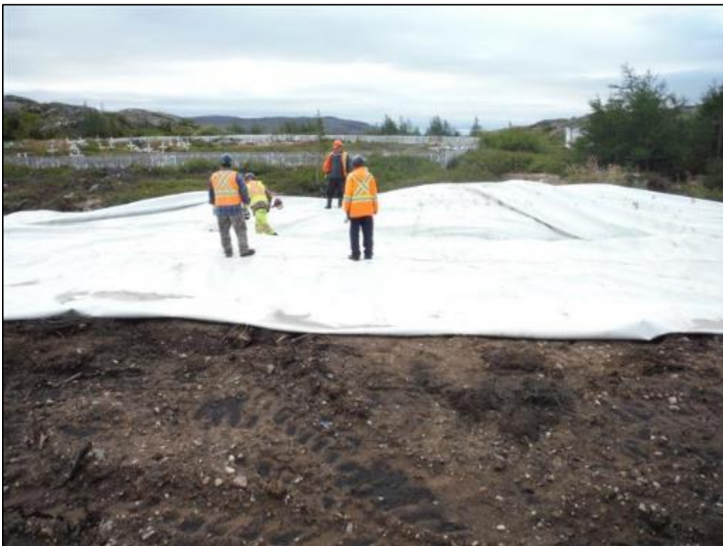
Photo 4 Placing the cover on the biopile, August 29, 2015.
