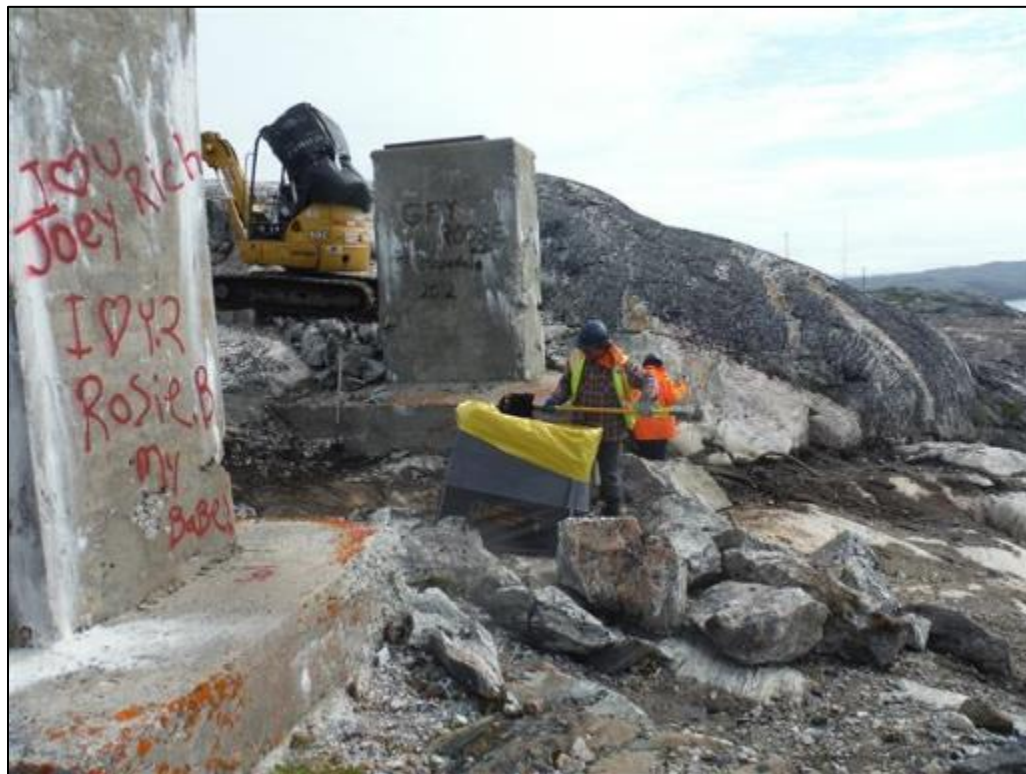
Photo 20 Soil removal at Main Base-Area 1, looking southeast, August 24, 2015.
