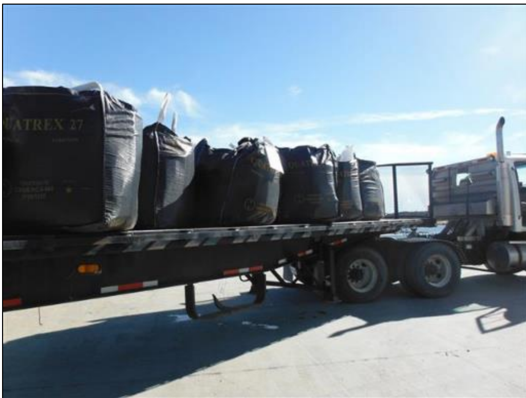
Photo 54 Transport of impacted soil bags by a flat bed truck from Pit No. 1 to the dock, September 14, 2015.
