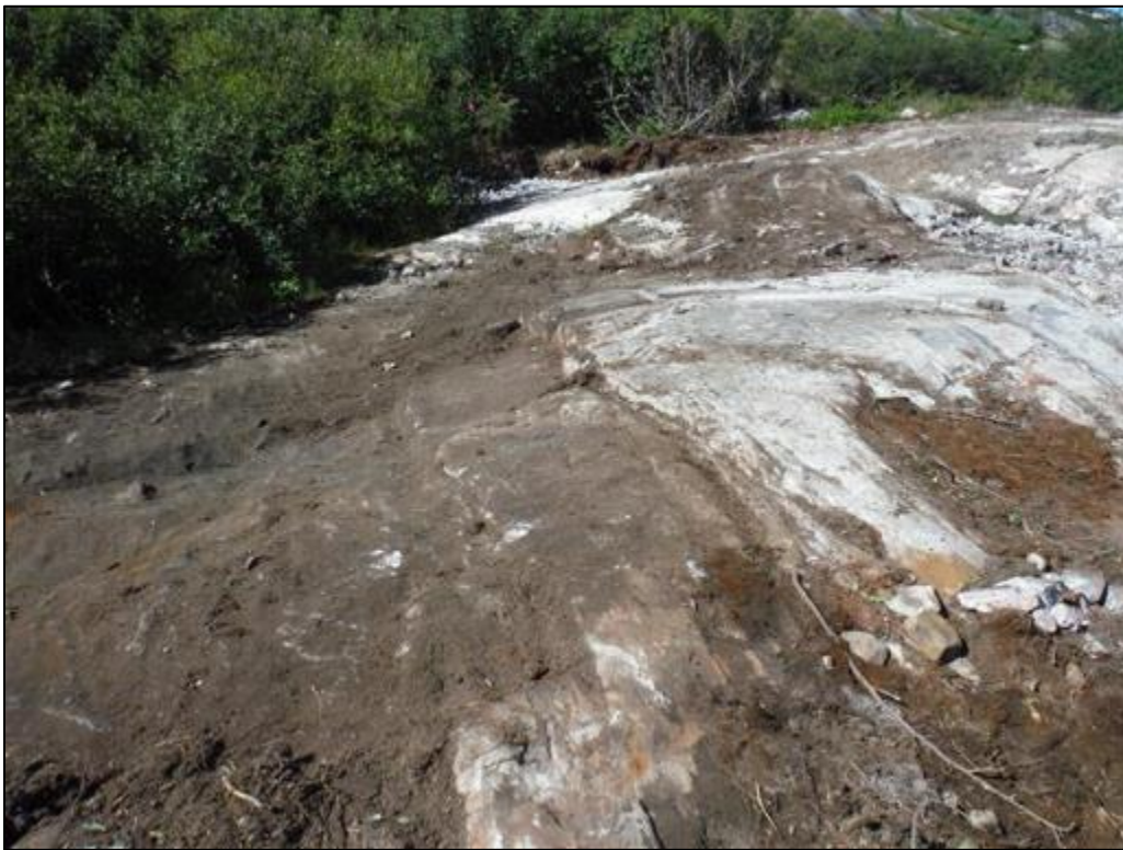
Photo 33 POL Compound-Area 3 following soil removal, looking northwest, August 30, 2015.
