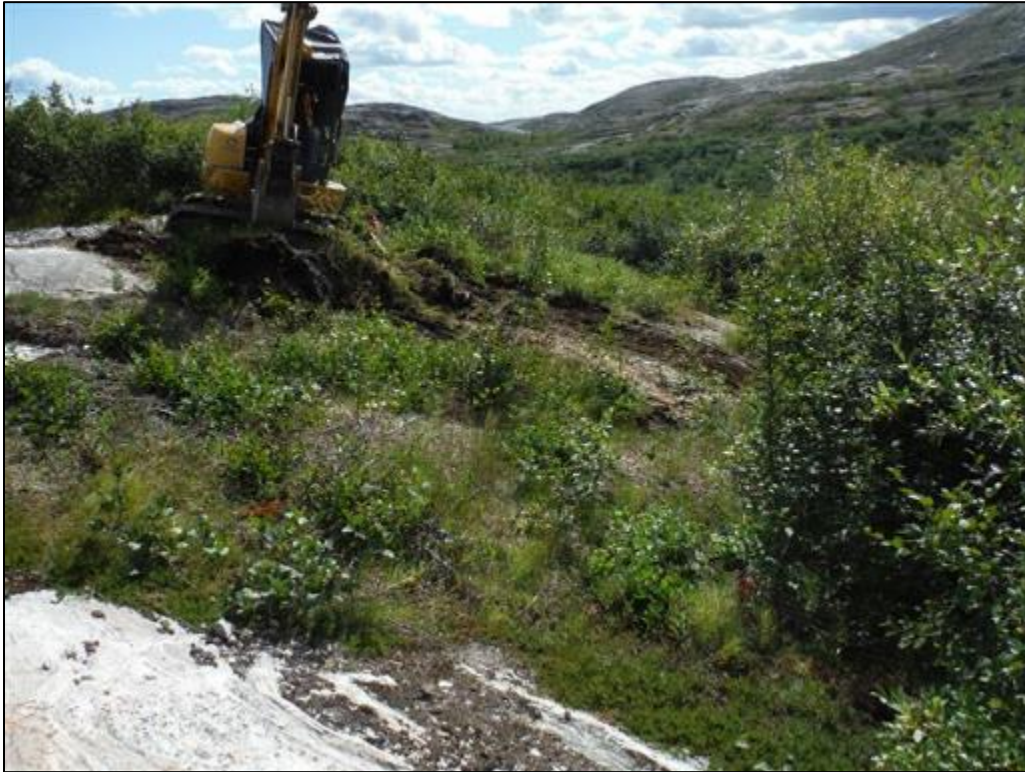
Photo 32 Soil removal at POL-Area 3, looking southeast, August 30, 2015.
