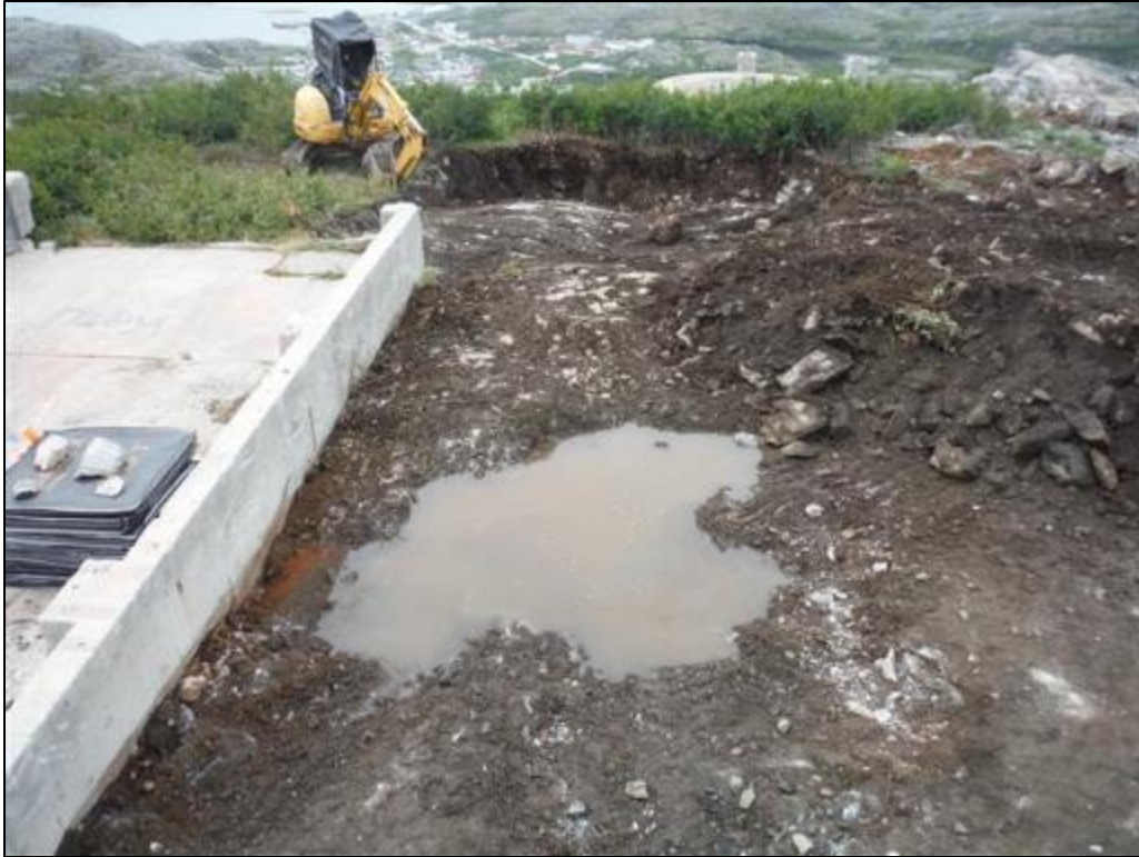
Photo 25 Soil removal at Main Base-Area 2, looking south, August 26, 2015.
