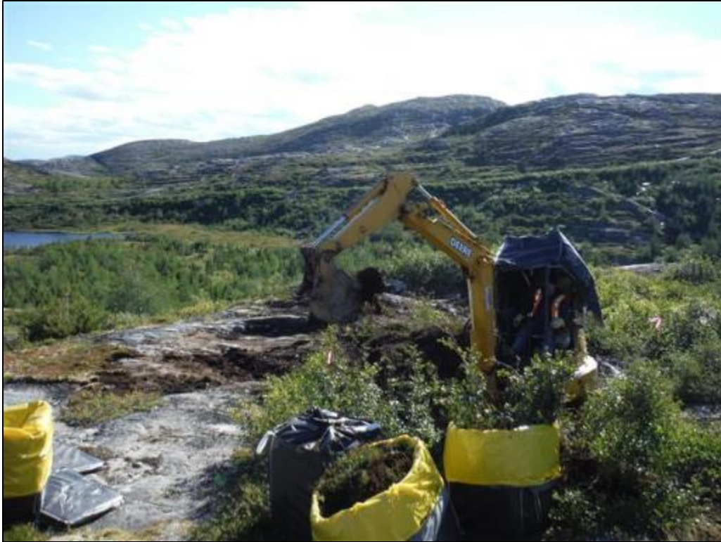
Photo 34 Soil removal at POL-Area 4, looking southwest, August 30, 2015.
