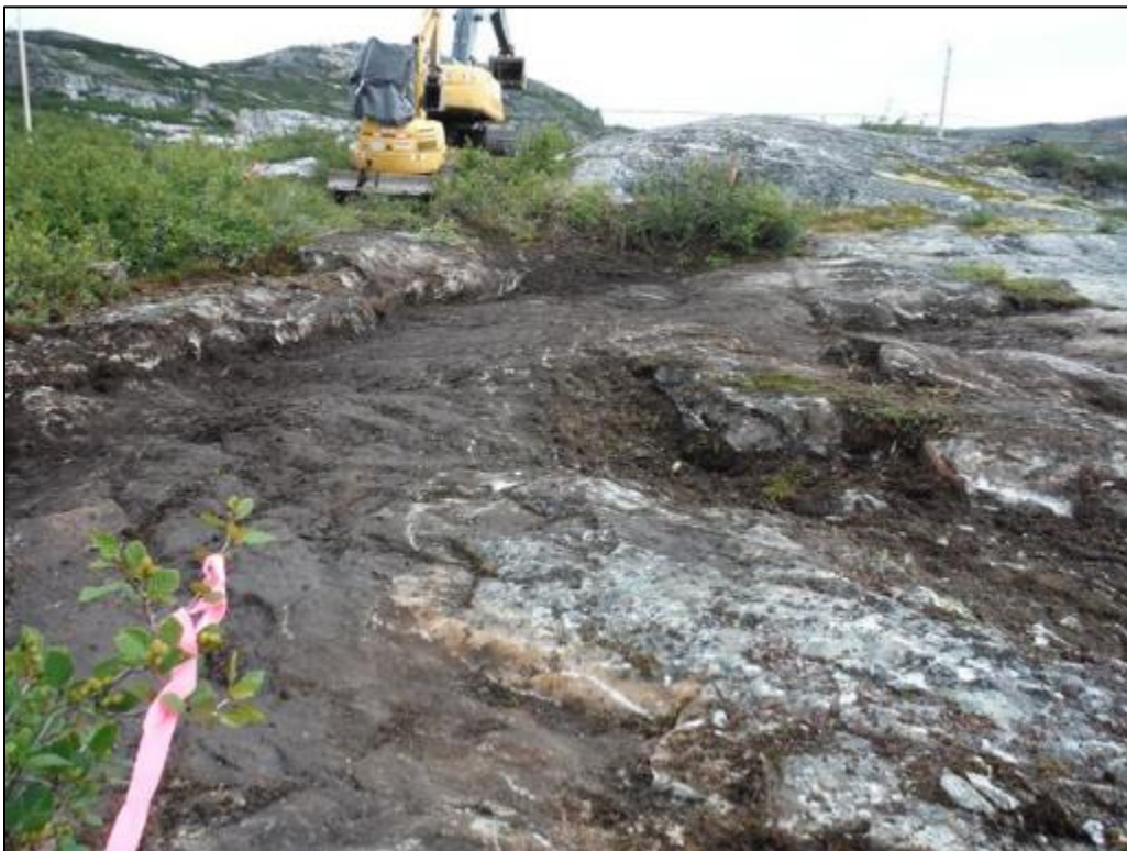
Photo 37 POL Compound-Area 4 following soil removal, looking north, August 30, 2015.
