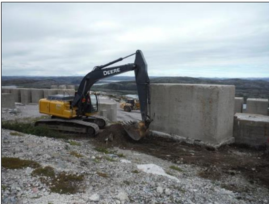
Photo 9 Soil removal at BMEWS-Area 5, August 29, 2015.
