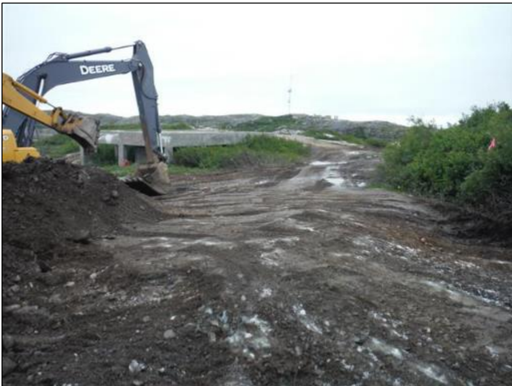
Photo 24 Soil removal at Main Base-Area 2, looking west, August 25, 2015.
