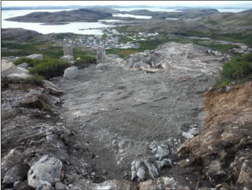
Photo 27 Remedial excavation backfilled at Main Base-Area 1, September 1, 2015.
