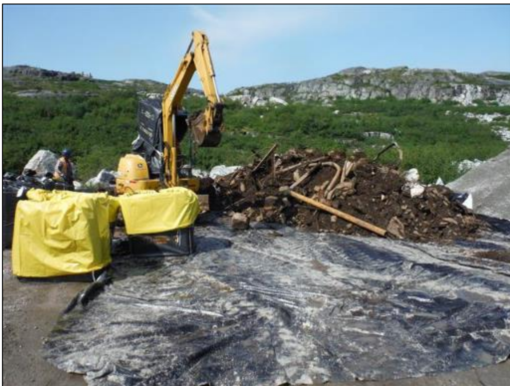
Photo 42 Separating metal debris and filling bags with impacted soil at Pit No. 1, August 21, 2015.
