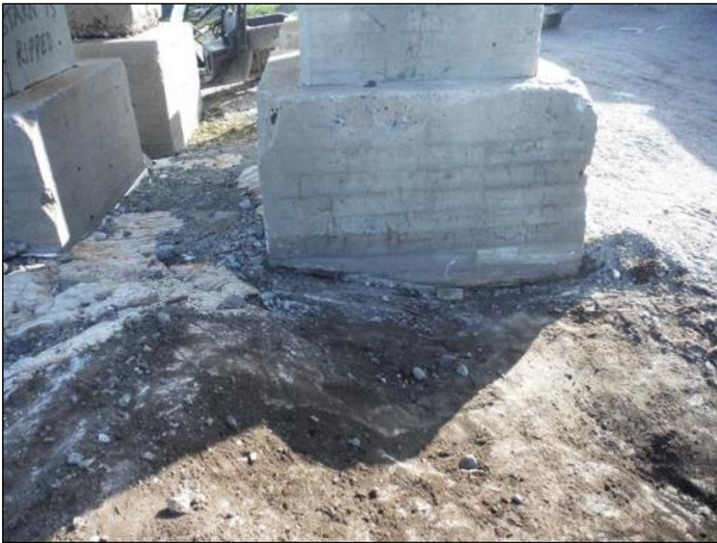
Photo 8 Soil removal at BMEWS-Area 4, August 19, 2015.
