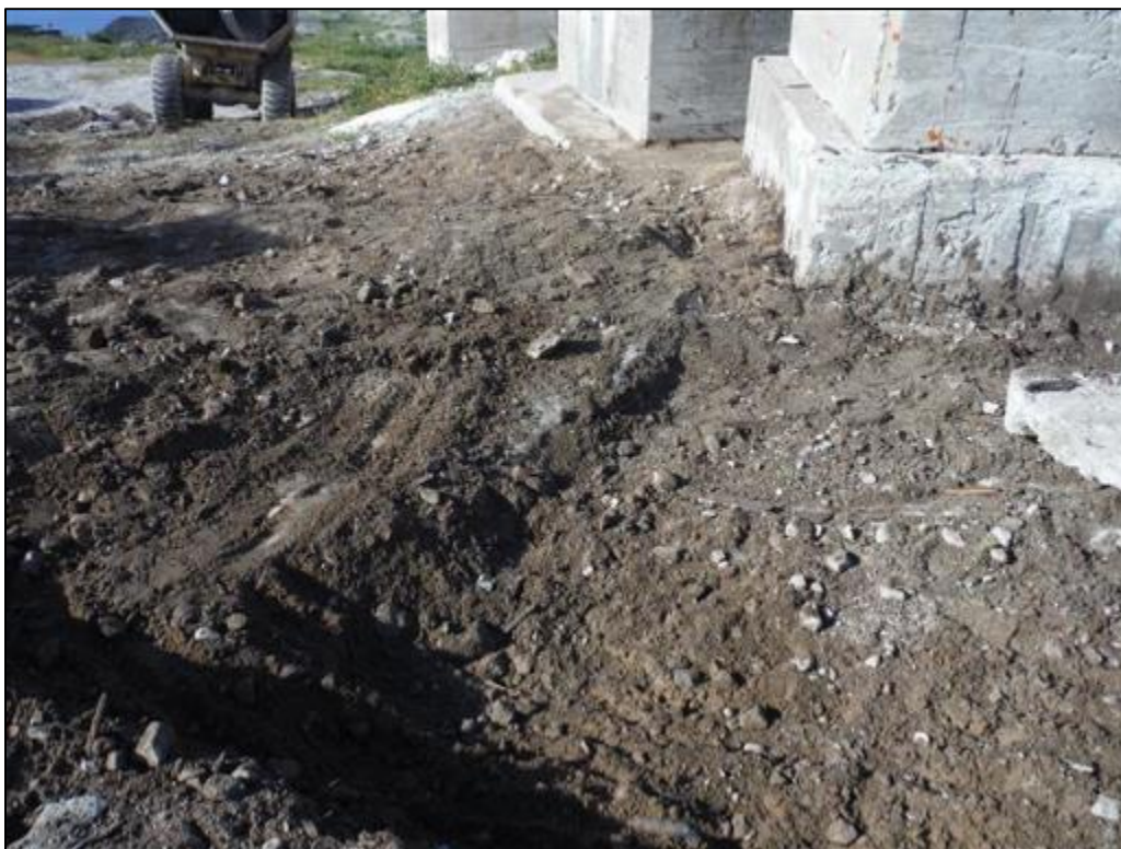
Photo 10 Soil removal at BMEWS-Area 5, August 29, 2015.
