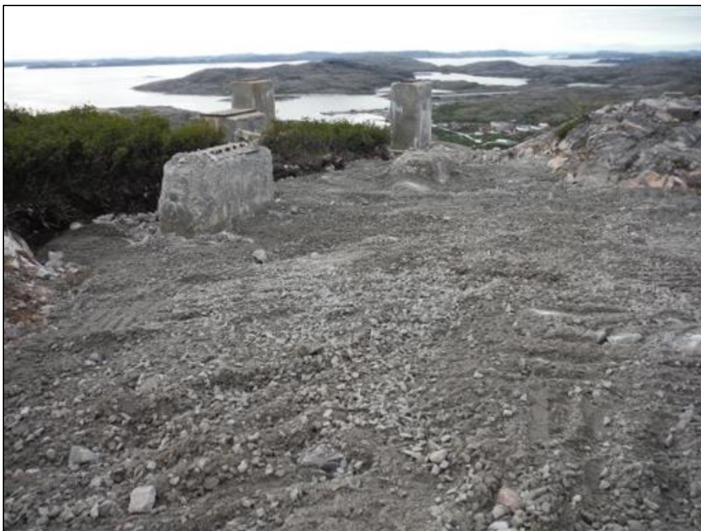
Photo 29 Remedial excavation backfilled at Main Base-Area 1, September 1, 2015.
