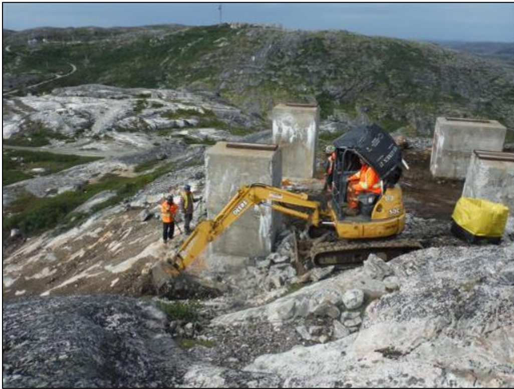
Photo 19 Soil removal at Main Base-Area 1, looking east, August 24, 2015.
