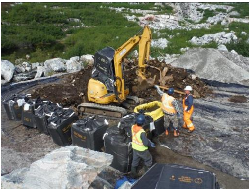
Photo 43 Separating metal debris and filling bags with impacted soil at Pit No. 1, August 21, 2015.
