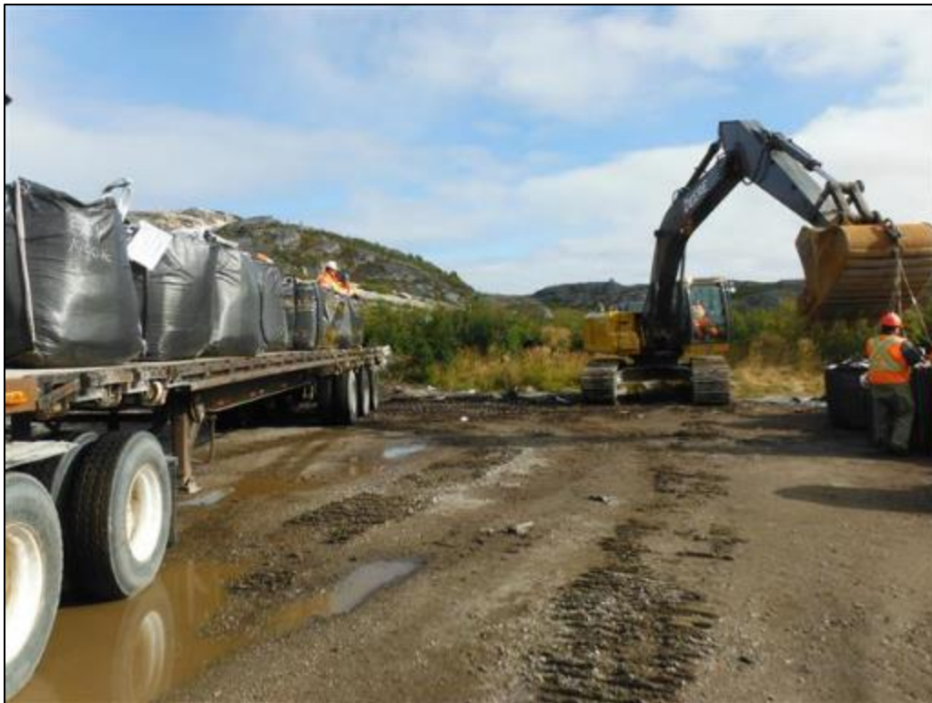
Photo 60 Pit No. 1, transferring the impacted soil bags to a flat bed truck for transport to the dock, September 16, 2015.
