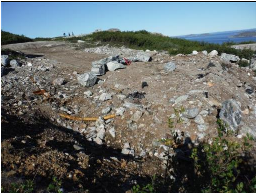
Photo 12 Main Base-Area 1 prior to soil removal in Year 5, August 18, 2015.
