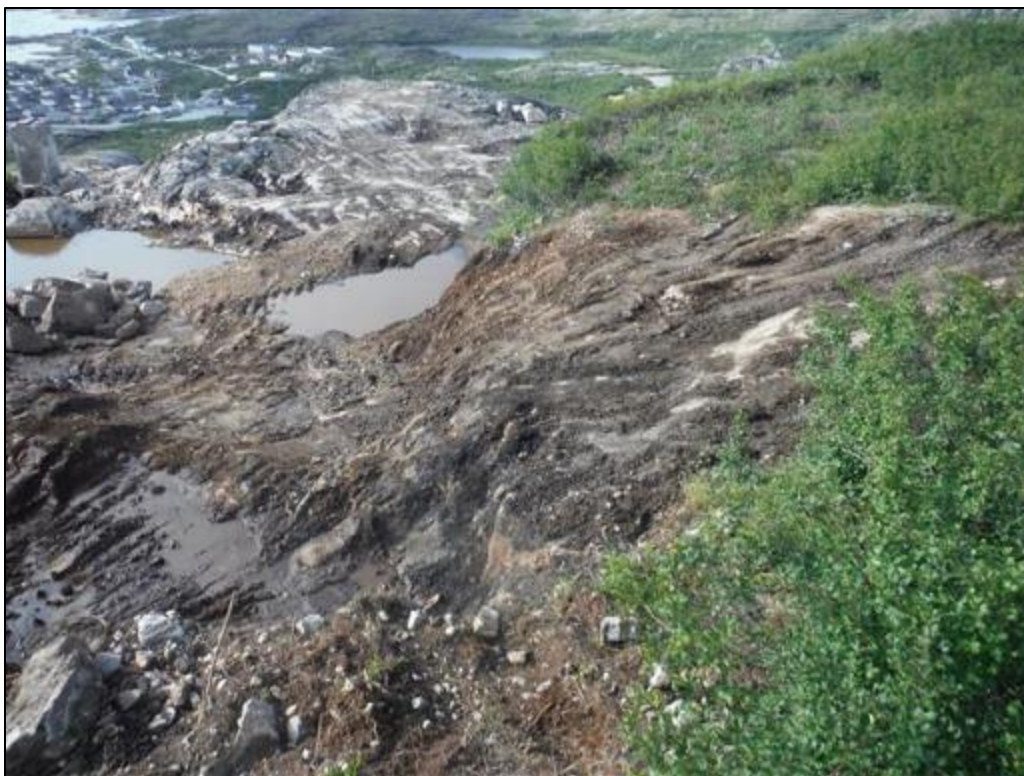
Photo 17 Soil removal at Main Base-Area 1, looking south, August 24, 2015.
