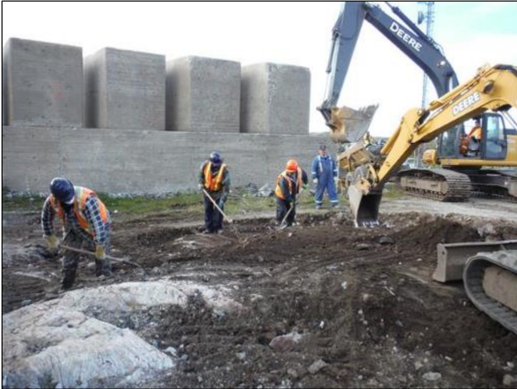
Photo 7 Soil removal at BMEWS-Area 4, August 19, 2015.
