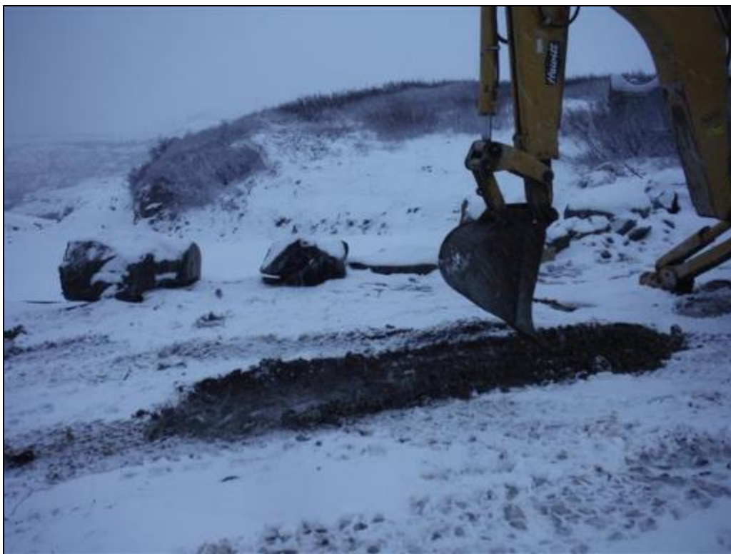
Photo 31 Additional delineation at Main Base-Area 1, October 30, 2015
