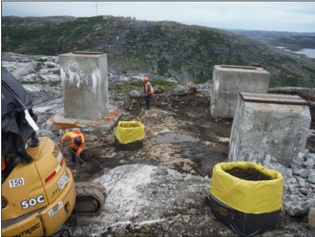
Photo 21 Soil removal at Main Base-Area 1, looking west, August 24, 2015.
