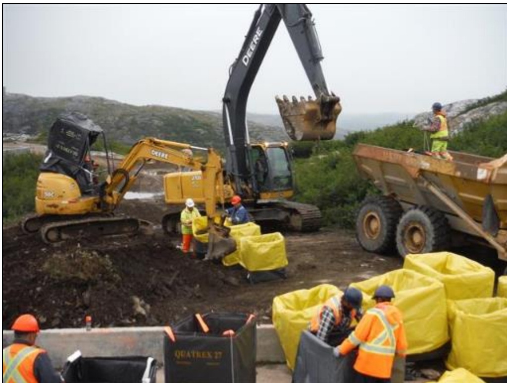
Photo 26 Bagging of removed soil at Main Base-Area 2, August 26, 2015.
