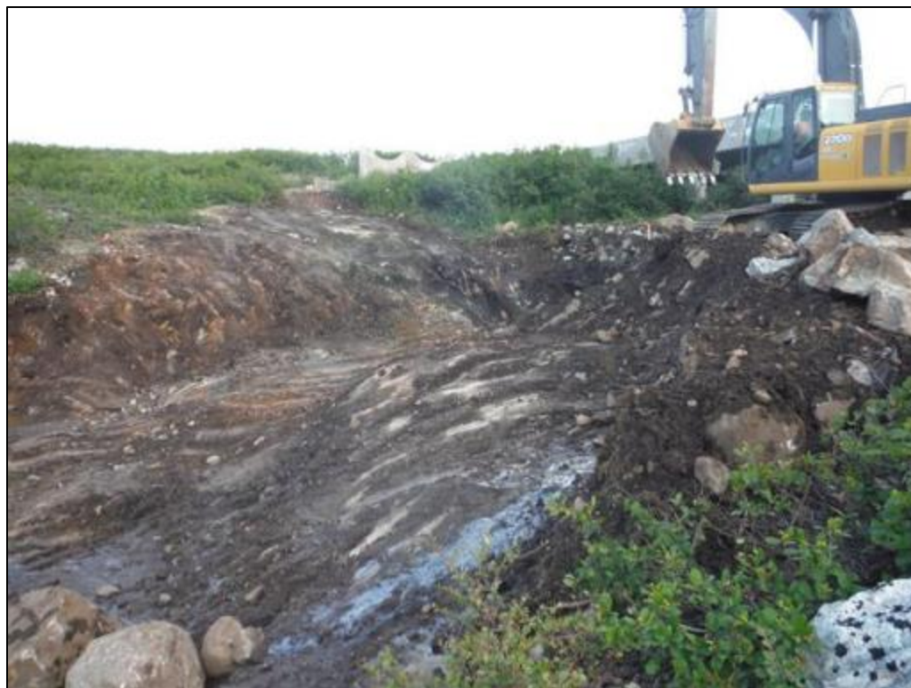
Photo 15 Soil removal at Main Base-Area 1, looking west, August 24, 2015.
