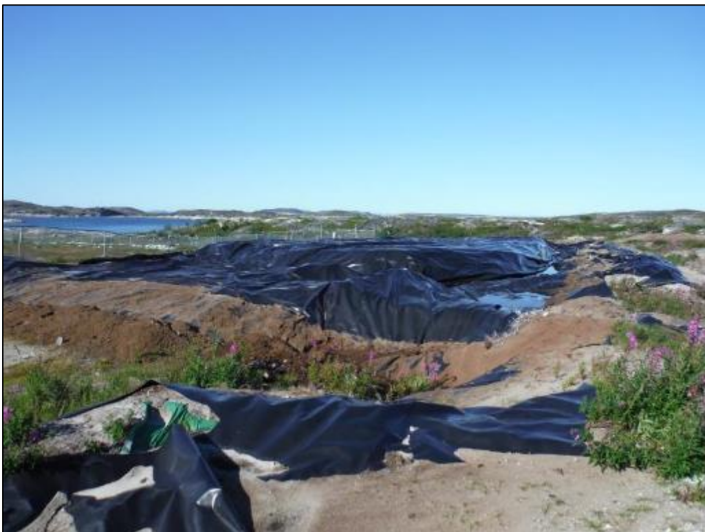
Photo 2 Biopile in Year 5 prior to soil sampling, August 18, 2015.
