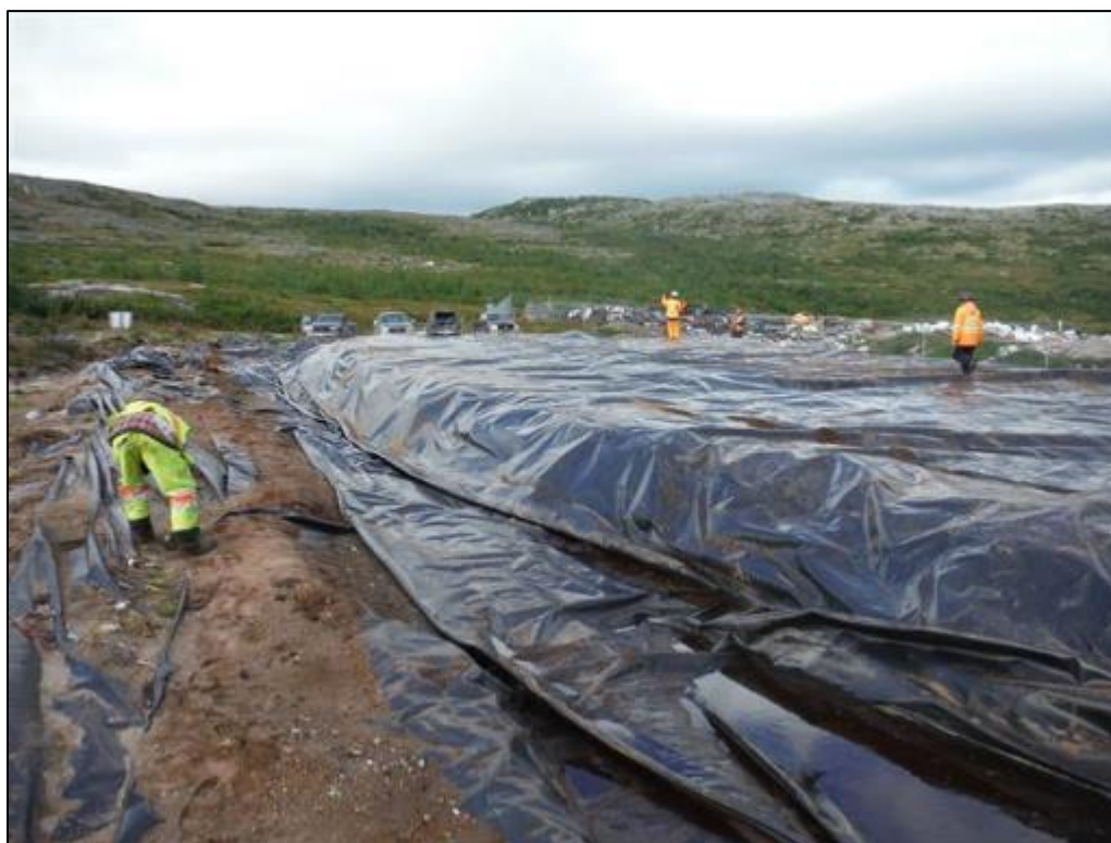
Photo 6 Securing the cover on the biopile, August 29, 2015.
