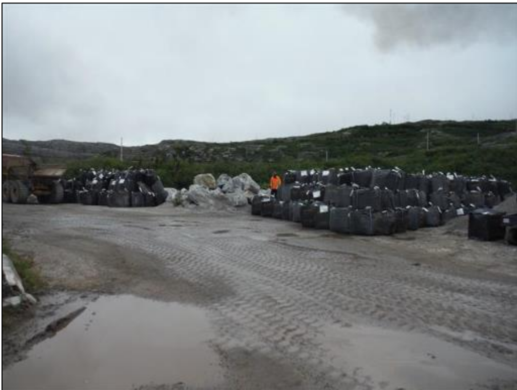
Photo 47 Pit No. 1, Staging Area for the storage of impacted soil bags, August 23, 2015.
