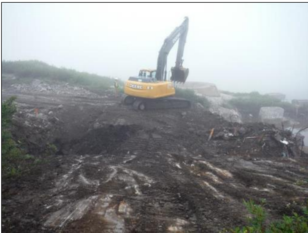
Photo13 Soil removal at Main Base-Area 1, looking east, August 21, 2015.
