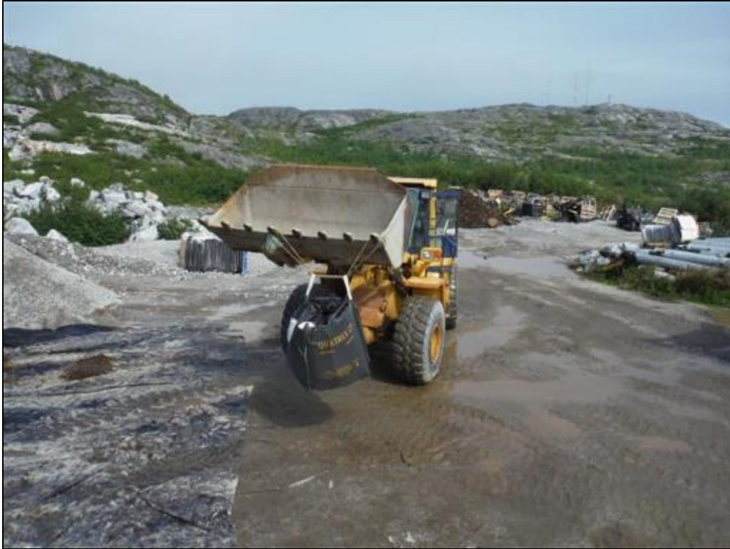
Photo 44 Pit No. 1, transporting filled soil bag at Staging Area, August 21, 2015.
