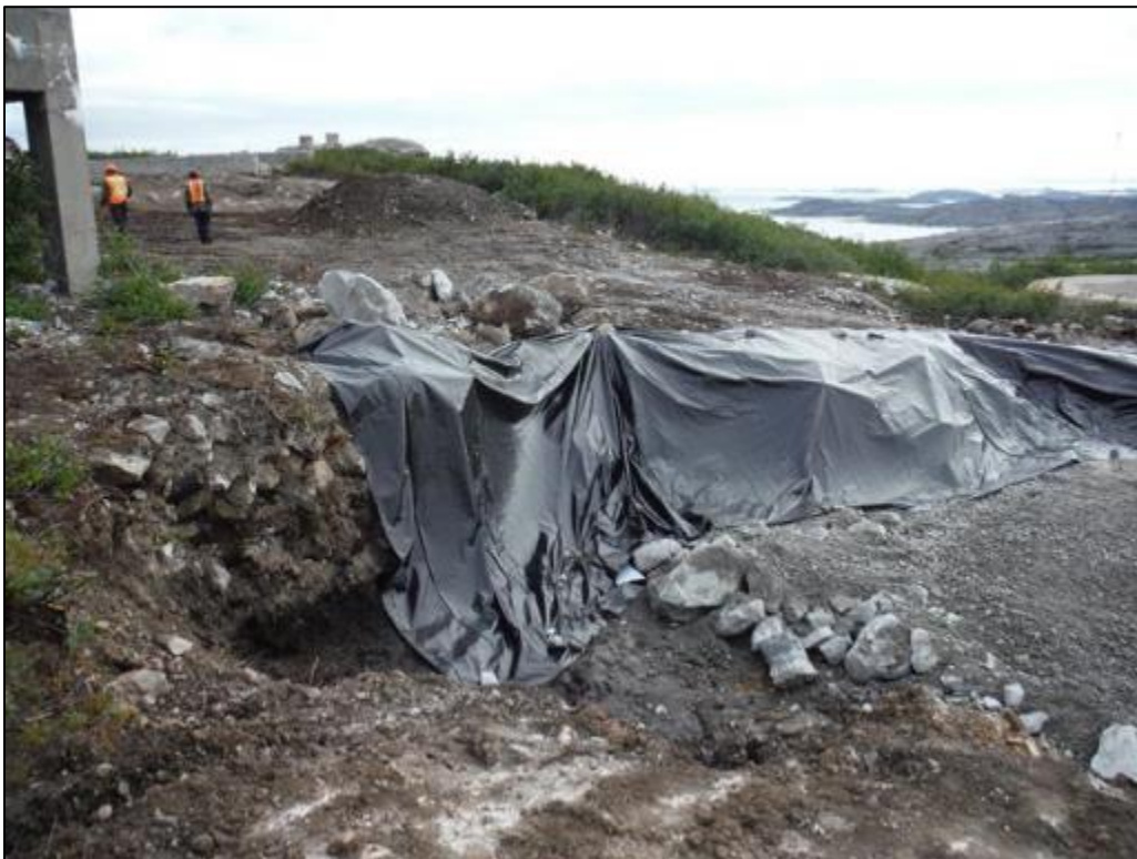
Photo 28 Remedial excavation backfilled at Main Base-Area 1 and remedial excavation boundary covered, September 1, 2015 .
