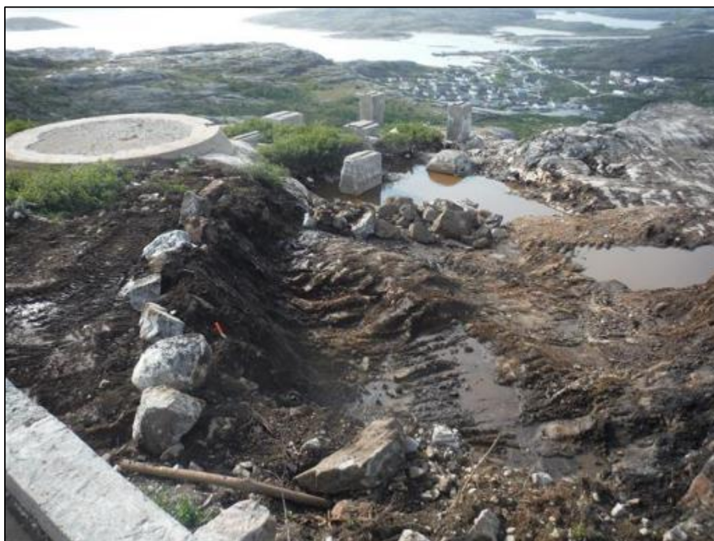
Photo 16 Soil removal at Main Base-Area 1, looking southeast, August 24, 2015.
