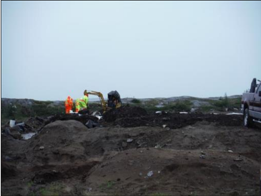
Photo 3 Application of amendments to the biopile, August 20, 2015.
