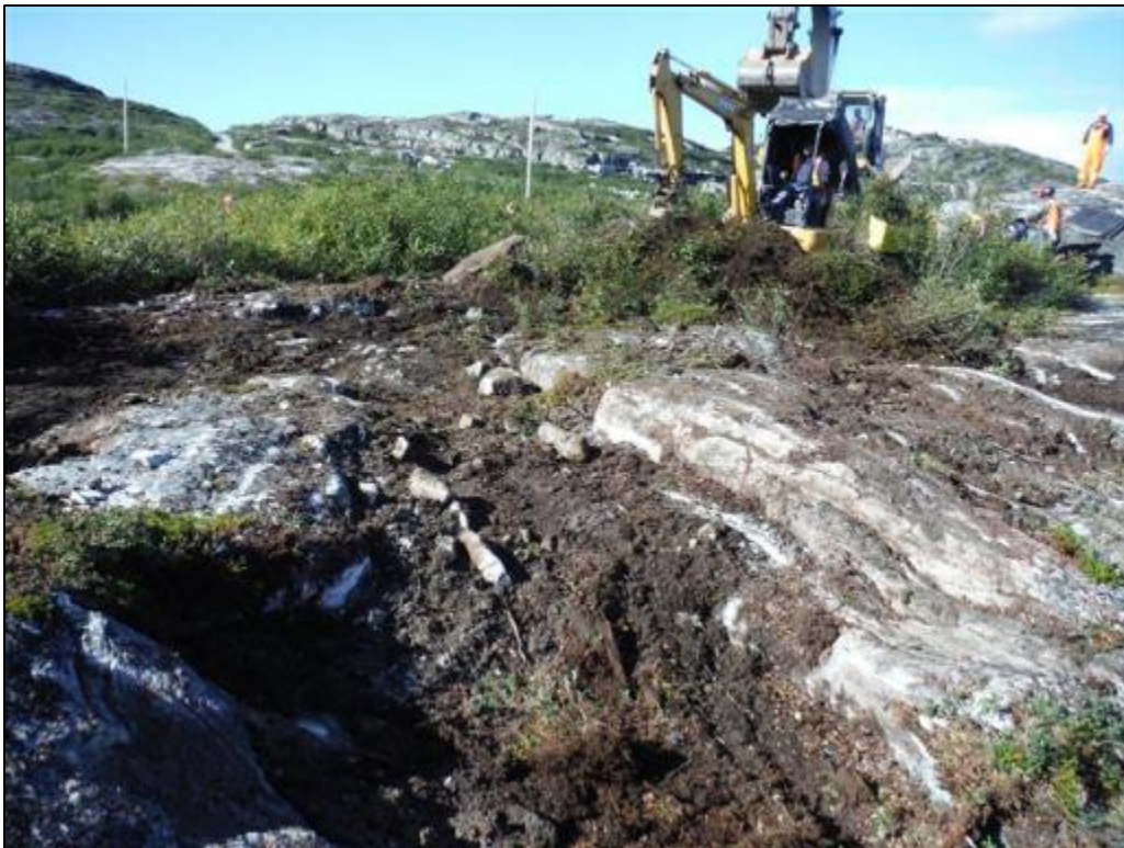
Photo 35 Soil removal at POL-Area 4, looking north, August 30, 2015.
