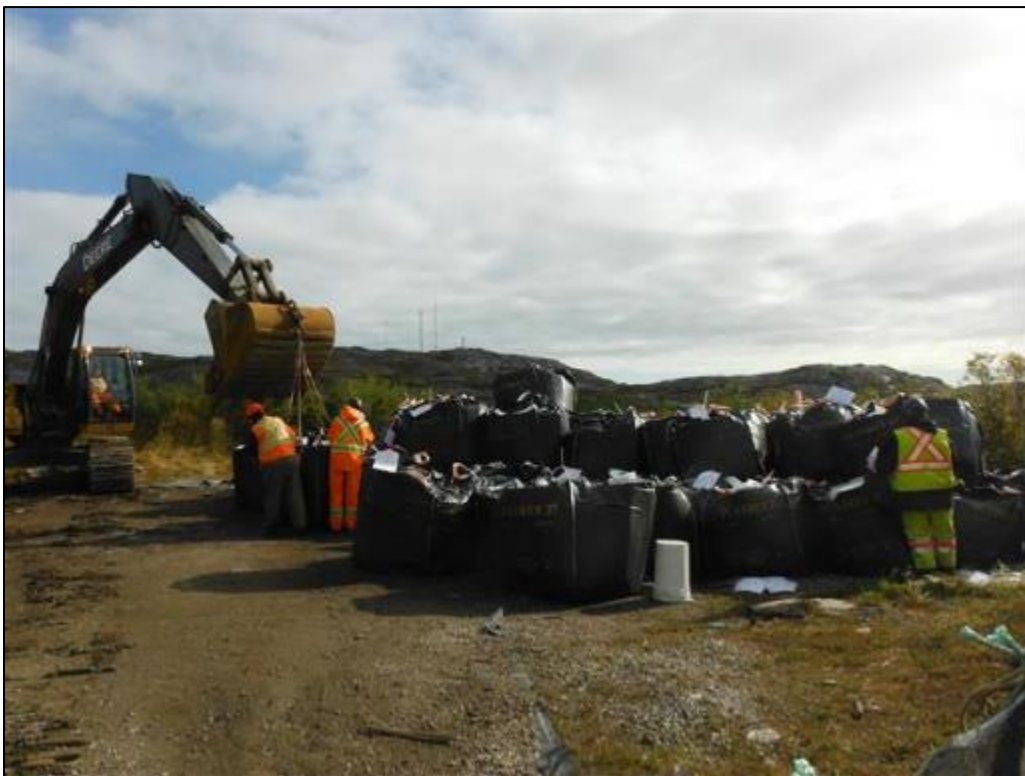
Photo 59 Pit No. 1, transferring the impacted soil bags for transport to the dock, September 16, 2015.
