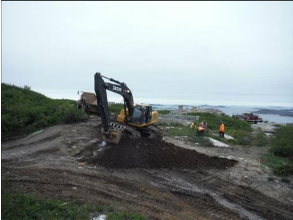
Photo 23 Soil removal at Main Base-Area 2, looking east, August 25, 2015.
