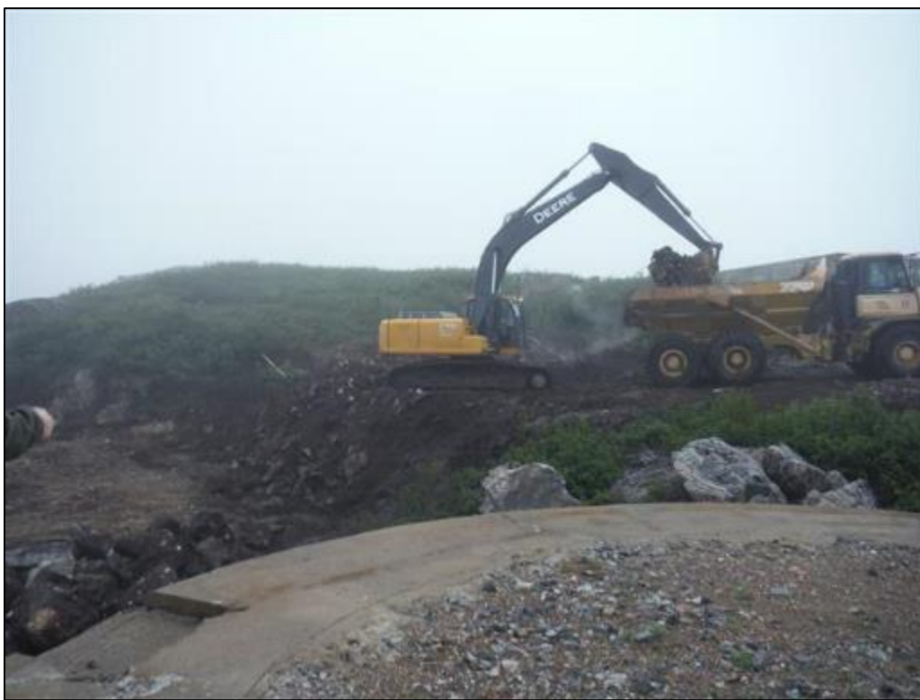
Photo 14 Soil removal at Main Base-Area 1, looking west, August 21, 2015.
