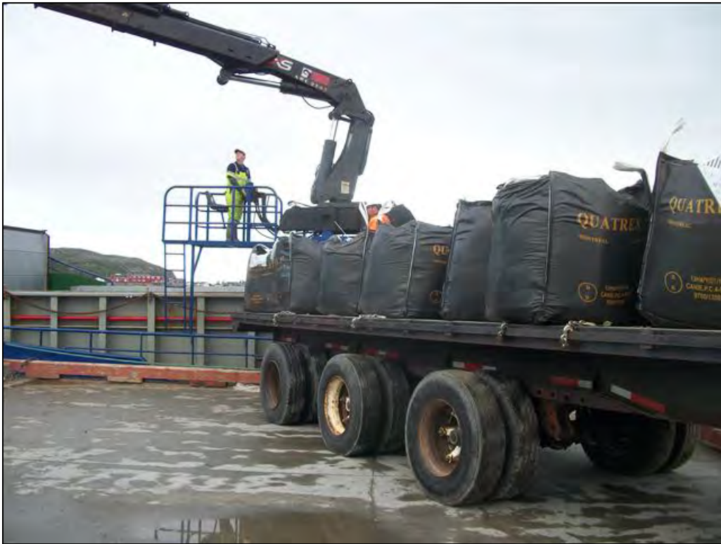
Photo 41 Loading of impacted soil bags from a flat bed truck, July 30, 2016.
