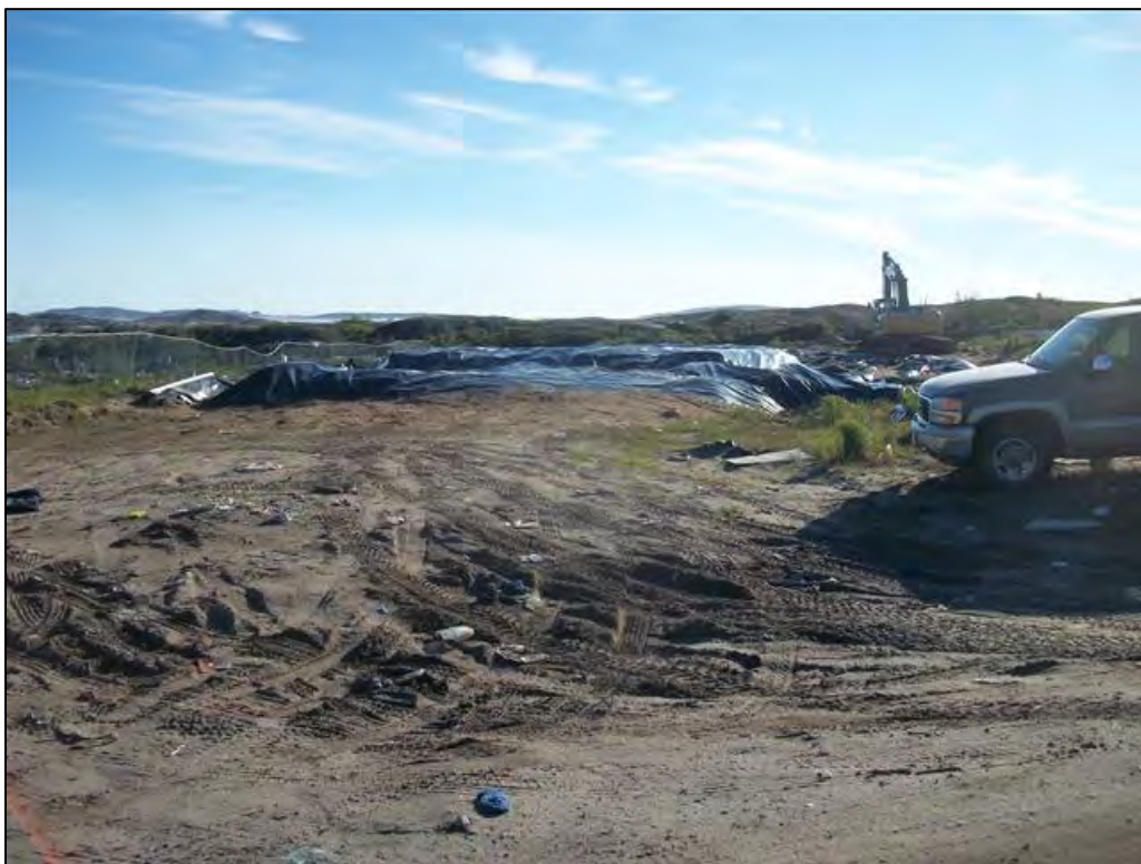
Photo 1 Biopile in Year 6 prior to soil sampling, July 7, 2016.
