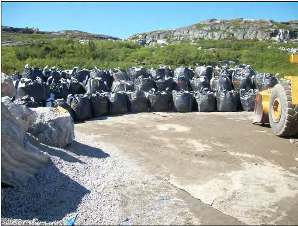
Photo 34 Stockpiled bags of impacted soil at Pit No. 1, July 11, 2016.
