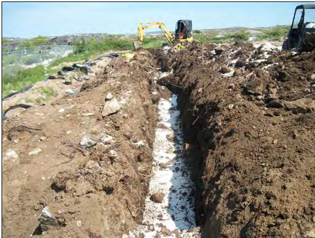
Photo 5 Application of amendments to the nutrients, July 17, 2016.
