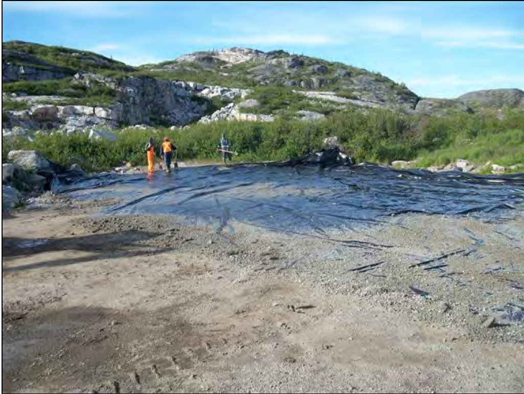
Photo 35 Pit No. 1, installing liner at staging area, July 11, 2016.
