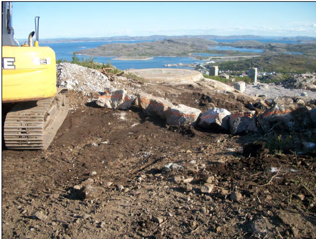
Photo 20 After soil removal at Main Base-Area 1 Northeast and remedial excavation boundary blocked by boulders, July 21, 2016.
