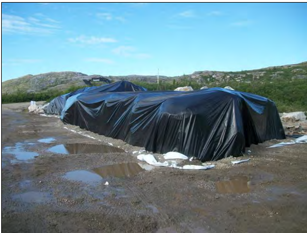
Photo 39 Storage of soil bags containing PCB-impacted soil for second shipment at Pit No. 1, August 3, 2016.
