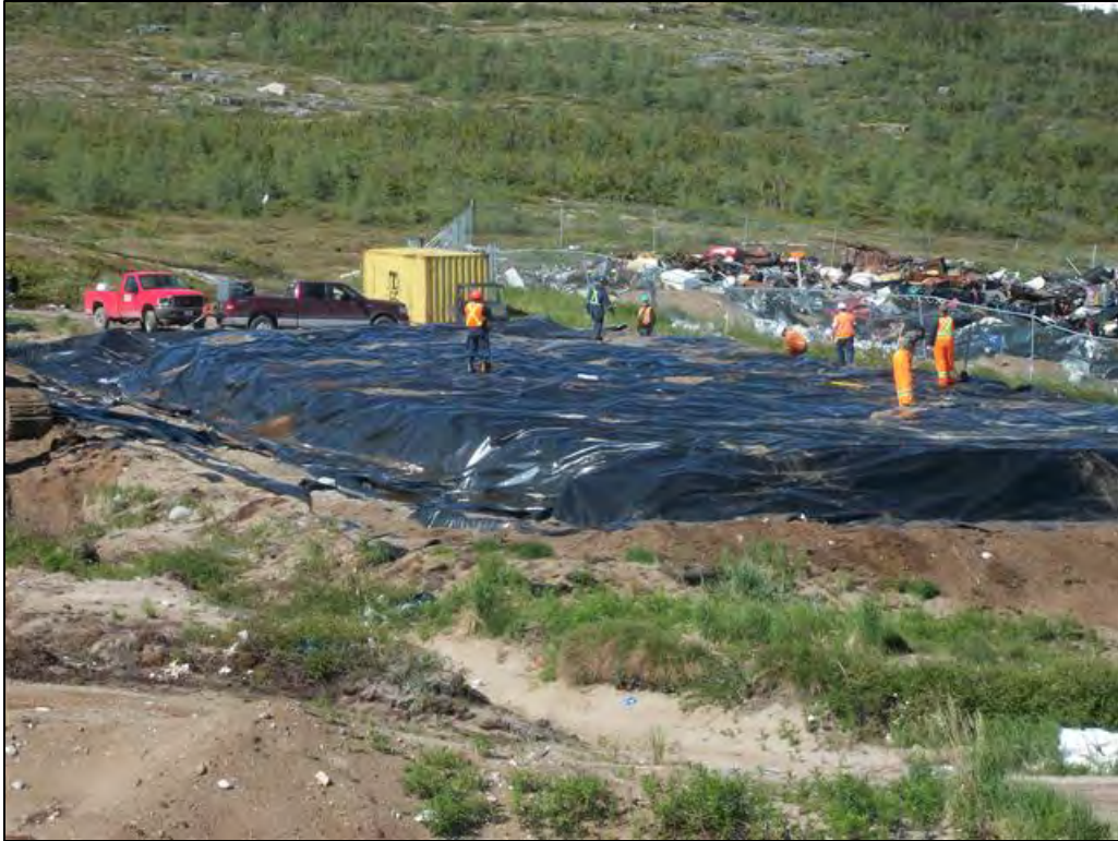
Photo 3 Biopile in Year 6 prior to soil sampling, July 7, 2016.
