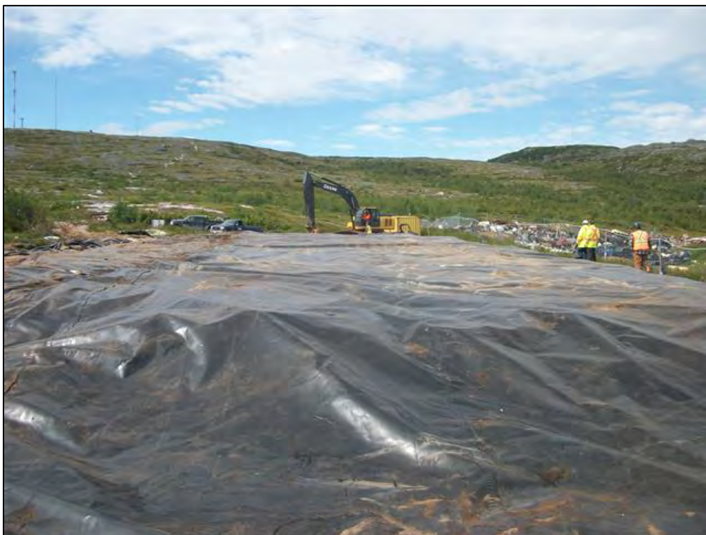
Photo 6 Securing the cover on the biopile, August 2, 2016.
