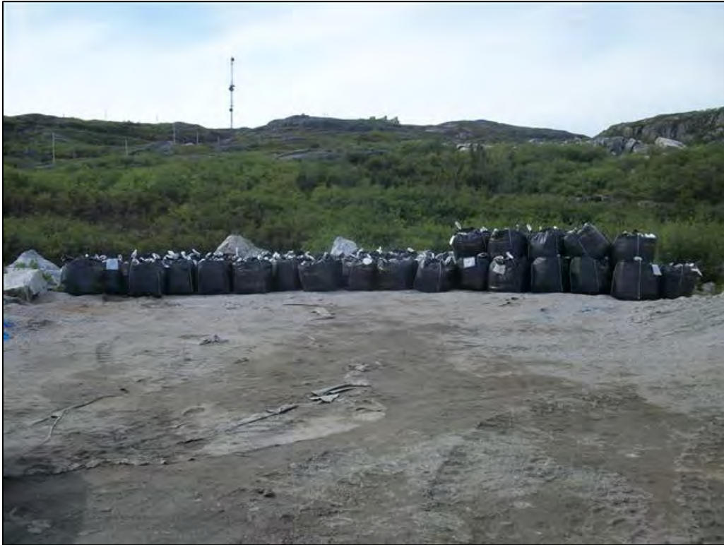
Photo 33 Stockpiled bags of impacted soil at Pit No. 1, July 8, 2016.
