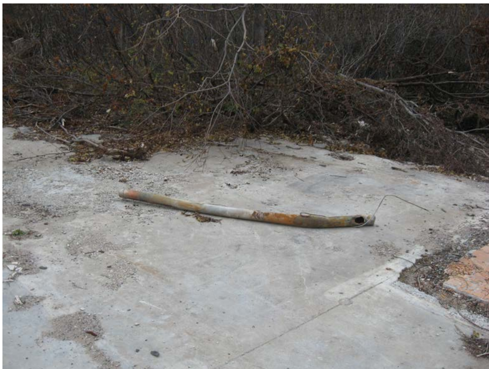
Photo 2 View of concrete building pad and surface debris (09-SD29) at the site
