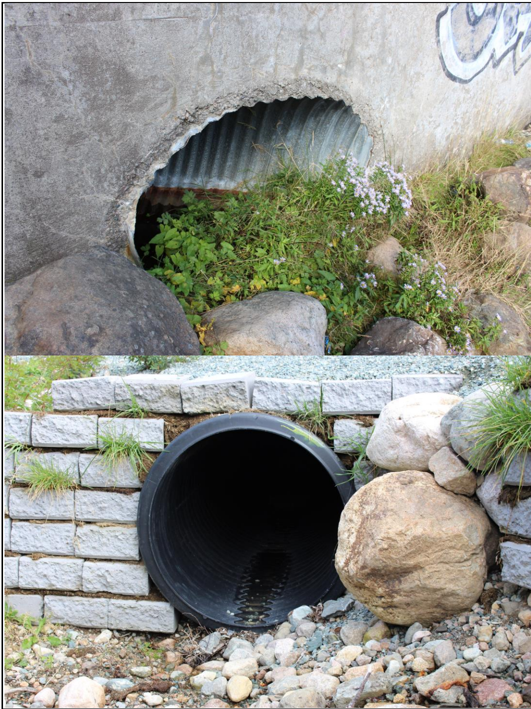
Figure 5.1 A Corrugated Steel Culvert Mitred to the Face of a Wall (Top), and a Small Plastic Culvert with a Masonry Headwall (Bottom)
