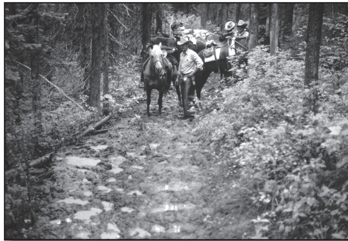
Figure 9—Standing water results in soft, boggy tread.
