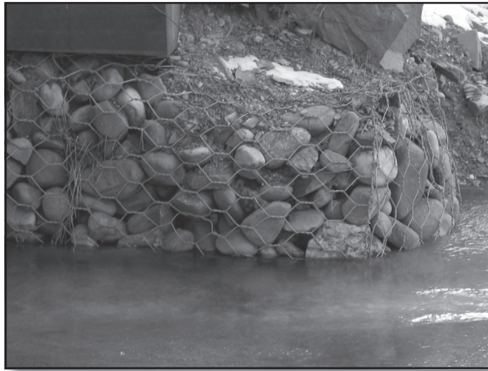
Figure 78—Wire baskets, often called gabions, are another retaining structure.
