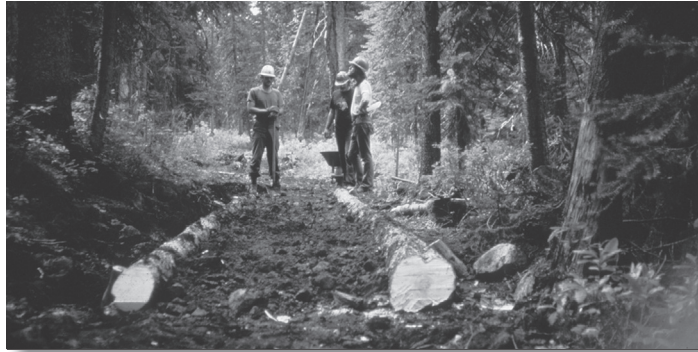
Figure 54—Subsurface puncheon covered with soil and rock.
