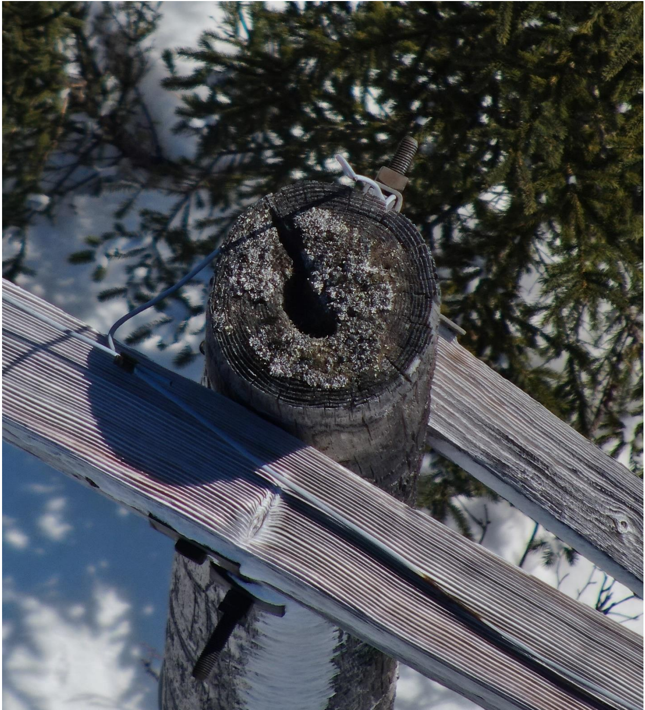
Figure A-1 – Void in Pole Top, Hollow Pole
