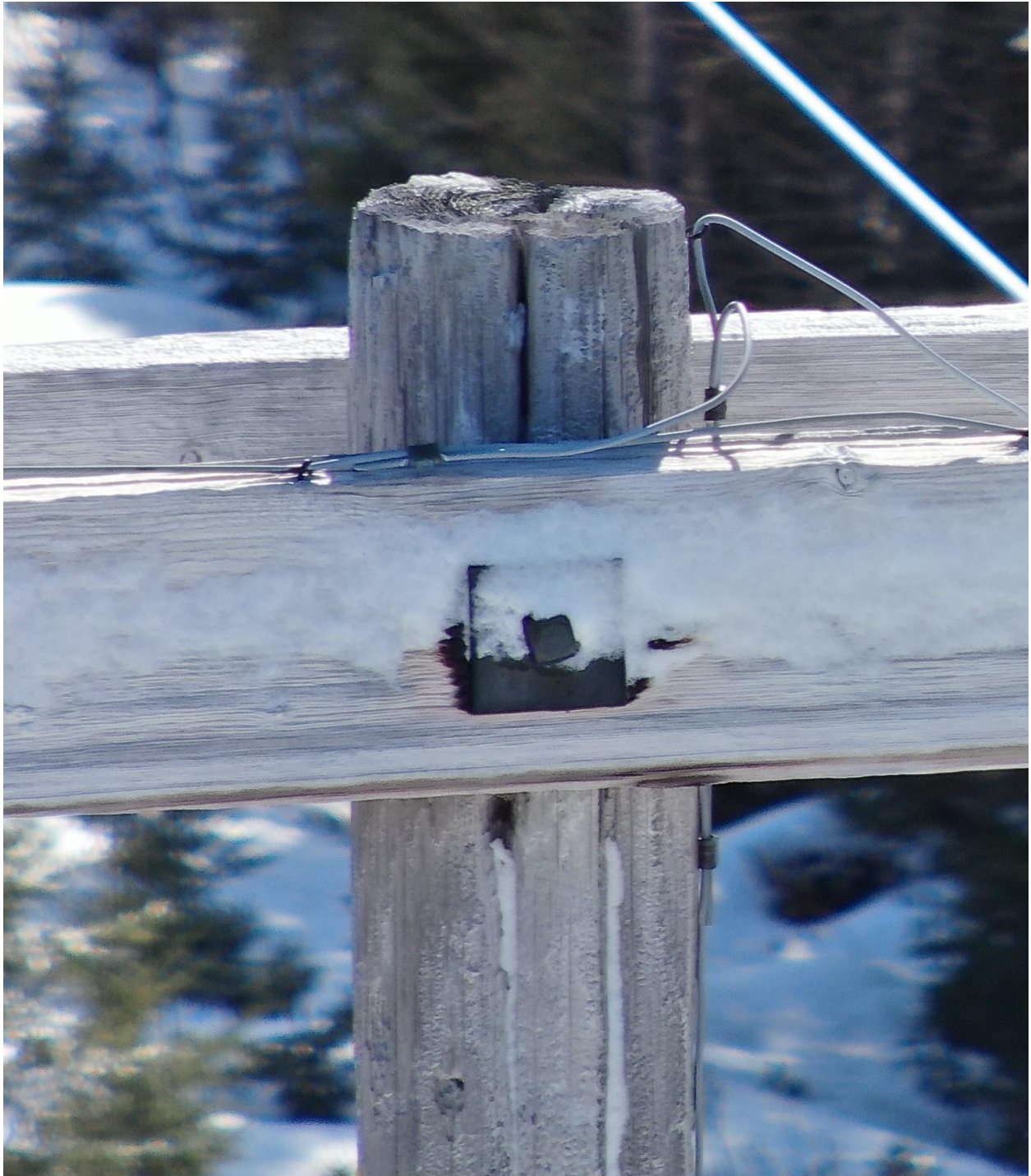
Figure A-3 – Severe Splits in Pole through Cross Arm Bolt Locations
