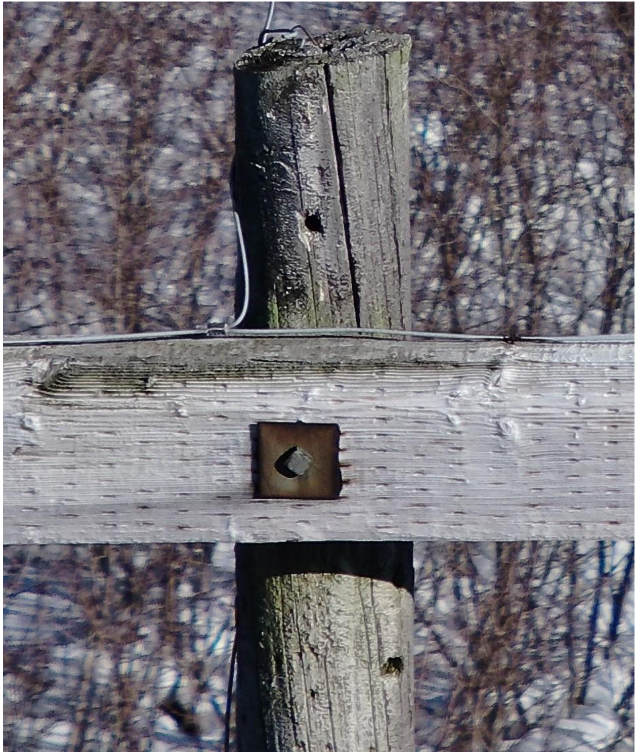
Figure A-6 – Split through Pole Top, Woodpecker Holes
