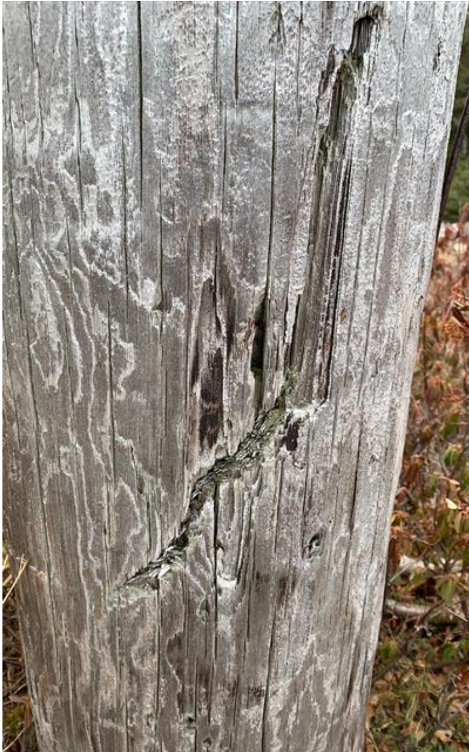
Figure A-13 – Pole Damage and Horizontal Crack
