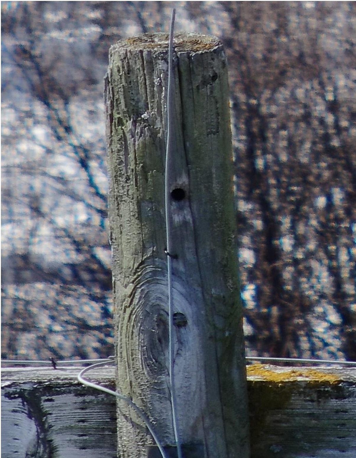
Figure A-7 – Pole Top Damage, Splits, Woodpecker Holes
