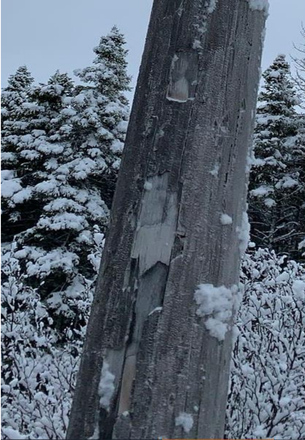
Figure A-14 - Shell Separation, Pole Damage
