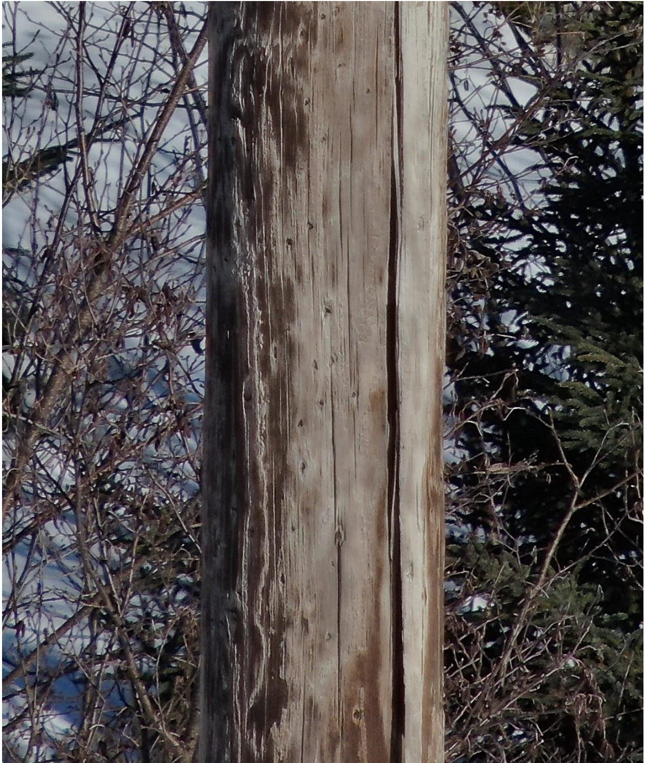
Figure A-5 – Large Split in Pole, Hollow
