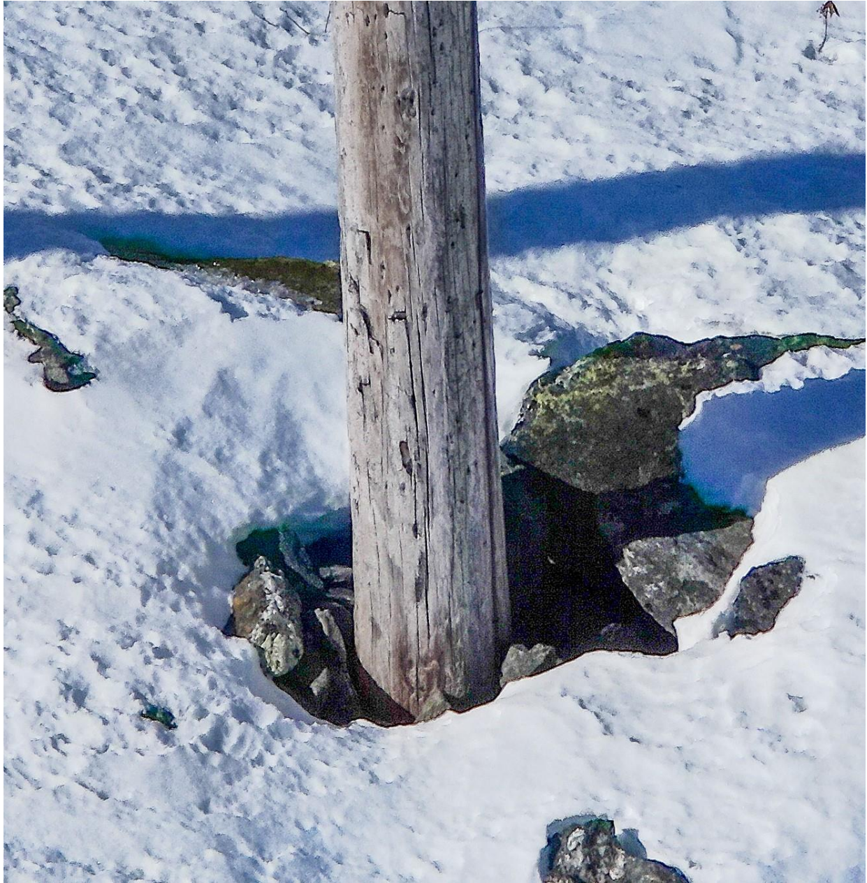
Figure A-10 – Shell Separation and Missing Crib
