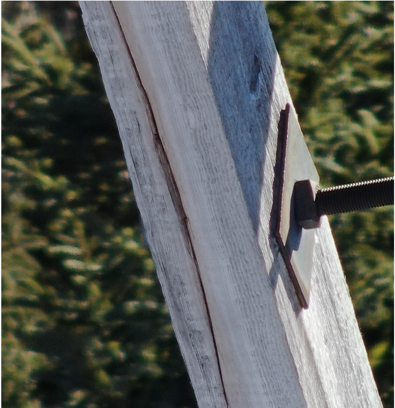
Figure A-4 – Large Crack through Cross Brace
