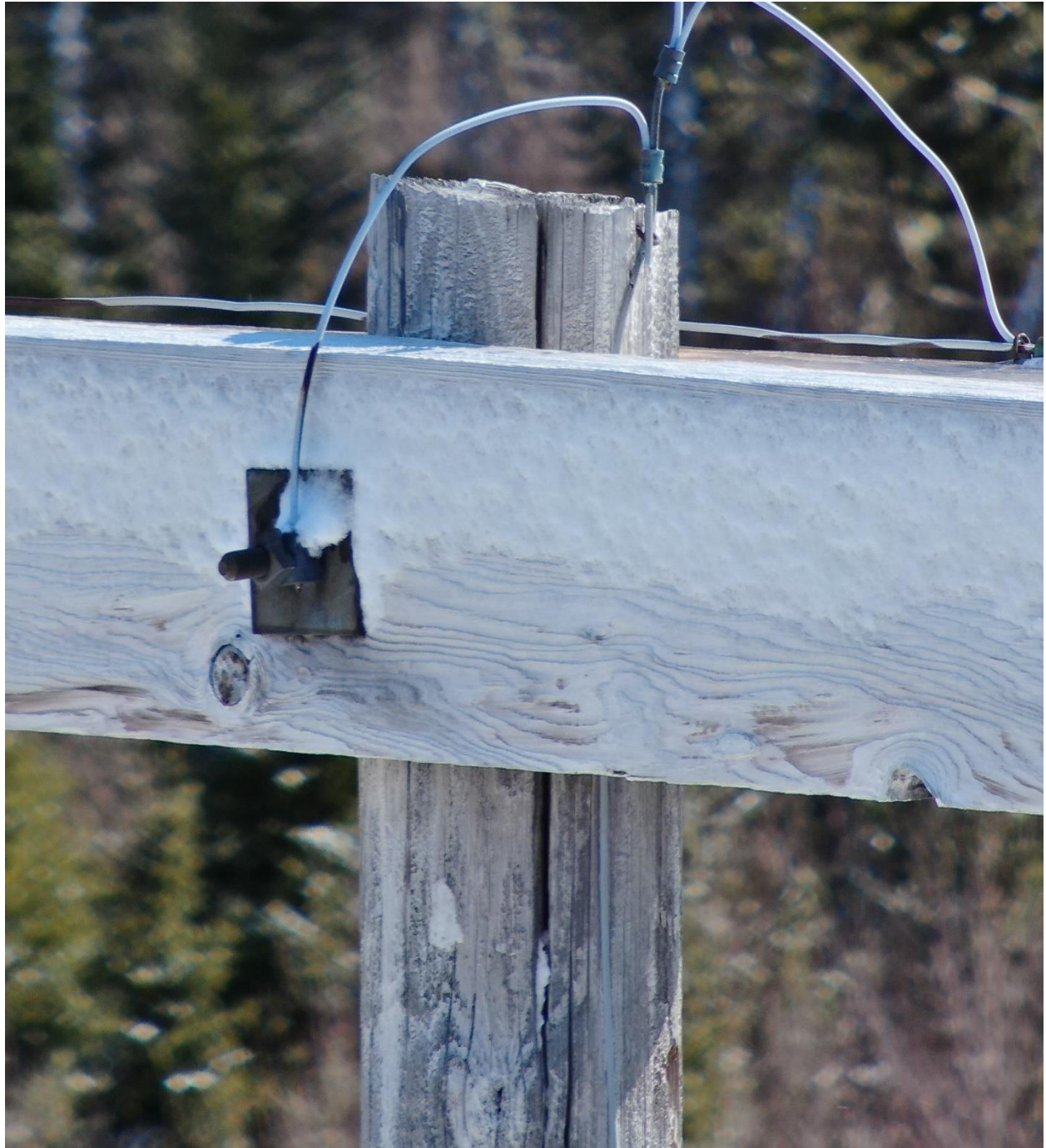
Figure A-2 – Deep Splits in Pole
