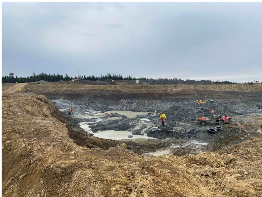
Picture 10: Labourers washing down bedrock in preparation for aerial survey and detailed geological mapping
