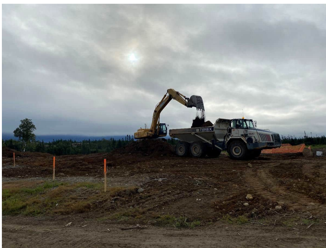
Picture 7: Excavator operator loading articulated rock truck with trench overburden
