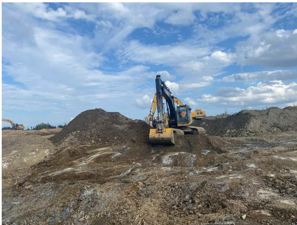
Picture 9: Heavy Equipment Operator scraping bedrock using excavator-mounted cleaning bucket
