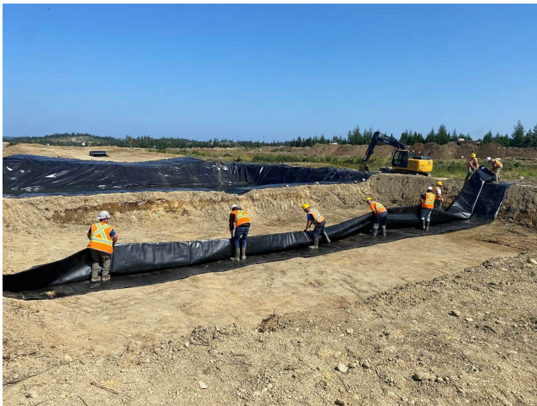
Picture 8: Labourers installing PVC liner at the Keats Trench settling pond
