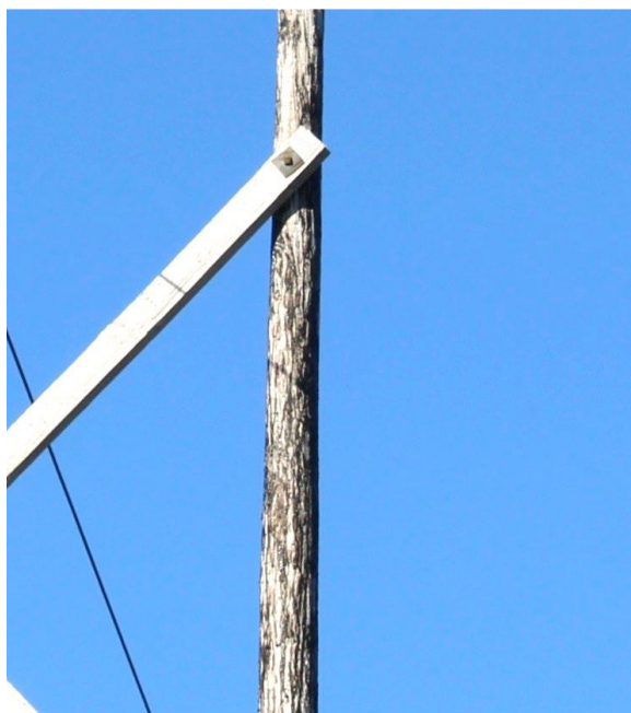
Figure A-2: Deteriorated Pole – Shell Separation
