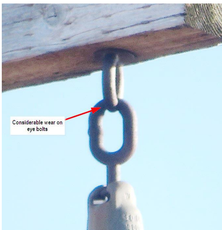
Figure A-6: Worn Ball Link Eye Bolt
