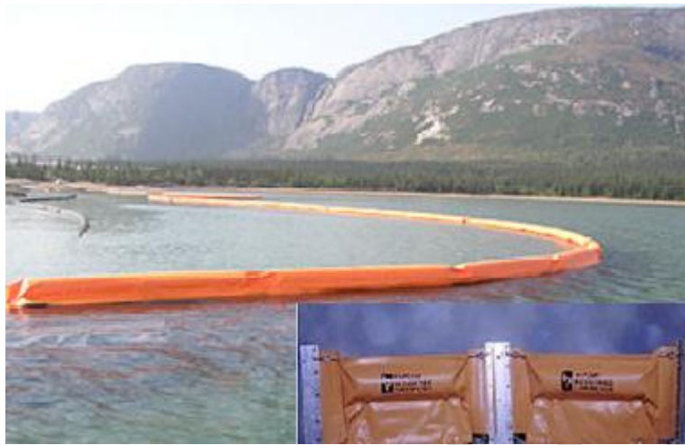
Figure 1. Containment boom for containing any drifting debris resulting from removal activities.
