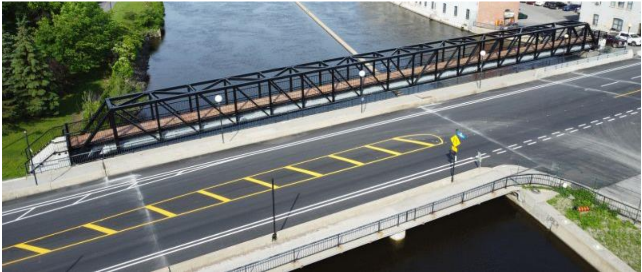
Figure 4.9. Example of bridge that could be deployed on the Demonstration Trail (e.g., at Portland Creek). Note: All bridges will be clear span bridges (i.e., no pilings/abutments in the water).
