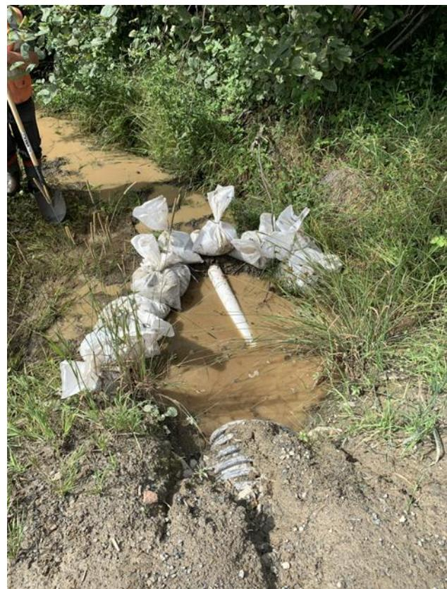
Figure 2 – Inverted Weir
