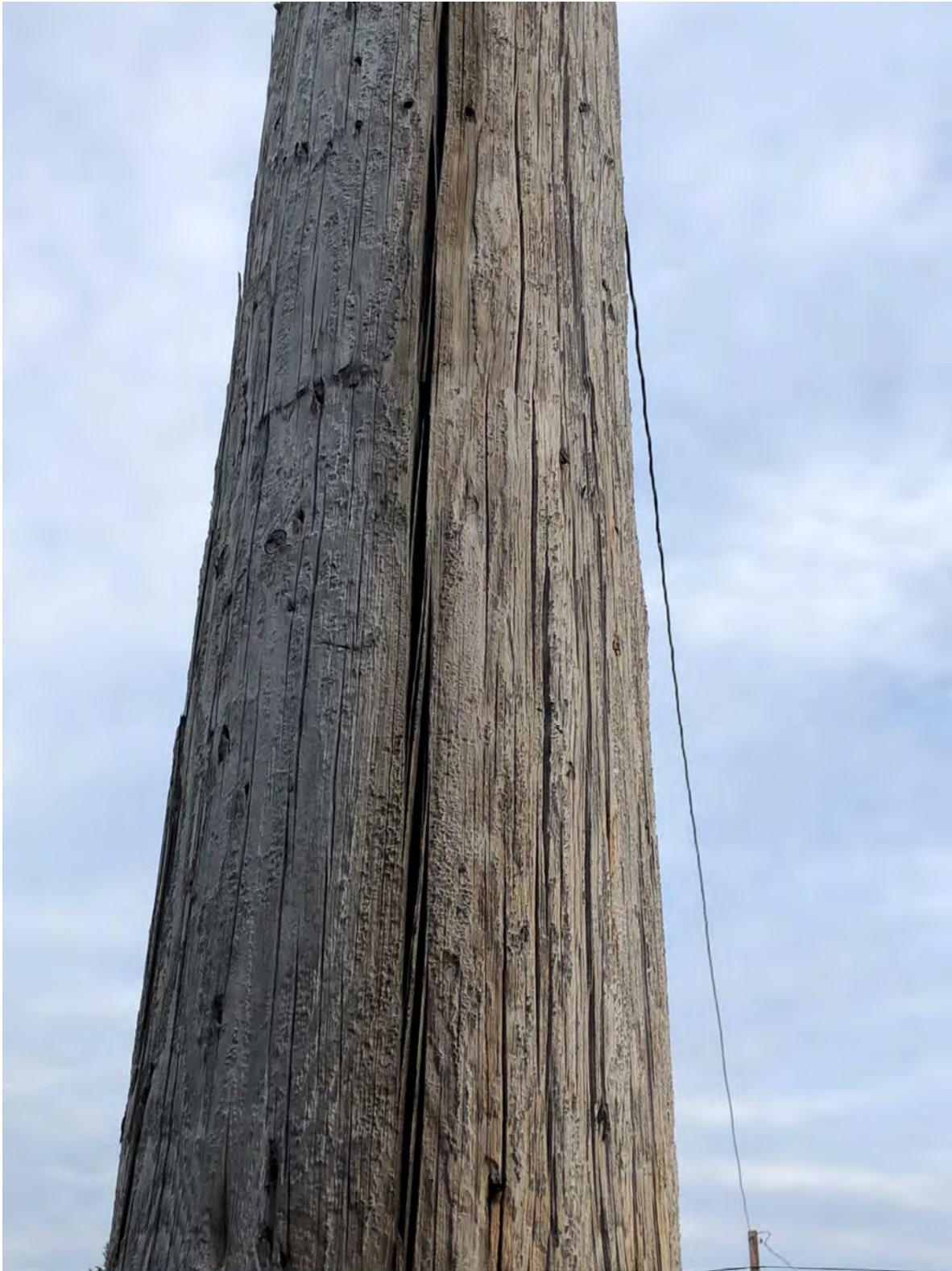
Figure A-3: Deep Splits, Hollow Pole
