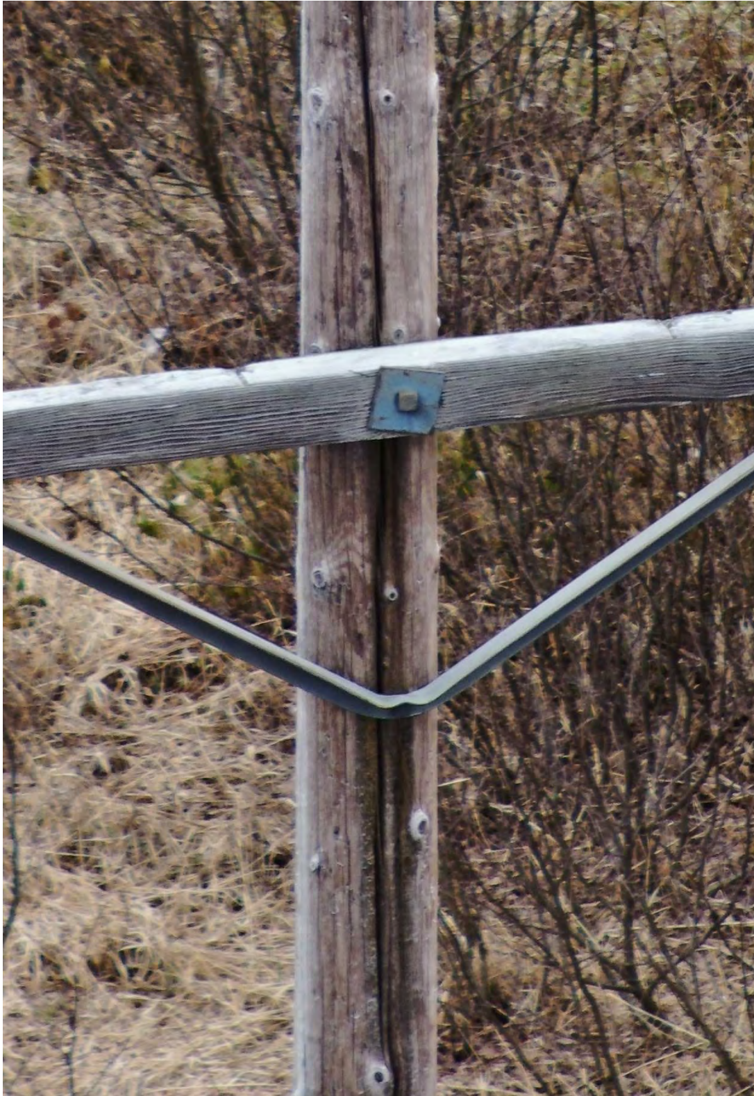
Figure A-4: Large Split Through Cross-arm Hardware
