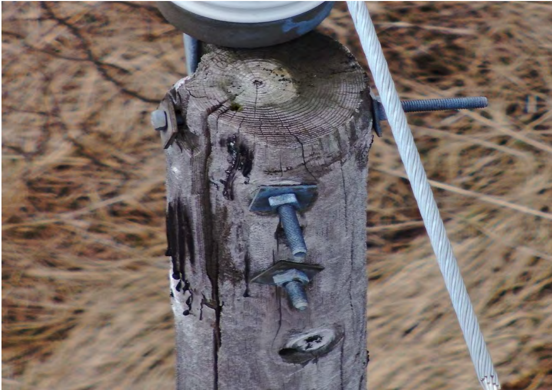
Figure A-8: Deteriorated and Narrowed Pole Top
