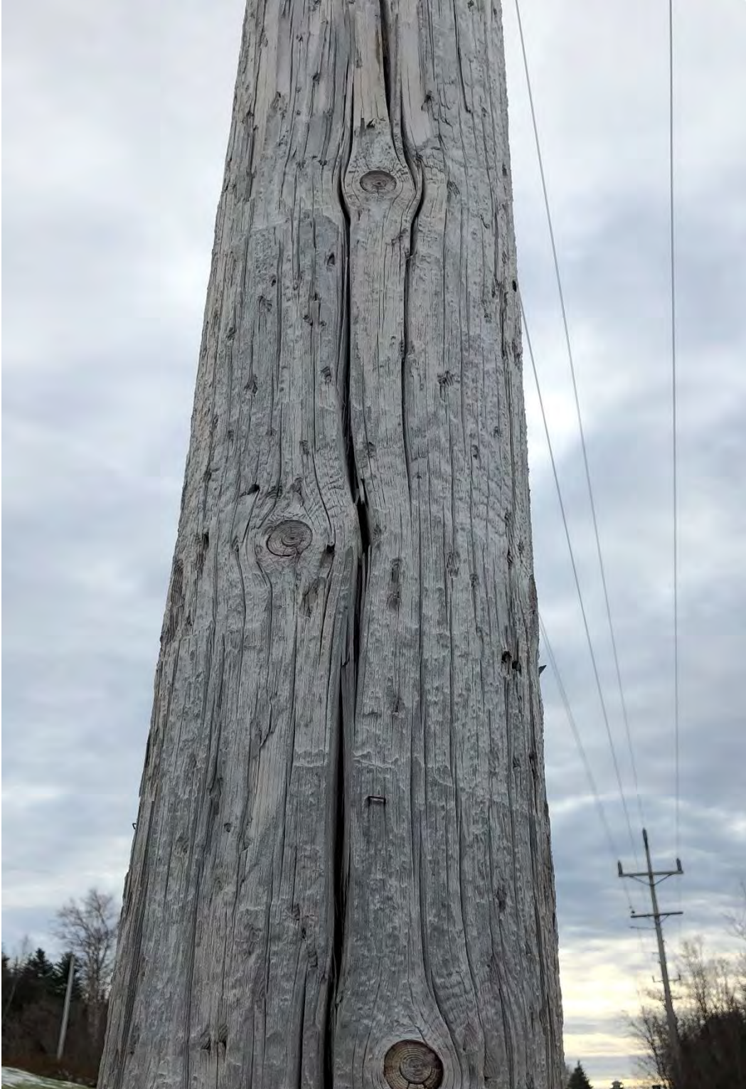
Figure A-1: Deep Splits Through Hollow Pole
