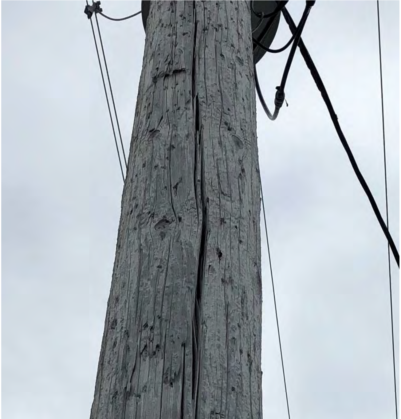
Figure A-2: Hollow Pole, Large Splits
