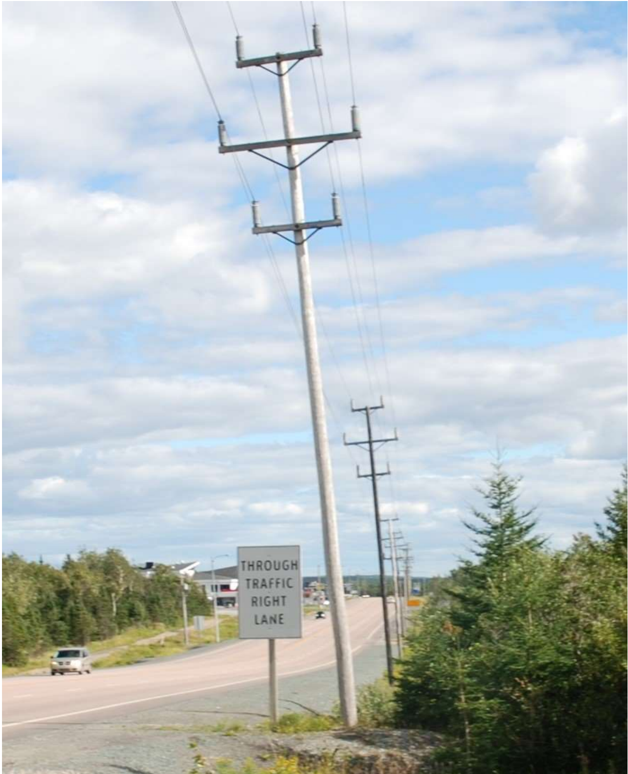
Figure A-10: Leaning Structure (Double Circuit Structure)
