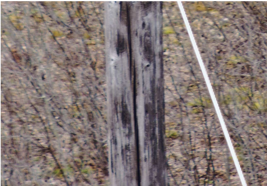
Figure A-7: Deep Splits Through Pole
