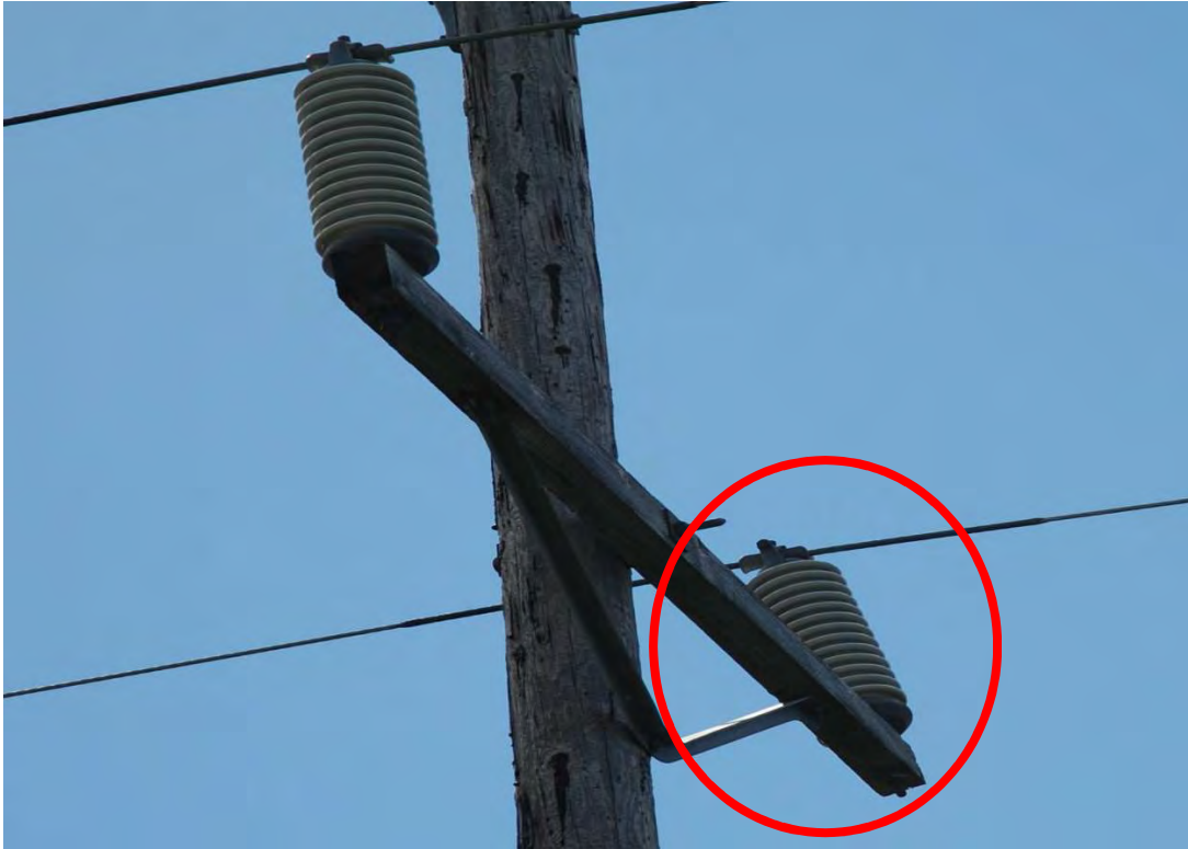
Figure A-11: Twisted Cross Arm Supporting Insulator
