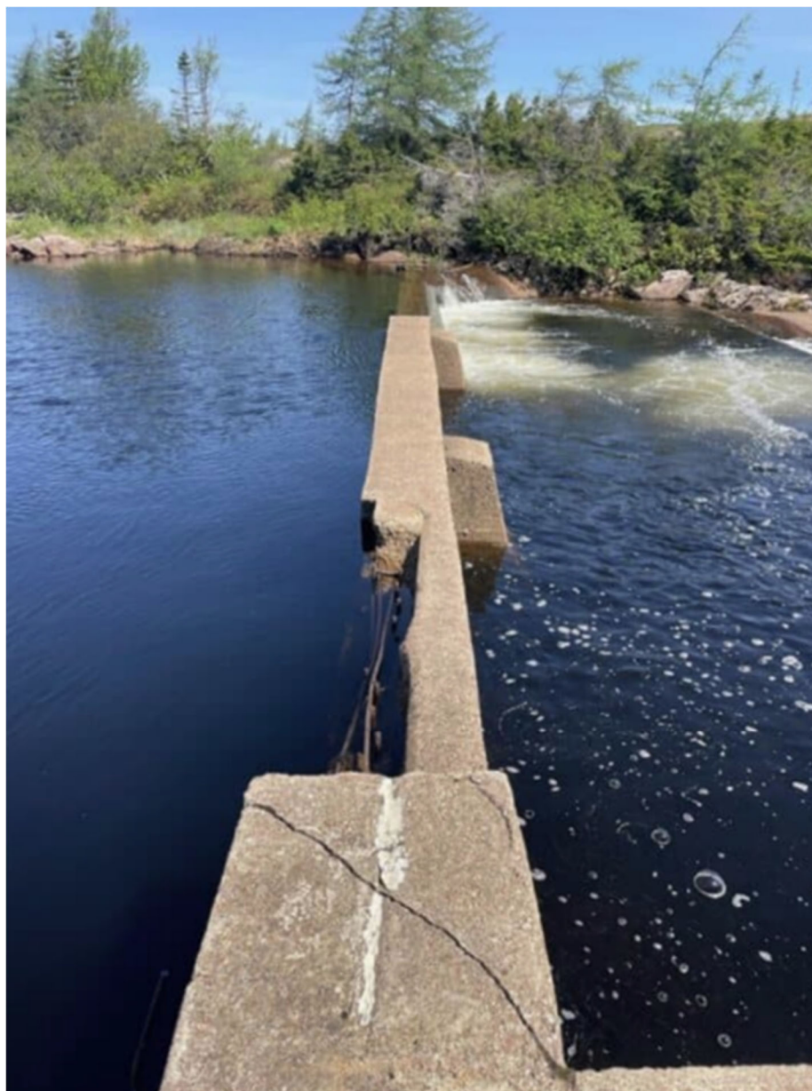
Figure 3-2 Existing Dam With 3.6 m Deteriorated Section
