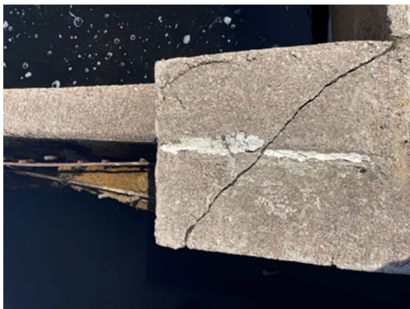
Figure 3-1 Deterioration to Existing Concrete Dam
