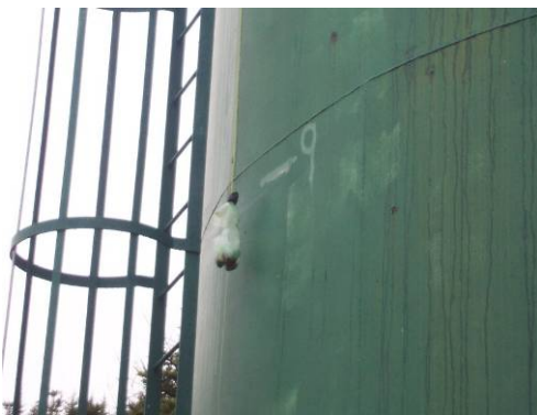
Figure 37: Water level indicator on St. Alban's tank
