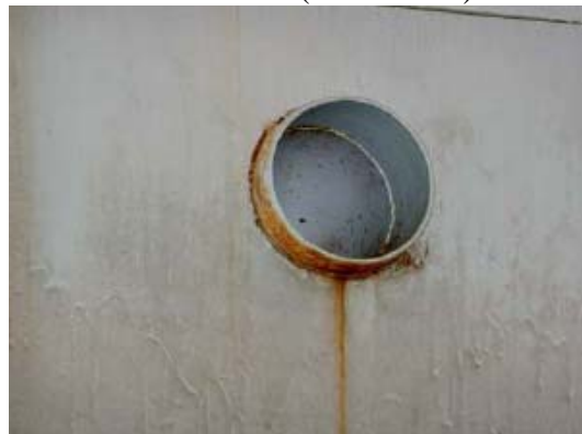
Overflow Weir Box (inside tank)
