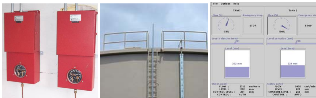
Figure 6: Radial pressure gauge (St. Alban's), gauge board and SCADA readout used to monitor water level in tank
