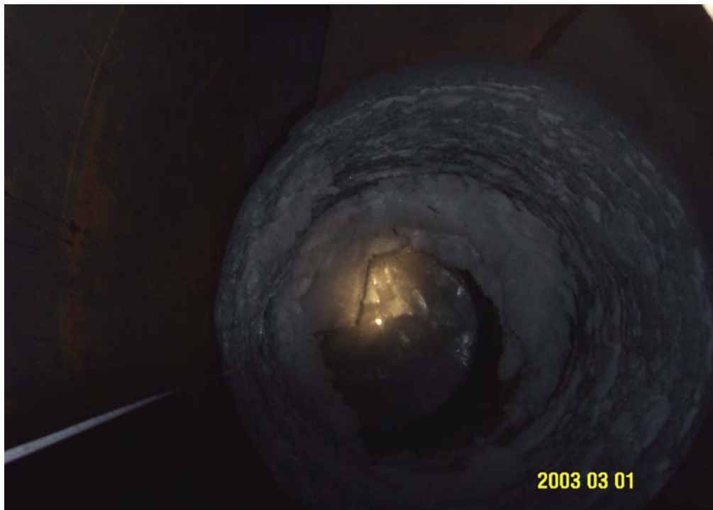
Figure 28: Ice build-up inside Badger standpipe is double in thickness on the windward side of tank
