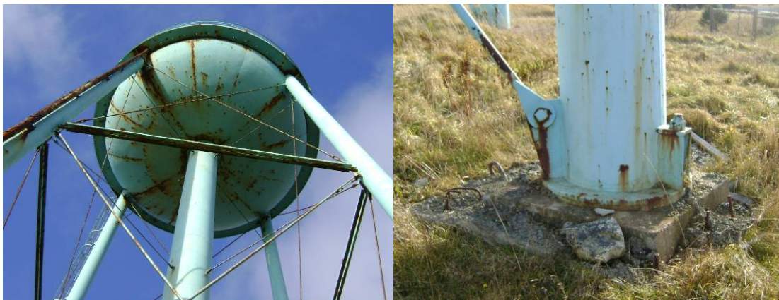
Figure 40: Condemned elevated water storage tank in Trepassey
