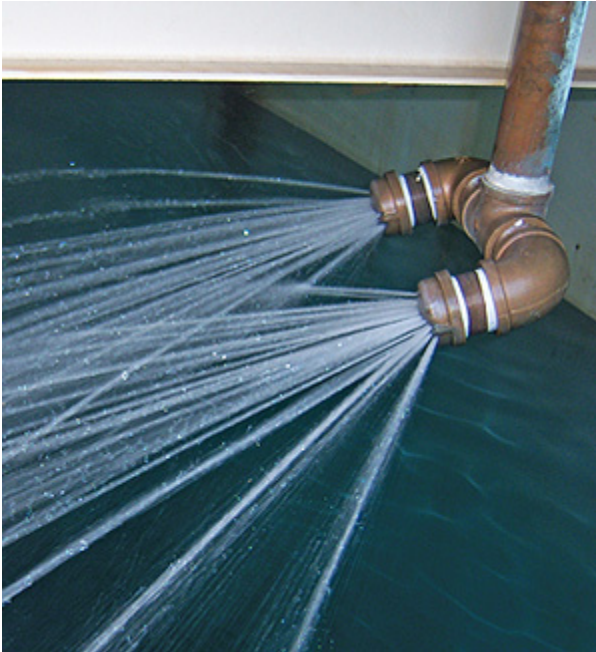
Figure 15: Spray aeration system in water storage tank (Walfoot, 2008)
