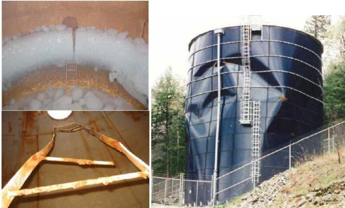
Figure 19: Examples of ice damage in a water storage tank
