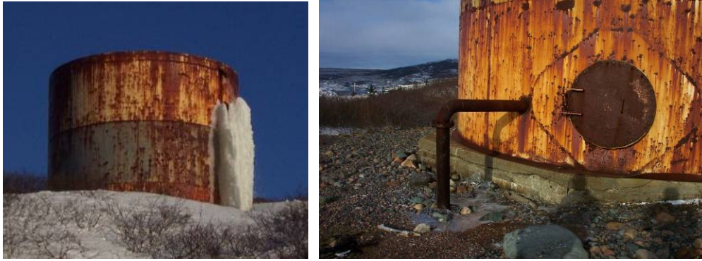
Figure 32: Frozen overflow and frozen intake pipe from Lawn water storage tank
