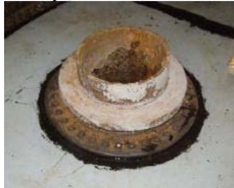
Silt Stop (inside tank)
