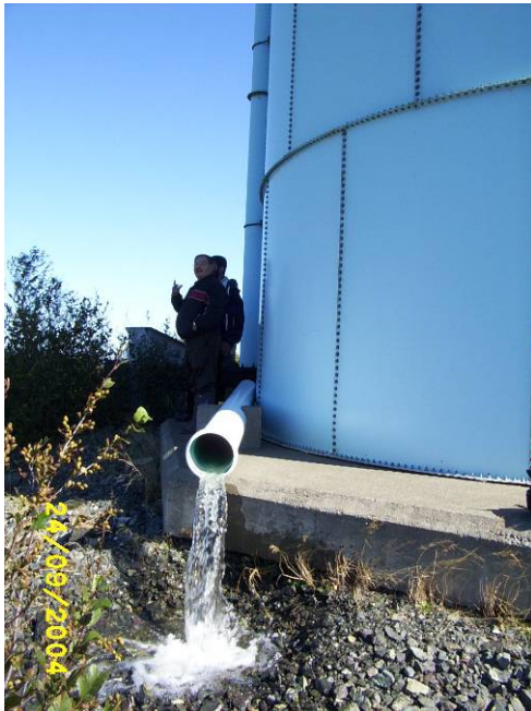
Figure 30: Brighton tank overflowing
