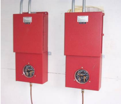
Pressure Gauges (pump switches)
