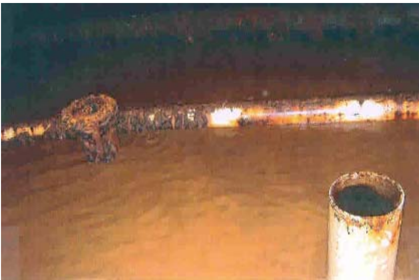
Figure 43: Interior of Woody Point tank including sediment accumulation and broken overflow pipe
