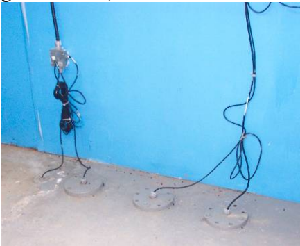
Sensor Cables- Water Level (from in-ground tank)
