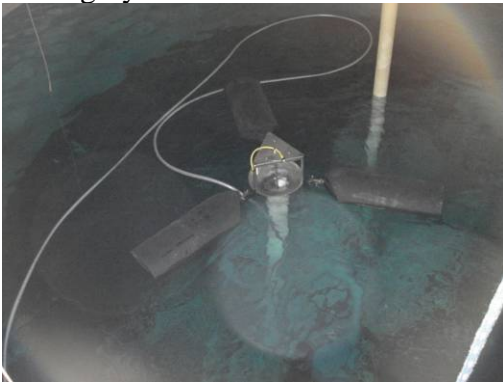
Mixing System- Duckbill Valve
