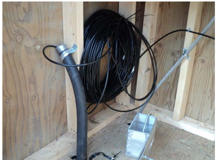
Protective conduit and connection cable for real time water quality monitoring equipment
