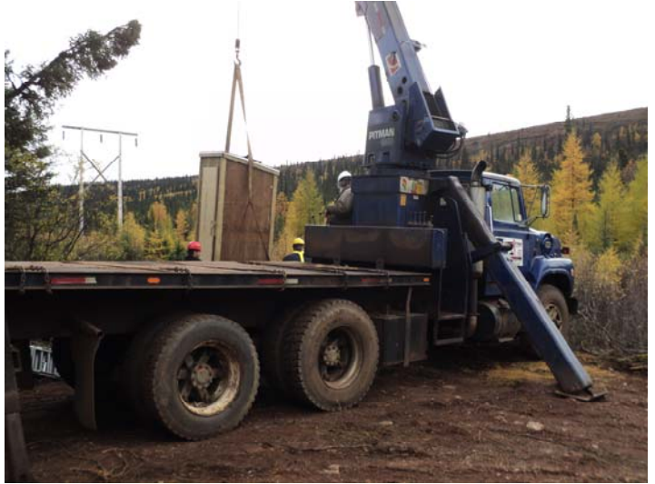
Boom truck moves station shelter into place
