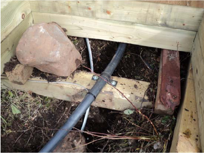
Protective conduit houses the connection cable and is securely fastened to the station shelter
