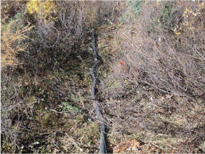
Protective conduit house the connection cable which runs from the hut to the river
