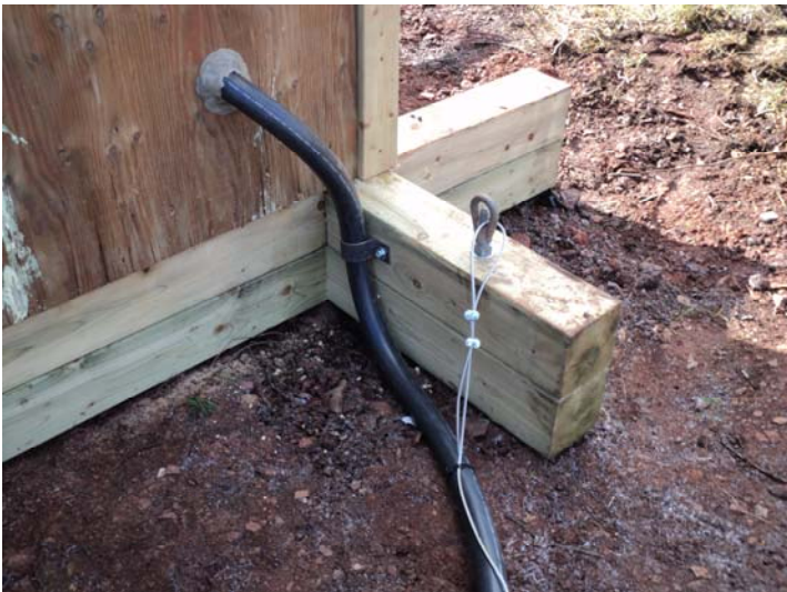
Protective conduit is securely fastened to the station
