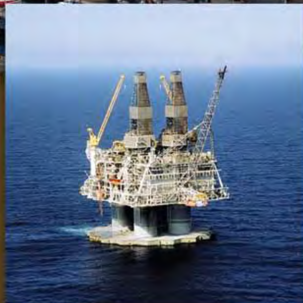
4.184 The Hibernia Platform began producing oil on November 17, 1997. It has a design capacity of 135 000 to 150 000 barrels of oil per day.
