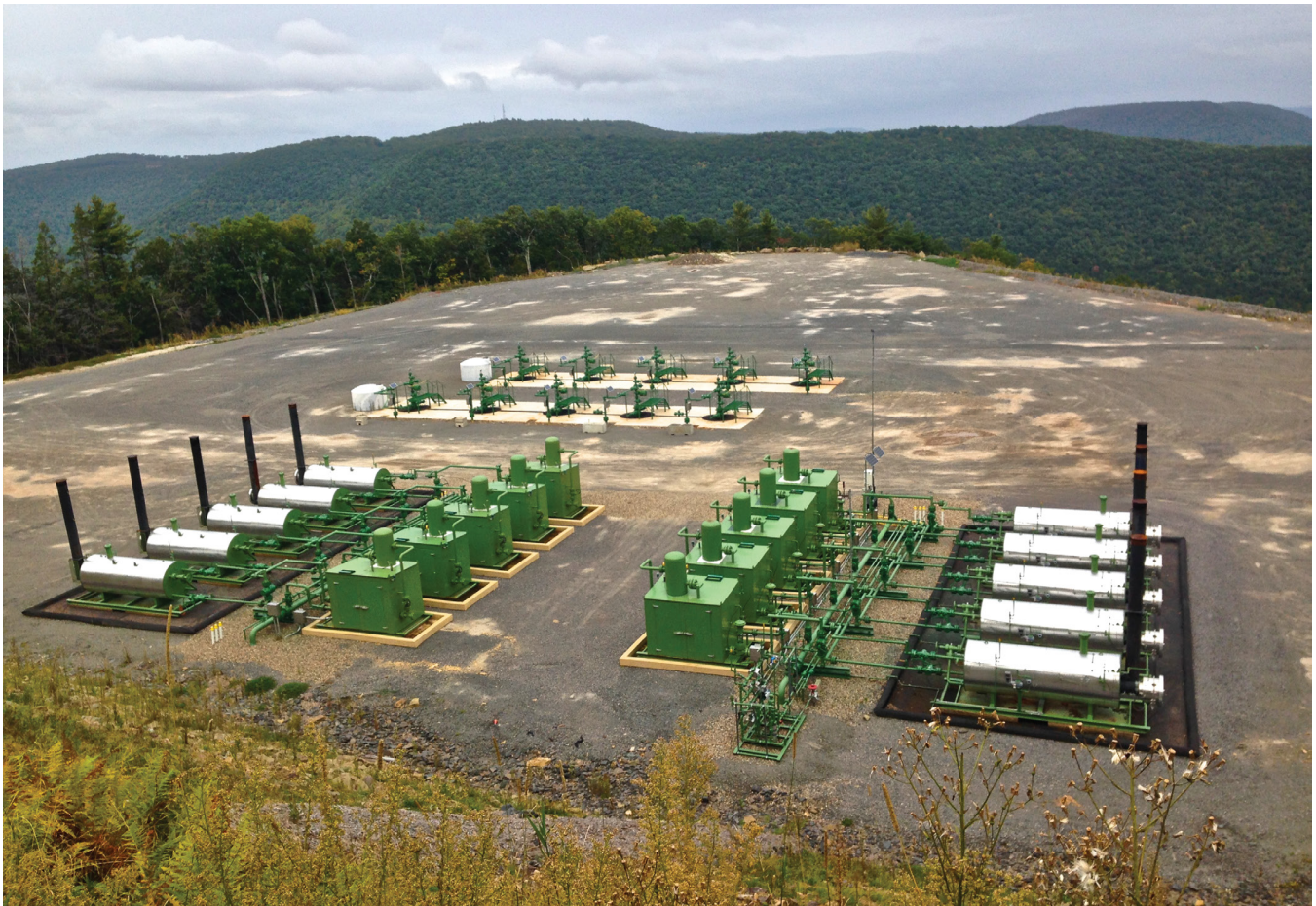
Figure 15. A producing well pad containing 10 gas wells near Williamsport, Pennsylvania.
