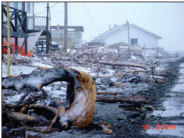
Plate 2. Storm surge caused coastal flooding, erosion and overwash on the main road in the Beaches, White Bay.
