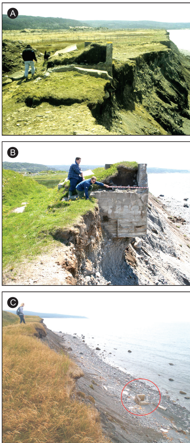
Plate 6. Cliff erosion at Point Verde. A) Cliff line in 1995. B) Cliff line in 2005. C) Cliff line in 2012. The concrete structure associated with the lighthouse shown in the 1995 and 2005 photos has now fallen to the base of the cliff.
