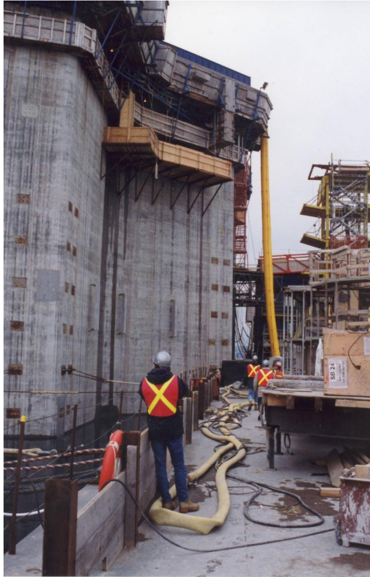
Figure 7 - Profile View of the Hibernia GBS Ice-wall Construction
