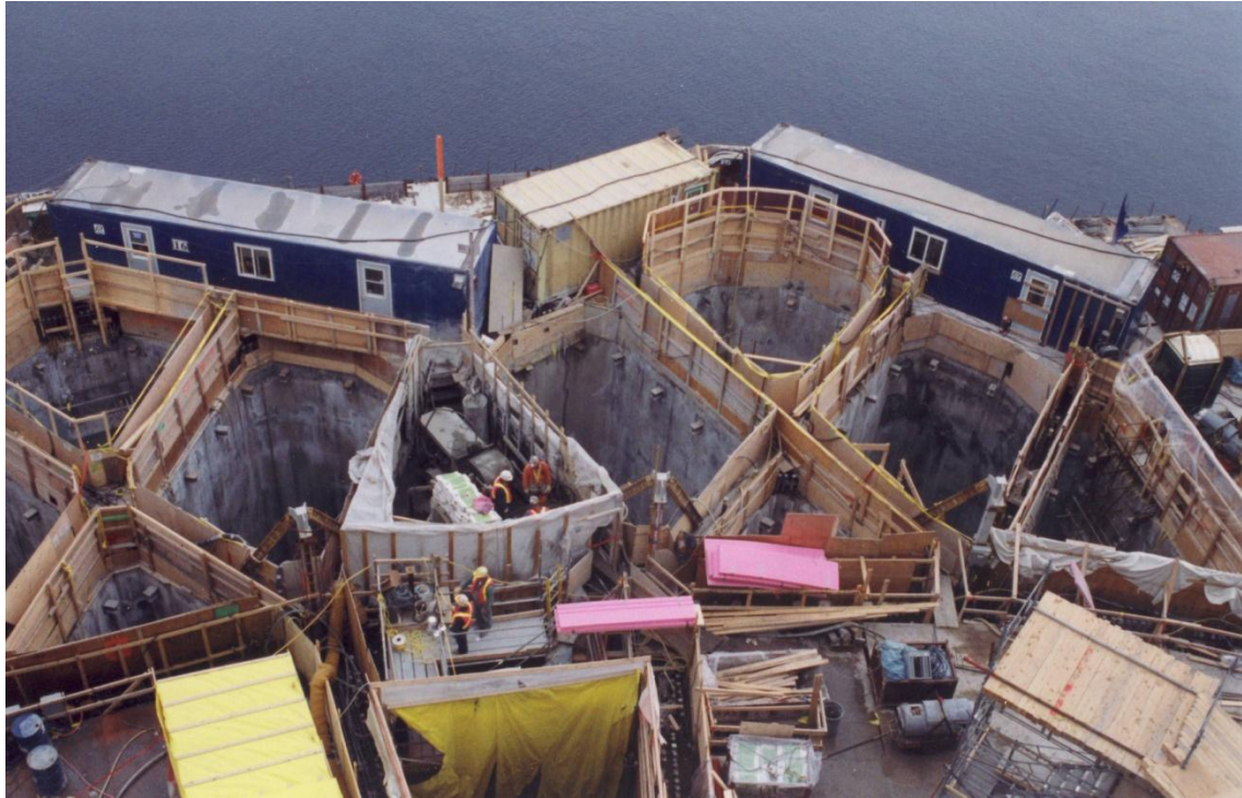
Figure 6 - Plan View of the Hibernia GBS Ice-wall Construction
