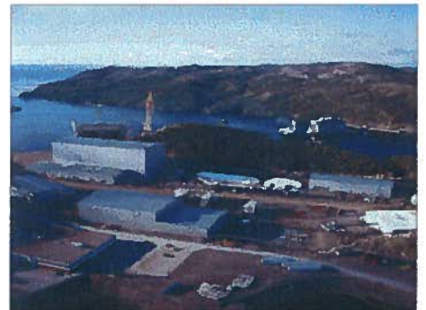
Topsides Fabrication and Assembly Area
