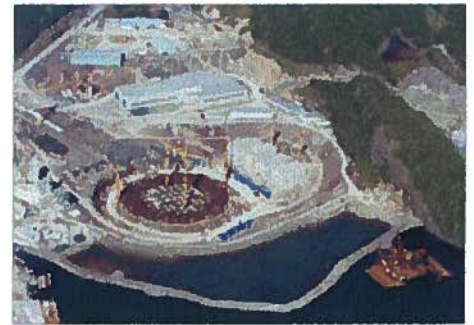
Drydock Construction and Fabrication Site
