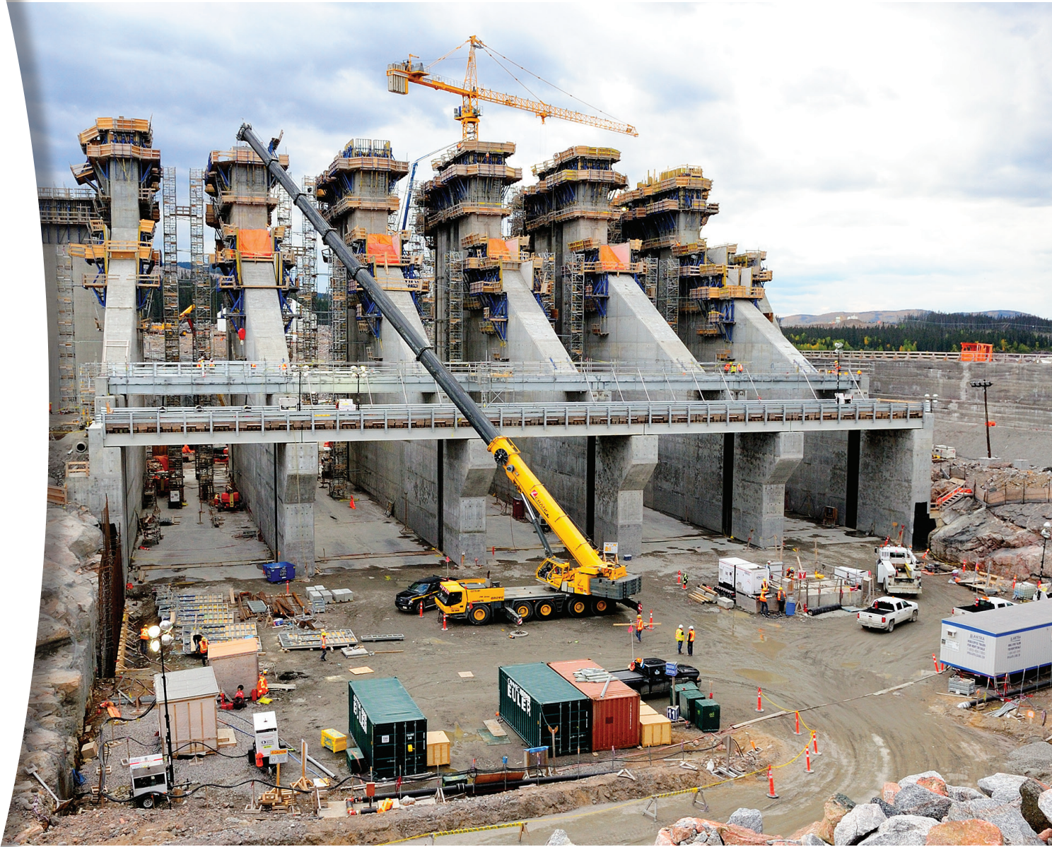
Spillway construction at Muskrat Falls. Courtesy: Nalcor Energy.
