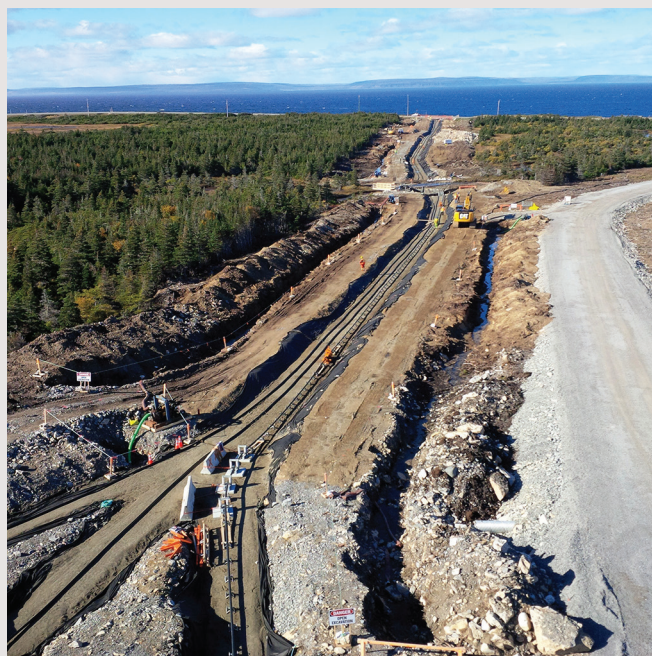
Land Cable Trench, Shoal Cove. Courtesy: Nalcor Energy.
