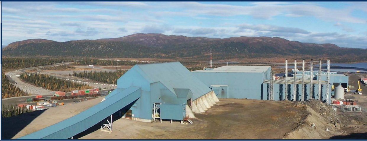
Voisey's Bay Concentrator Complex
