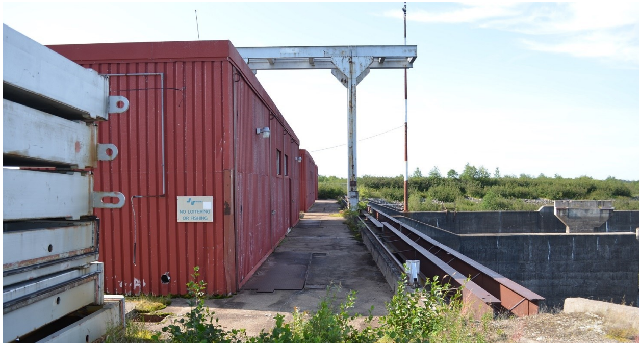
Figure 6: Twin Falls upper control room looking south. Control room buildings on the left. On the right, removed bridge support beams that prevent the intake gates from being raised. The remains of the concrete base on the bridge are on the far right (photo by the author)
