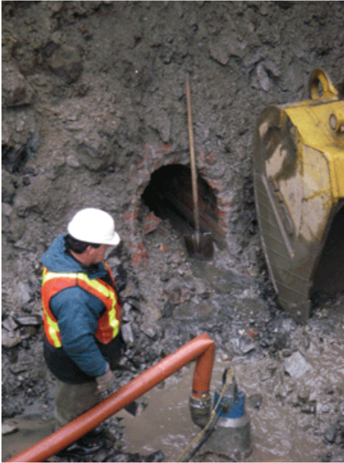
Figure 10: Ovoid brick sewer, 16 May (Penney & Cuff)
